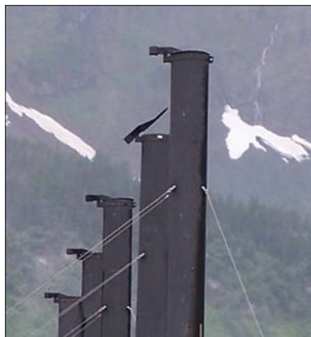
Figure 9. Example of Open and Closed Flapper Rain Caps
