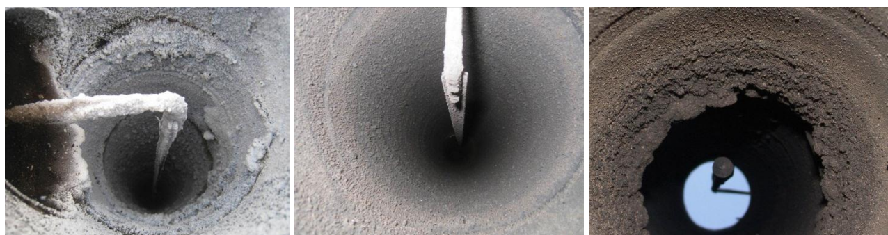
Figure 3 View to the different chimneys. From left to right: log boiler, log fire and pellet stove.
