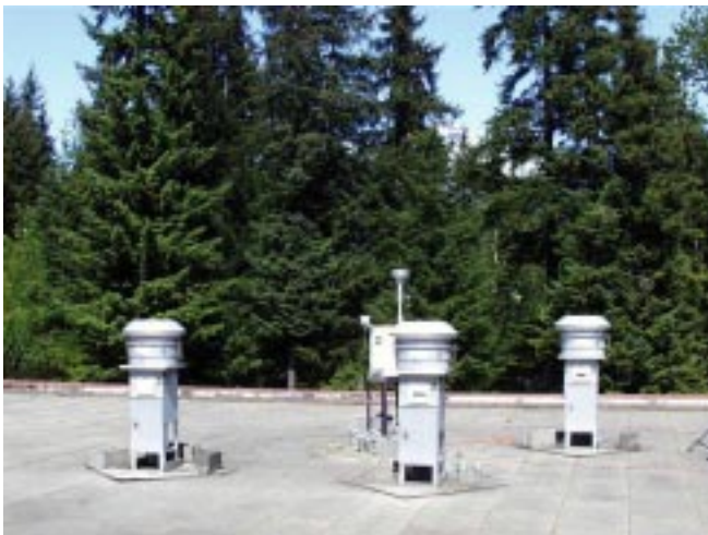
Photograph F2 - Facing north from the roof of Floyd Dryden.
