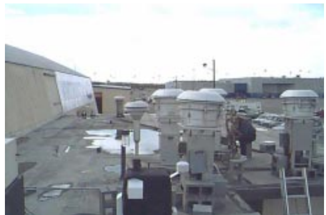
Photograph C7 - facing west from the roof of 1820 Gambell St.
