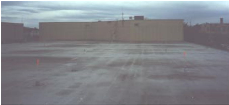
Photograph E2 - facing east from the monitoring site.
