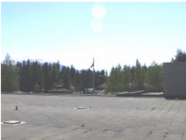
Photograph F4 - Facing south.
