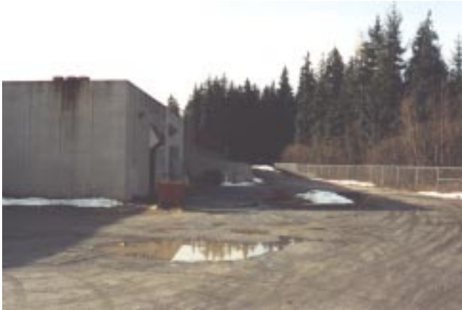
Photograph F6 - The rear of Floyd Dryden facing north-west.
