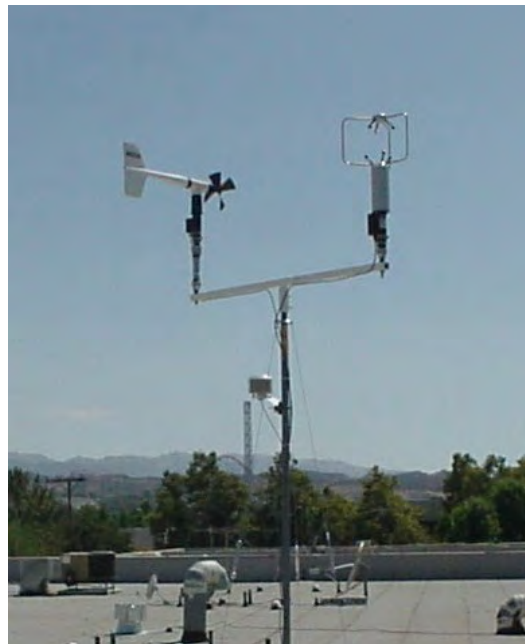
Figure 2.18 Sensor Mounting for the Testing and Evaluation of the Audit Wind Sensor Against a Sonic Anemometer
