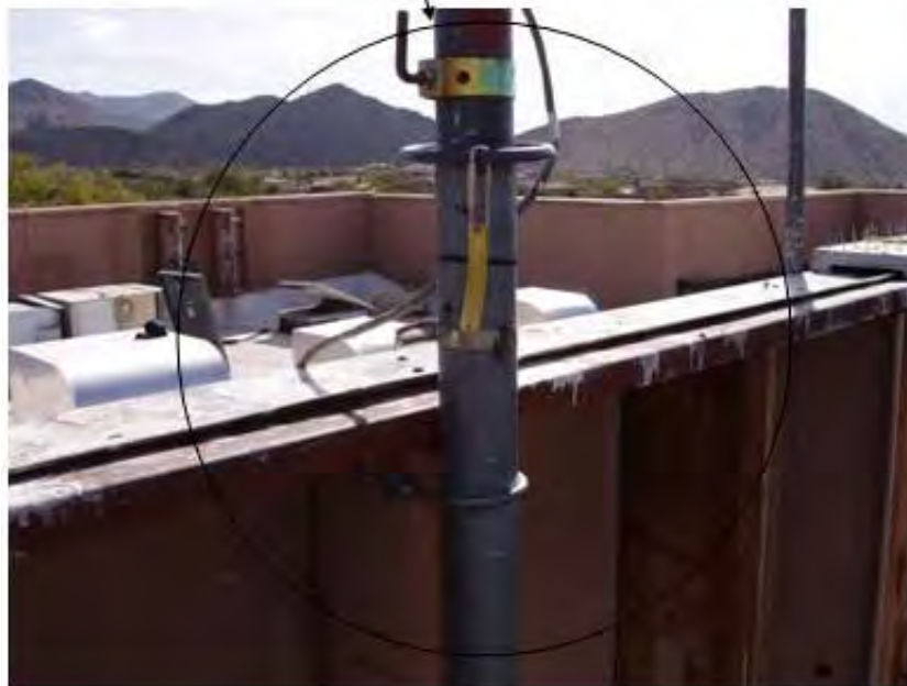
Figure 1.10 (a) Metal Wall Support—Telescopic Tower (Expanded View); (b) Metal Wall Support—Telescopic Tower (Close-Up View)
