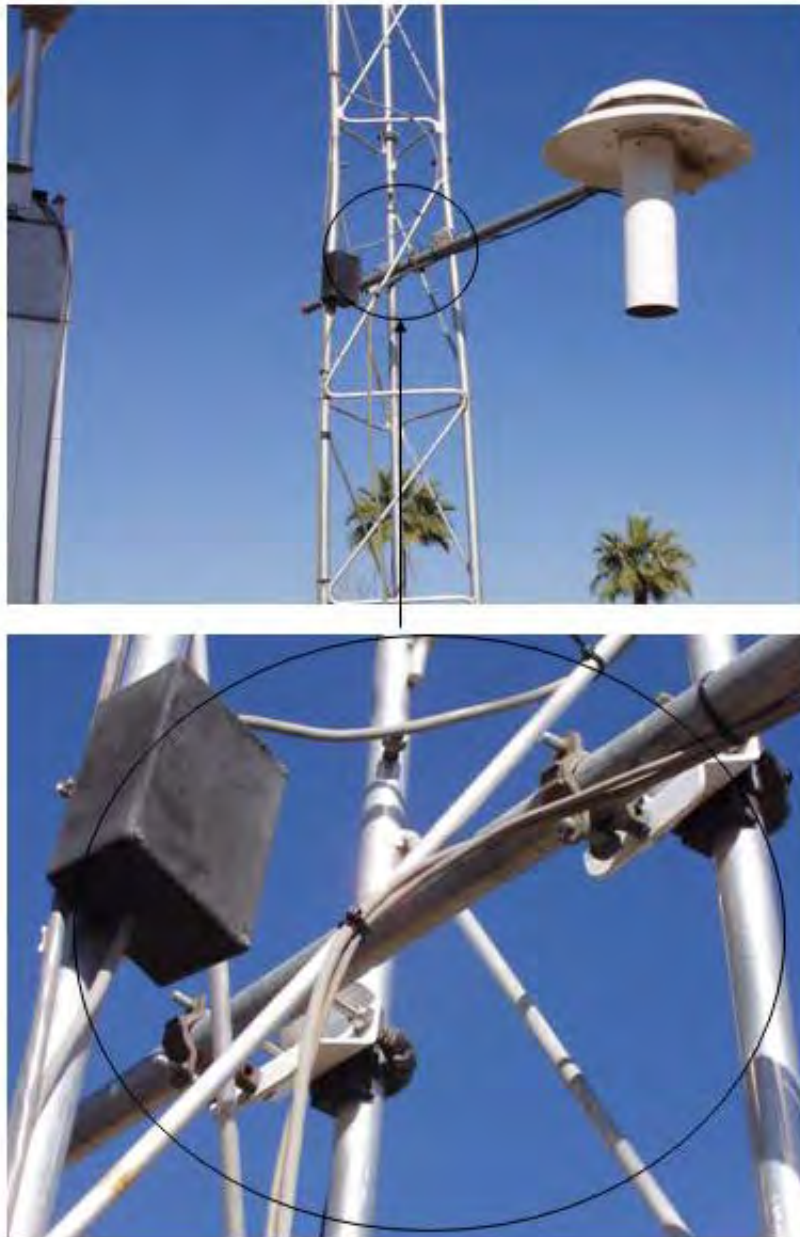
Figure 1.14 Temperature Cable Installation and Expanded/Close-Up Views
