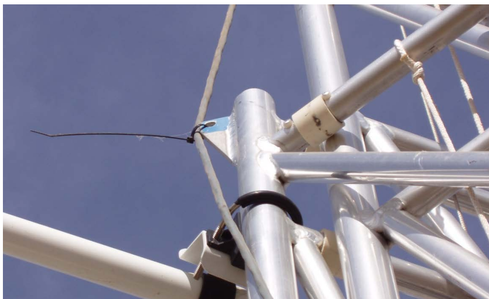
Figure 1.15 Wiring on a Crank-Down Tower
