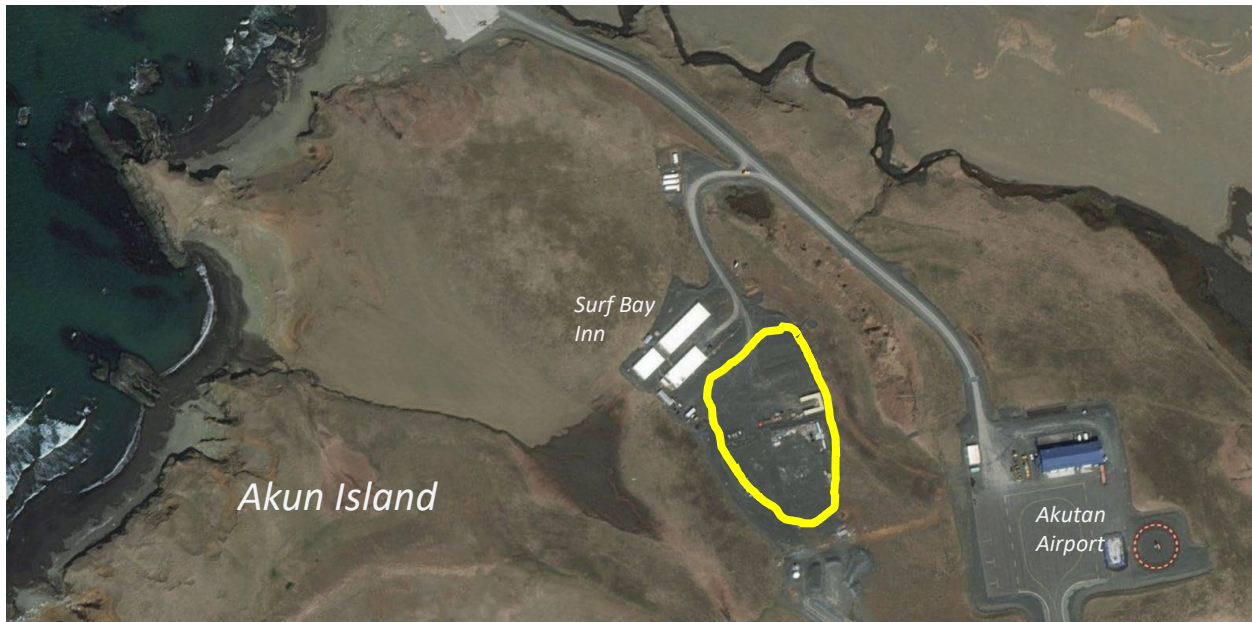
Figure 45. Potential Dredge Material Storage Site
