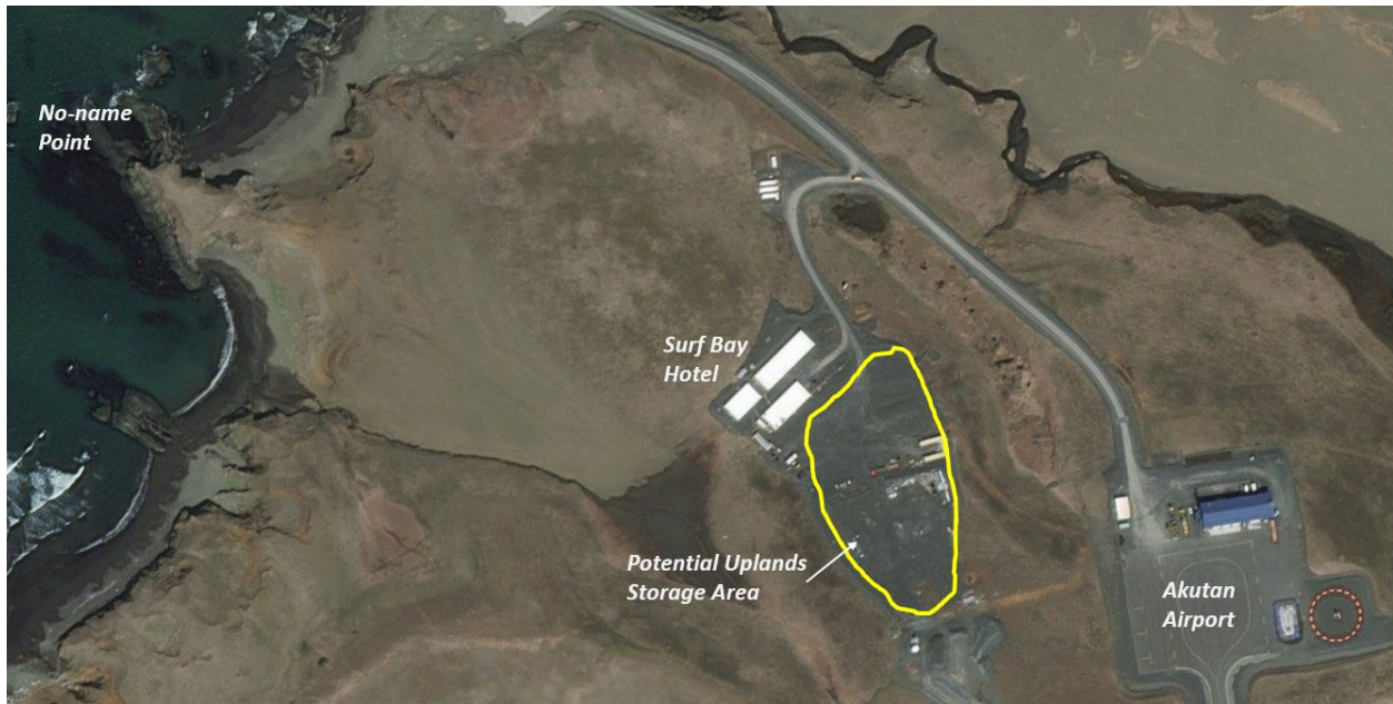
Figure 44. Potential Upland Storage Location.
