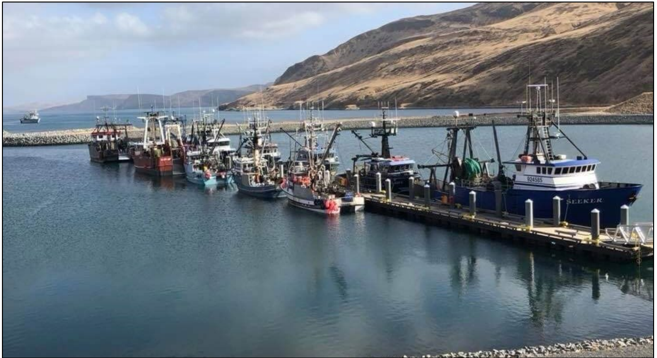
Figure 23. Akutan Harbor (small boat harbor)
