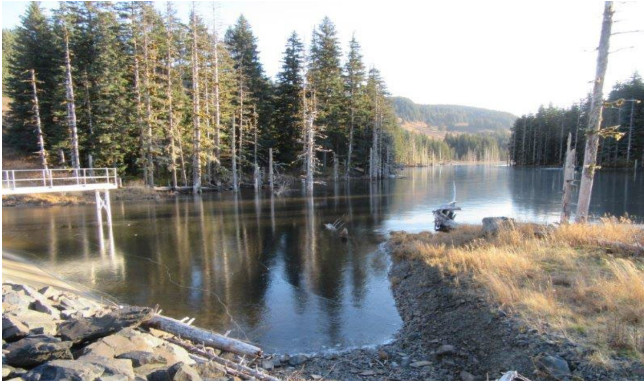
Reservoir in Ouzinkie, Alaska
