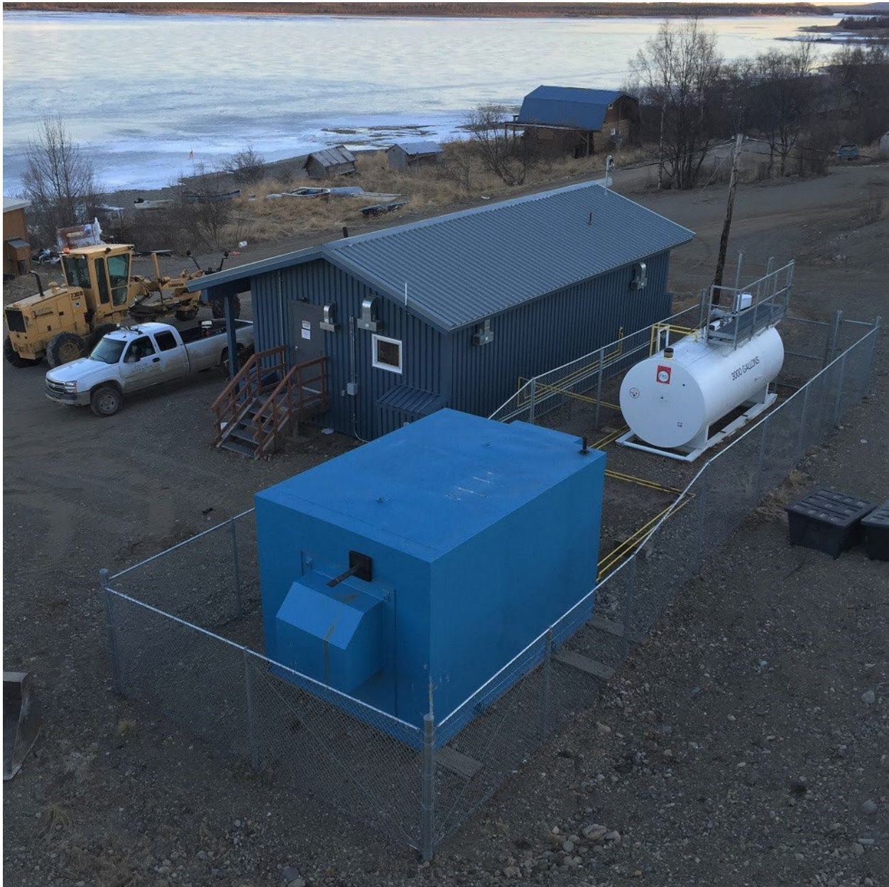
Water Plant in Nondalton, Alaska
