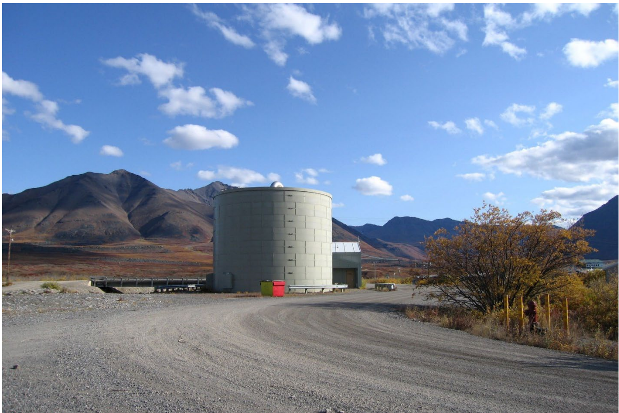
Water Plant in Anaktuvuk, Alaska
