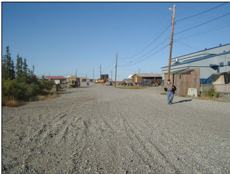
Figure 3 Unpaved Street in Noatak
