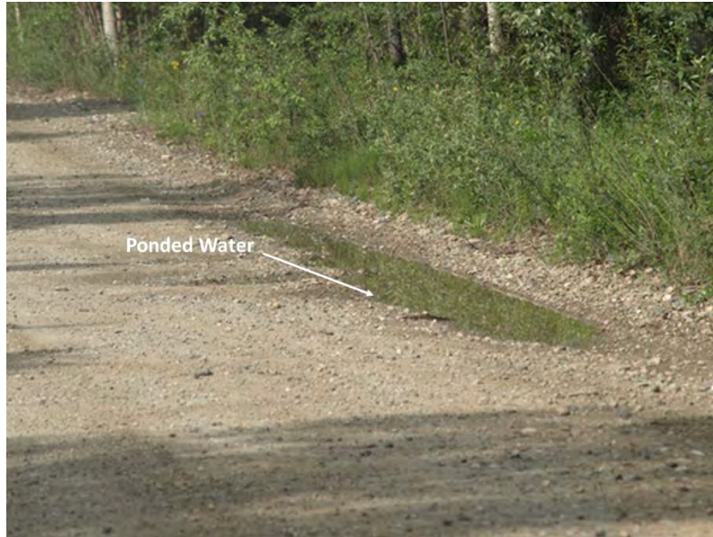
Figure 4.8 Ponded water due to improper ditching
