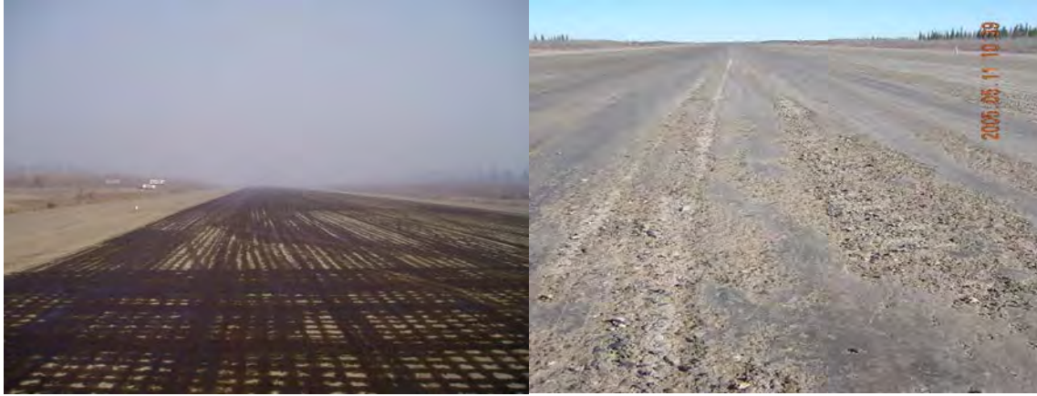
Figure 5.8 improper application (left) and performance (right)
