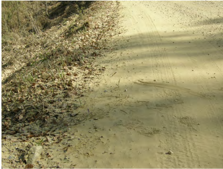
Figure 2.6. Relatively large dust particles that have settled out at the edge of a gravel road
