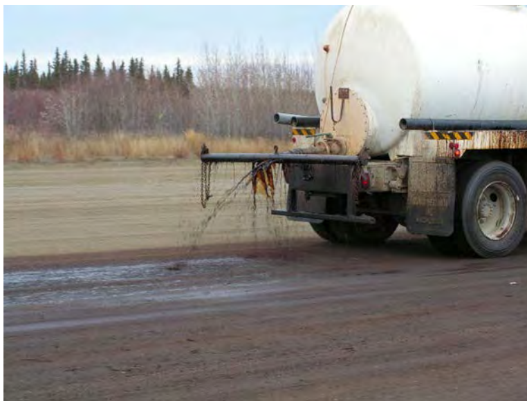
Figure 5.9 Uneven application with a water truck
