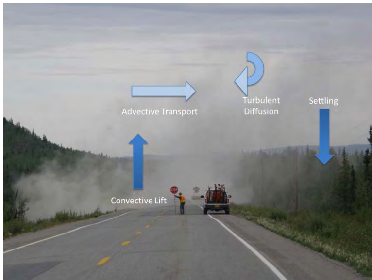
Figure 2.4. Process involved in particle movement and settling
