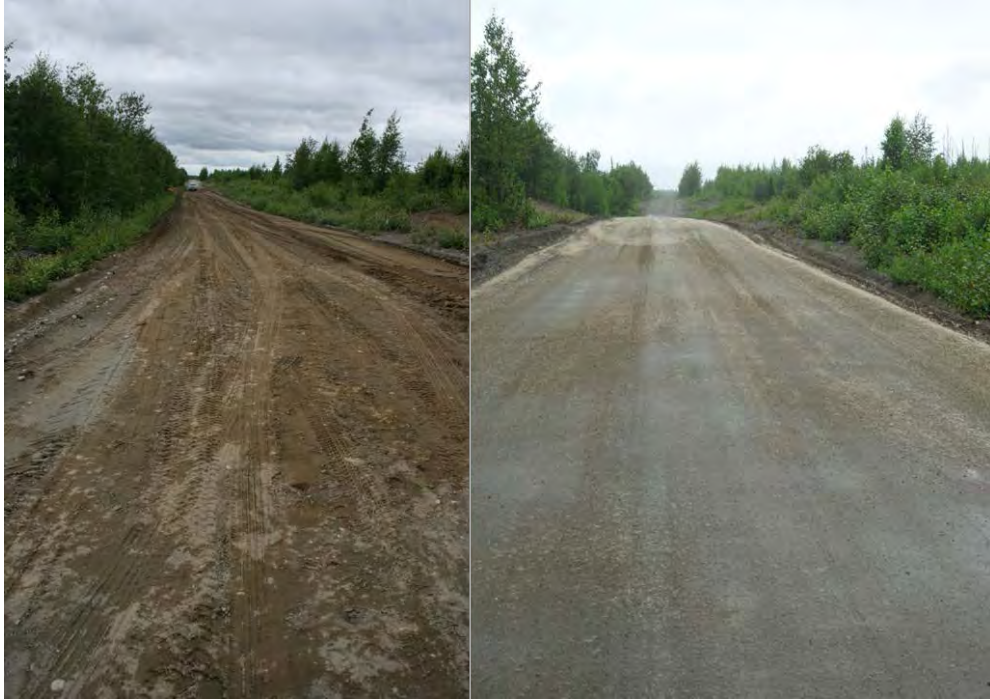
Figure 5.12 Horseshoe Lake Road before and after three years of applying polymer
