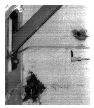
preventive measures include repairing cracks and holes and sealing the wall with concrete sealant paint.
