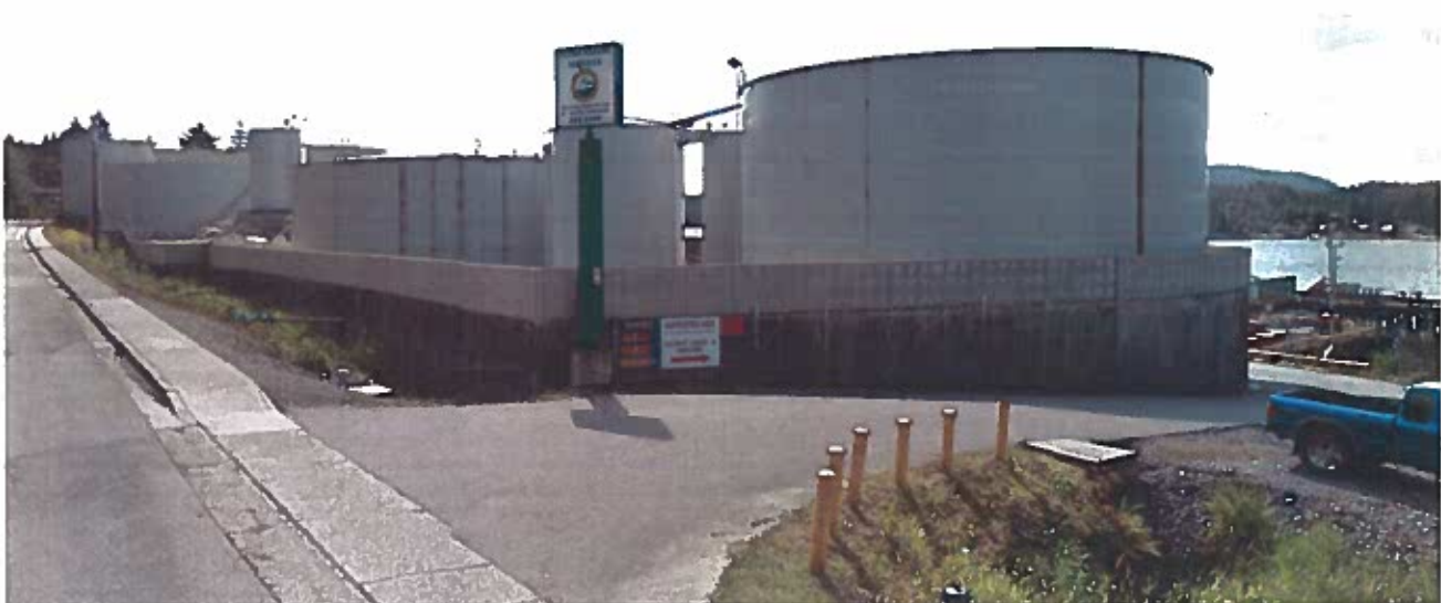
Figure 1. Entrance to the Petro Marine Facility from Stedman Street, northwest corner of the property
