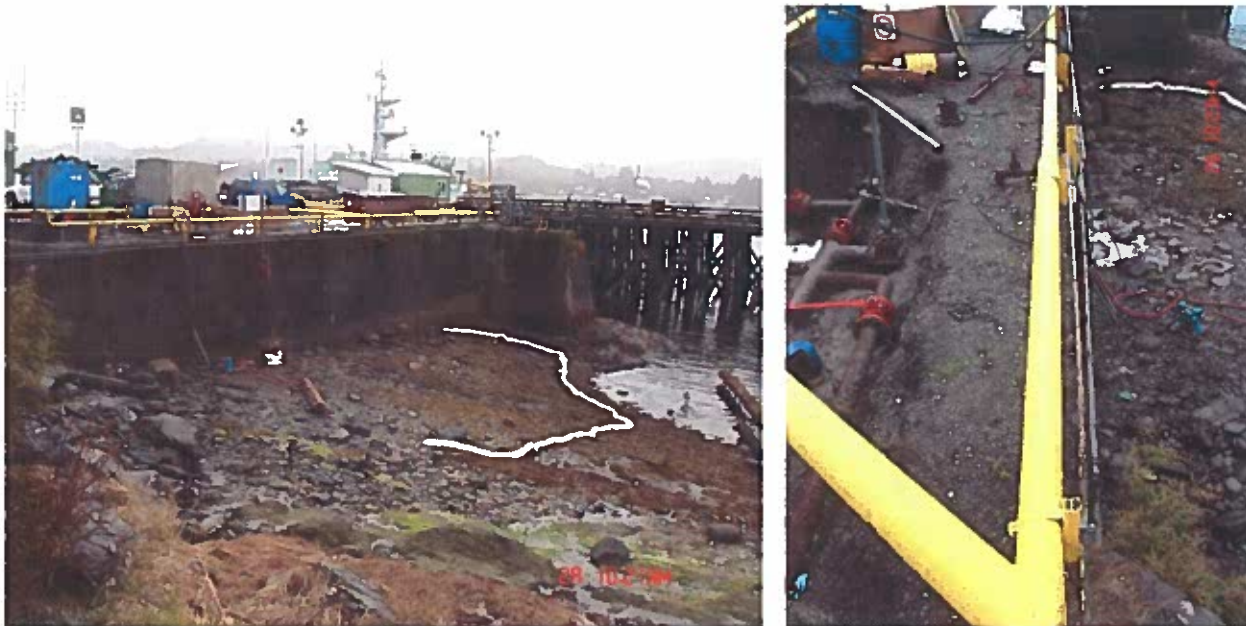
Figure 3. West facing seawall and sorbent boom
