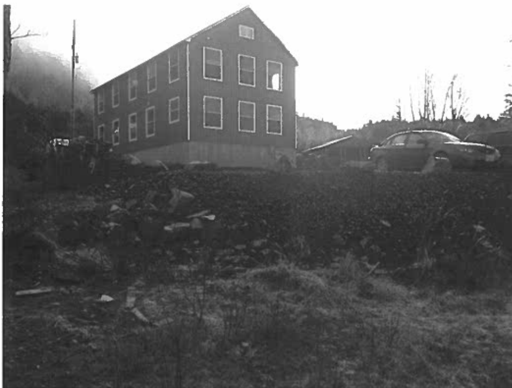
Figure 2: Former Kavalco bunkhouse, Kasaan, AK.
