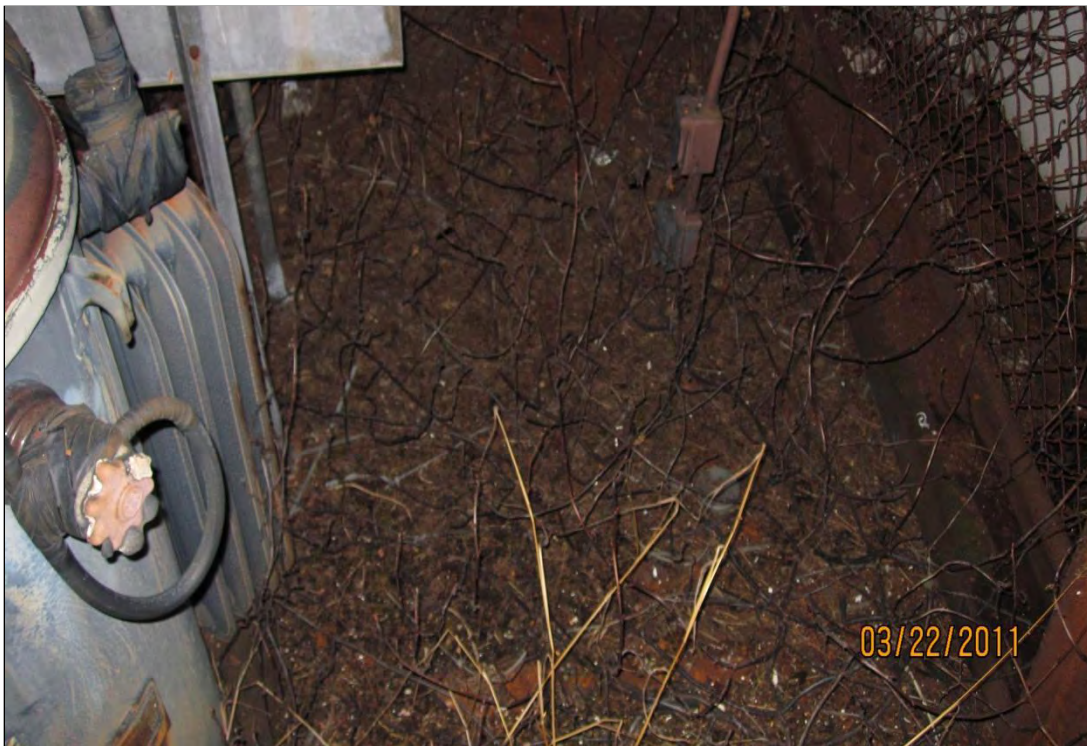
Photo 24. Discolored (stained) dirt over concrete foundation adjacent to PCB bearing transformers located on the exterior of the engine room building.
