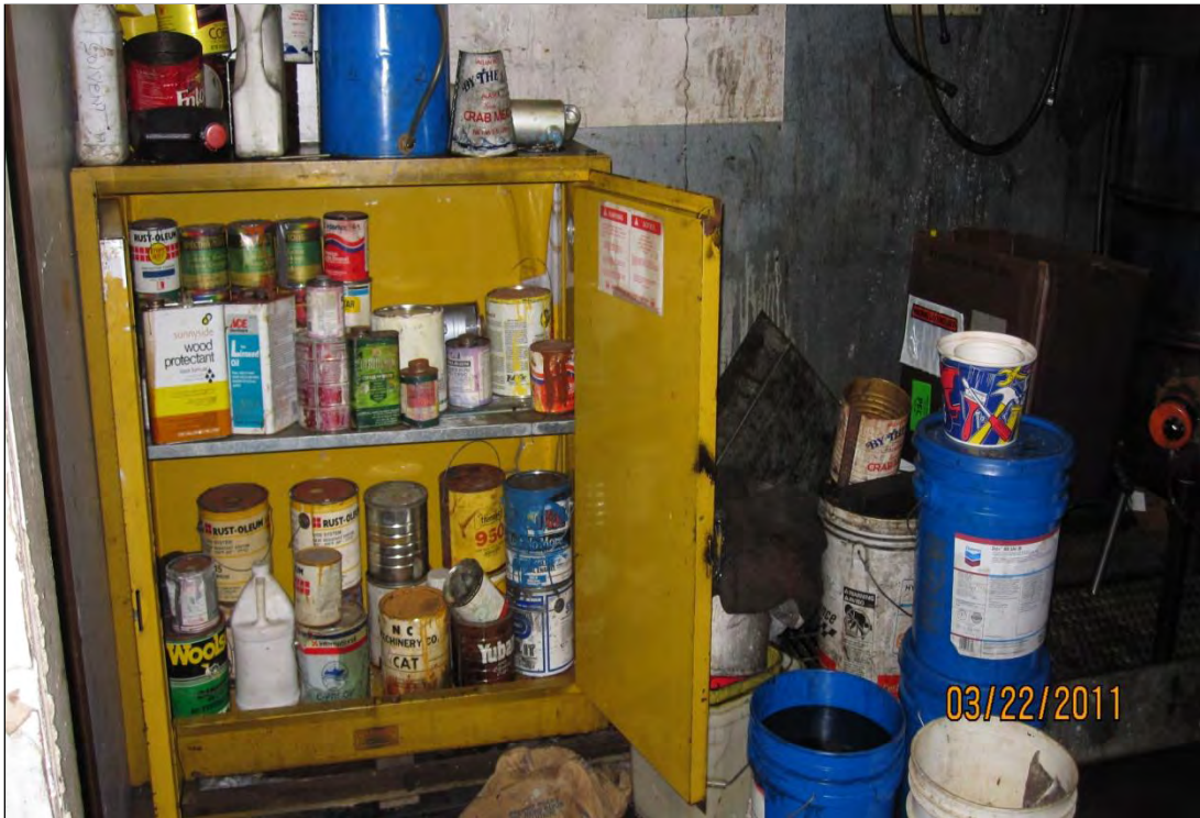
Photo 2. Flammable materials cabinet located on northeast side of engine room building.
