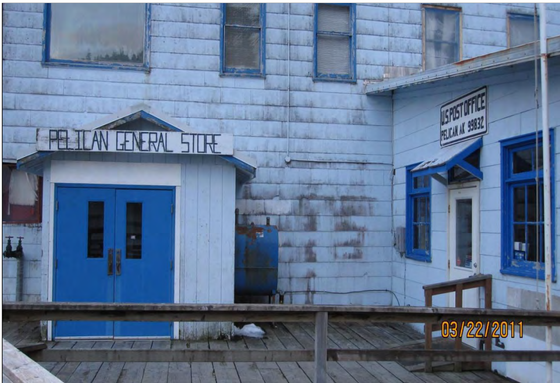
Photo 16. Heating oil AST located between the U.S. Post Office and the store.
