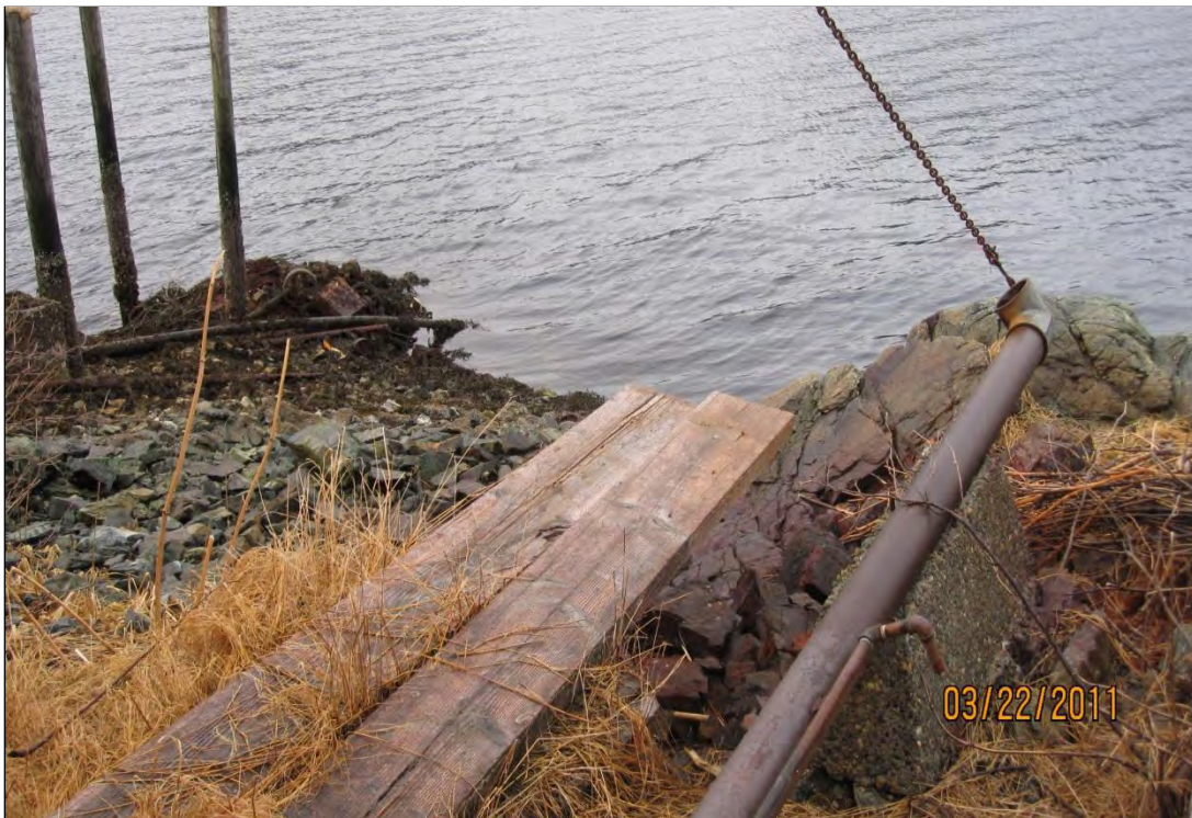
Photo 26. Discharge pipe protruding westward from engine room building. Smaller diameter pipe was reportedly used to drain oil from the ammonia compressors.
