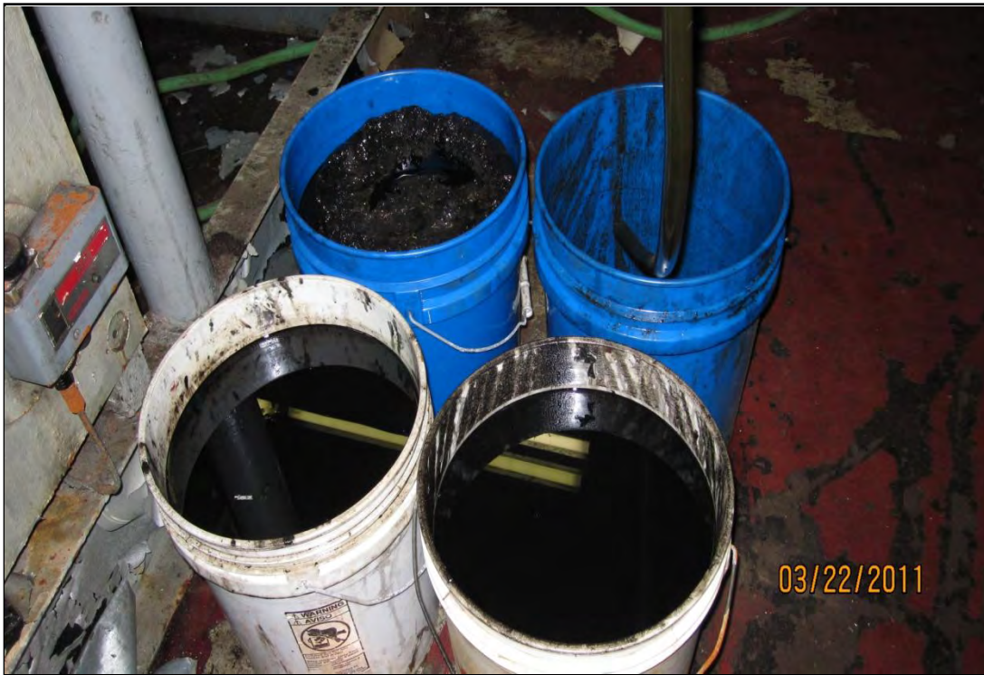
Photo 11. Open containers of used ammonia compressor oils inside engine room building.
