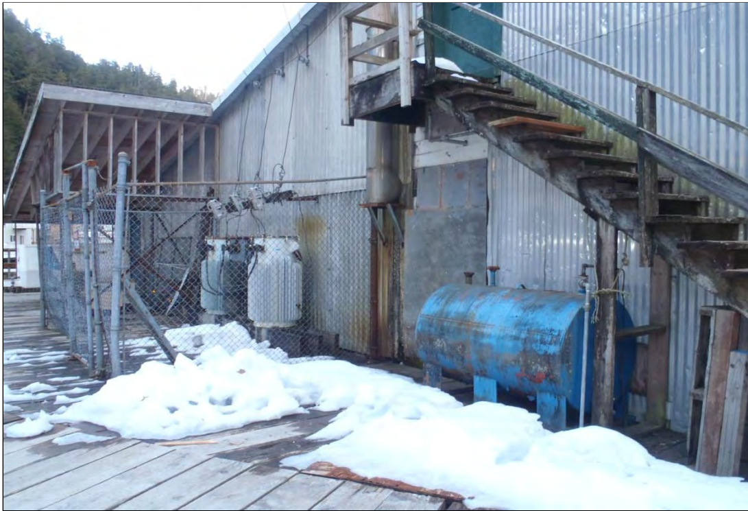
Photo 15. Heating oil AST located on the north side of the crab plant building.
