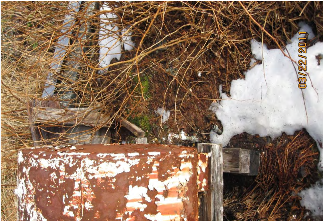
Photo 20. Easternmost company house (condemned) AST with missing pipe segment, stain, and stressed vegetation.
