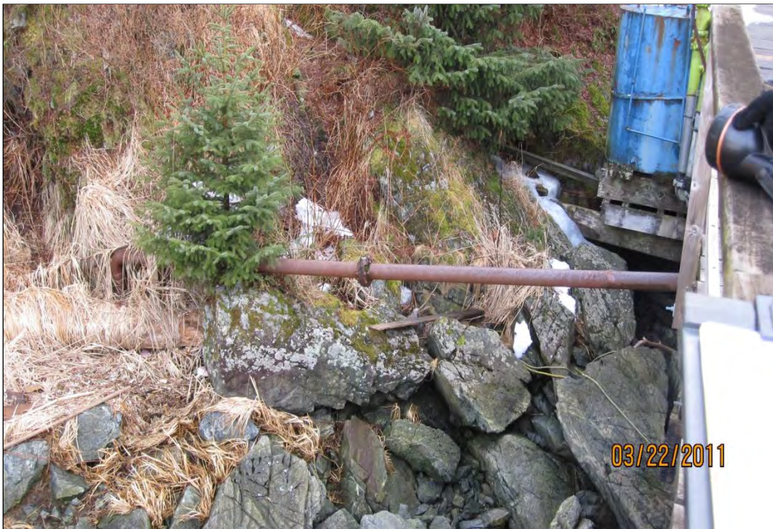
Photo 27. Unknown pipe (reportedly capped) located on the north side of boardwalk on the north side of the crab plant building.
