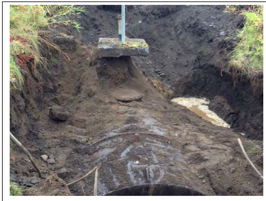
Photo 2: Water encountered during UST excavation; looking east. (September 16, 2014)
