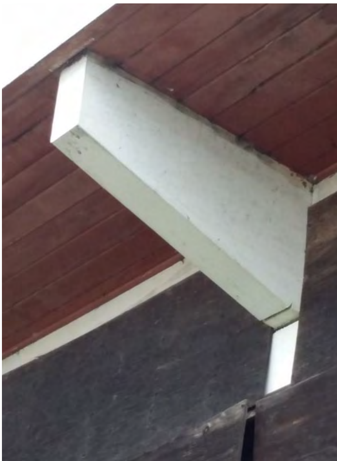
Figure 10. Detail of the trapezoidal wooden brackets (©TNSDS 2014).
