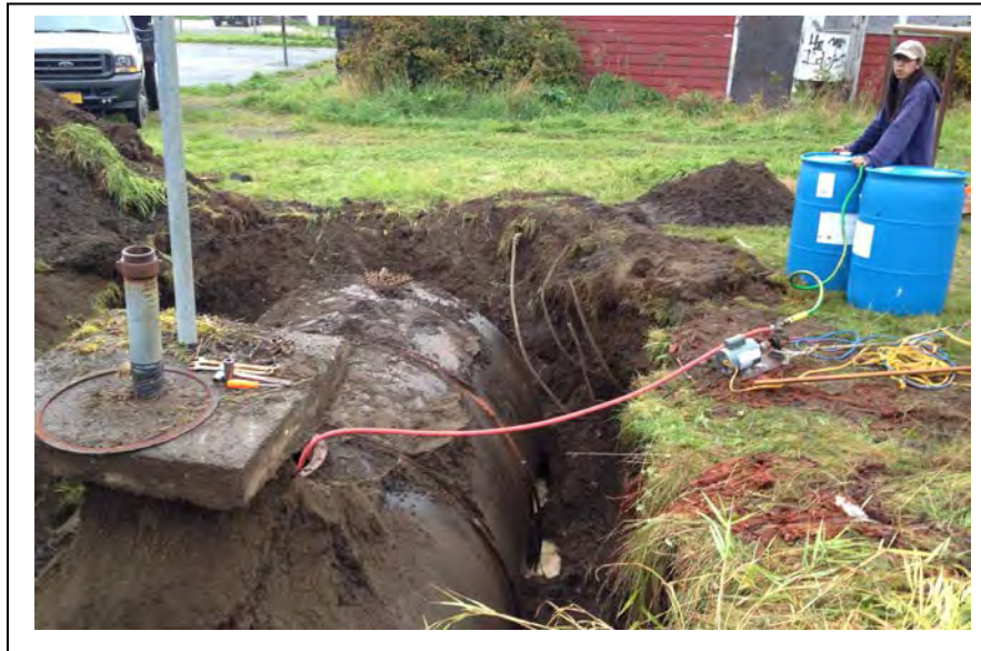
Photo 1: Removing the residual heating oil from the UST; looking west. (September 16, 2014)
