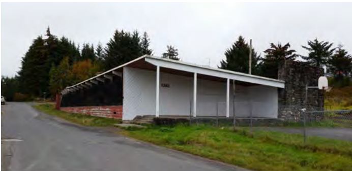
Figure 7. The Old Kake Elementary School, south and west facades (©TNSDS 2014).
