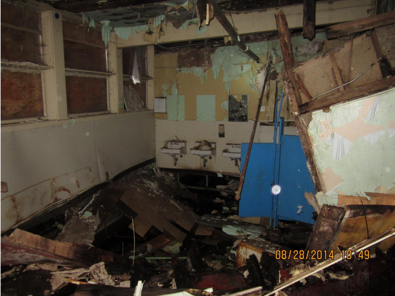
Figure 4: The interior of the School.
