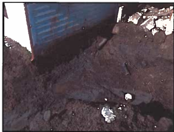
Excavation area on east side of building.
