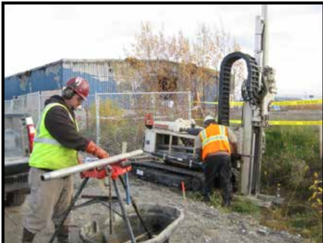
Photo 35: 9/28/2011 – Typical perimeter ditch soil-boring efforts.
