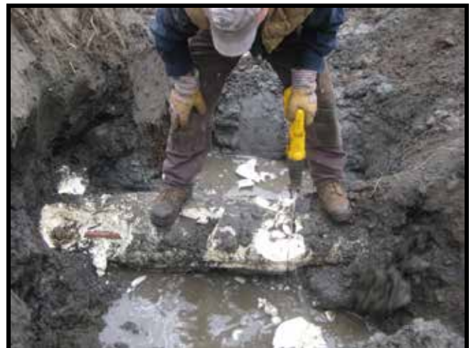
Photo 48: 10/11/2011 – Disconnecting water line near the main for winterization efforts.
