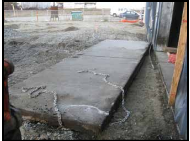
Photo 38: 10/12/2011 – Removal of southern apron for corrective action and characterization.
