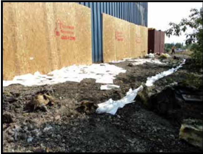
Photo 13: 5/29/2011 – West building perimeter sludge and surface migration control.
