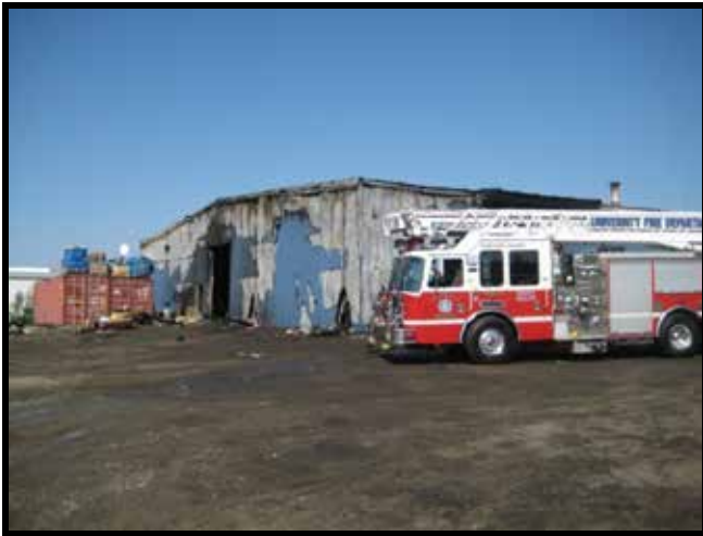
Photo 1: 5/27/2011 - South side of NAPA facility during initial visit.
