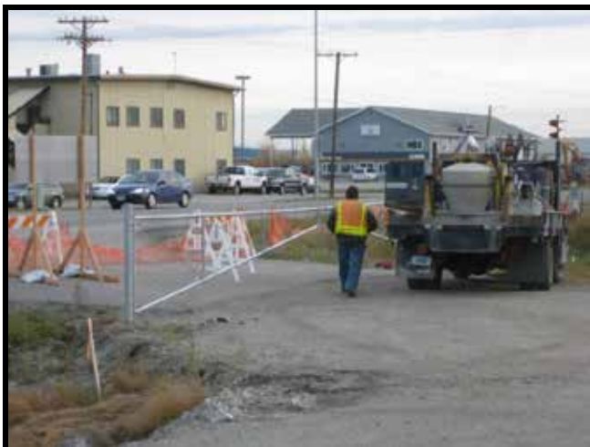
Photo 47: 10/3/2011 North Driveway gate installation.
