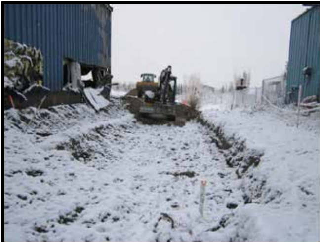
Photo 53: 10/17/2011 - Looking south along the West Ditch with MW1 in foreground
