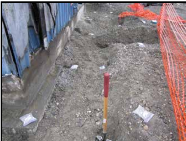
Photo 41: 10/16/2011 – Typical building perimeter field screening.
