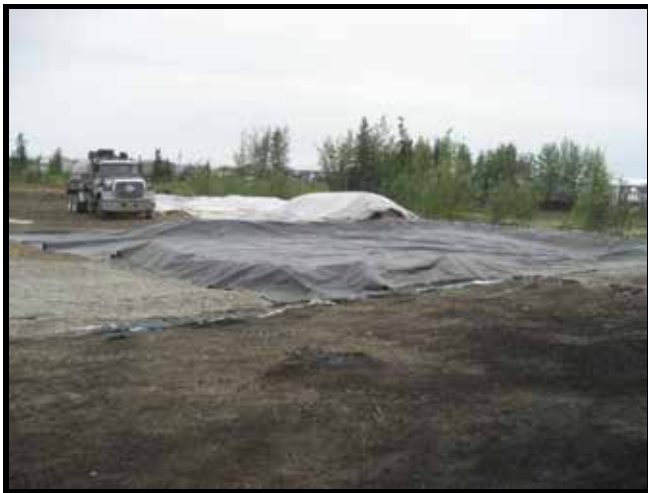
Photo 15: 6/2/2011 – Southern soil stockpile construction.
