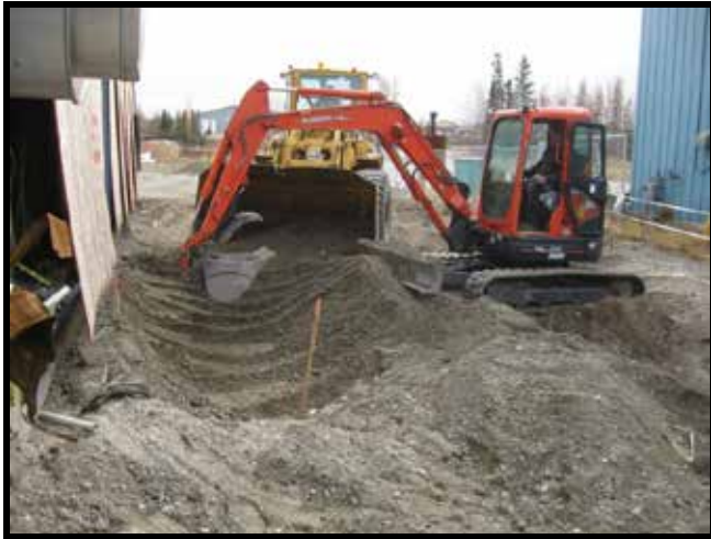
Photo 49: 10/11/2011 – Corrective action at 1:1 slope toward the West Ditch.
