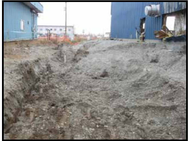
Photo 50: 10/13/2011 - Western and bottom limits of West Ditch excavation (MW2 in center).
