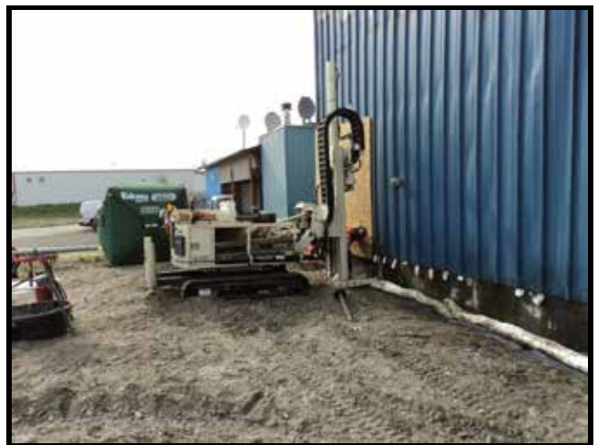
Photo 22: 6/9/2011 – Initial building perimeter soil boring.
