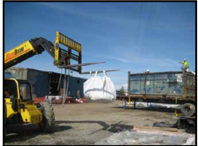
Photo 44: 8/26/2011 – Loading interior building waste for transport.
