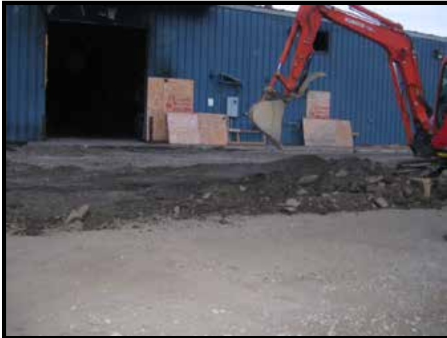
Photo 43: 10/4/2011 – Removal of East Driveway RAP.
