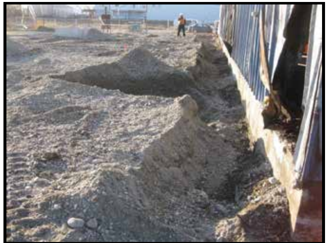
Photo 40: 10/12/2011 - Build perimeter corrective action on south side of building.
