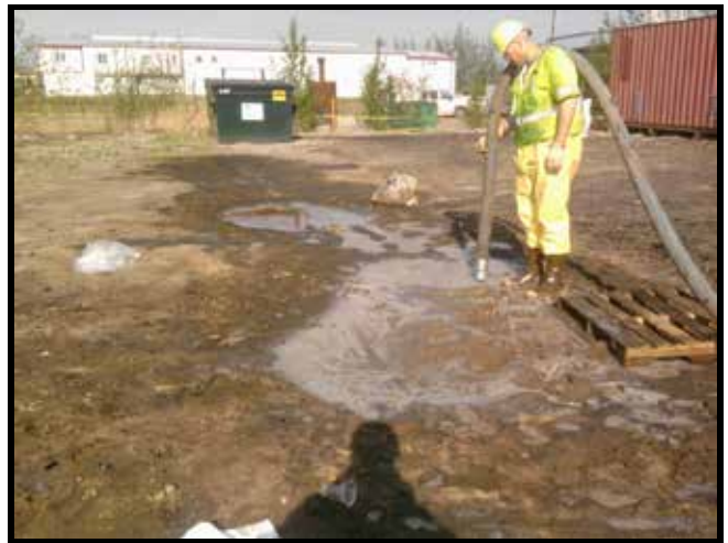
Photo 10: 5/28/2011 – Direct Vac-truck oil and sludge phase collection from south driveway.
