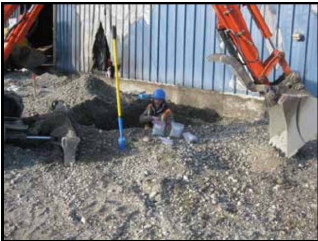
Photo 39: 10/12/2011 – Typical excavation for building perimeter profile characterization.
