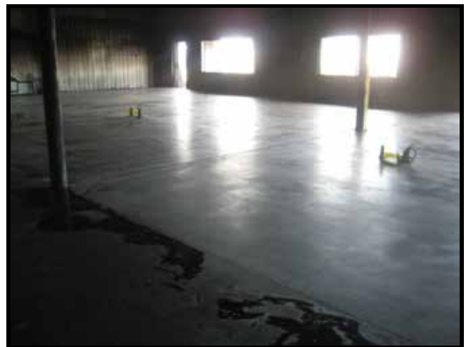
Photo 46: 9/29/2011-Typical concrete floor section after cleaning.
