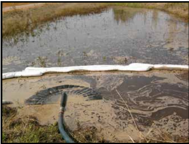
Photo 9: 5/28/2011 – “Stinger” collecting floating phase contaminants from the South Ditch.
