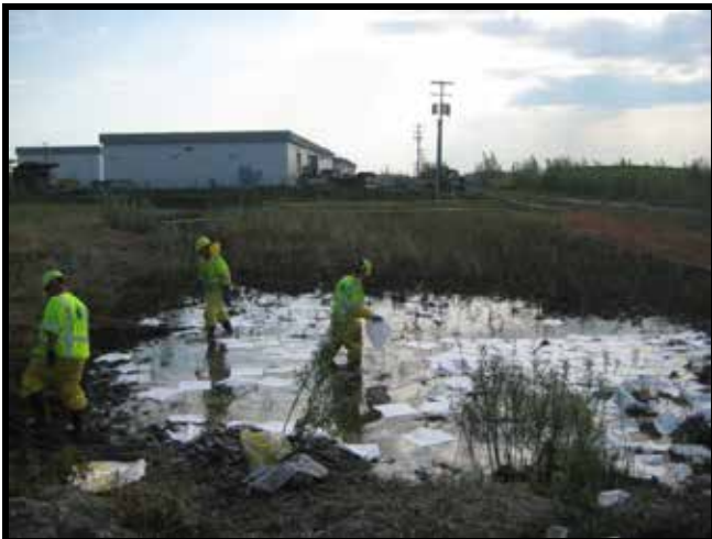
Photo 11: 5/29/2011 – Southeast perimeter Ditch surface contaminant absorption.
