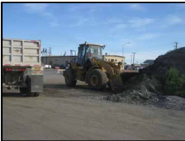
Photo 45: 9/26/2011 – Typical soil loading for thermal remediation.
