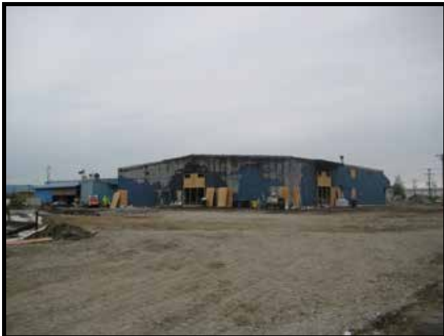
Photo 17: 6/2/2011 – South driveway and southern waste storage areas after initial surface scraping.
