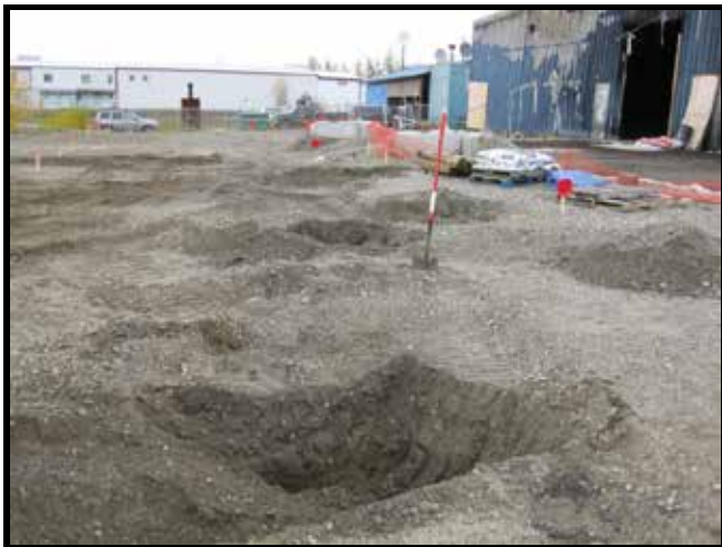
Photo 33: 9/22/2011 – Looking west across Pit 3 through Pit 6.
