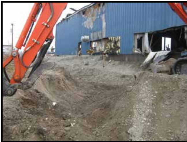
Photo 51: 10/13/2011 – Corrective action near the south end of the West Ditch.
