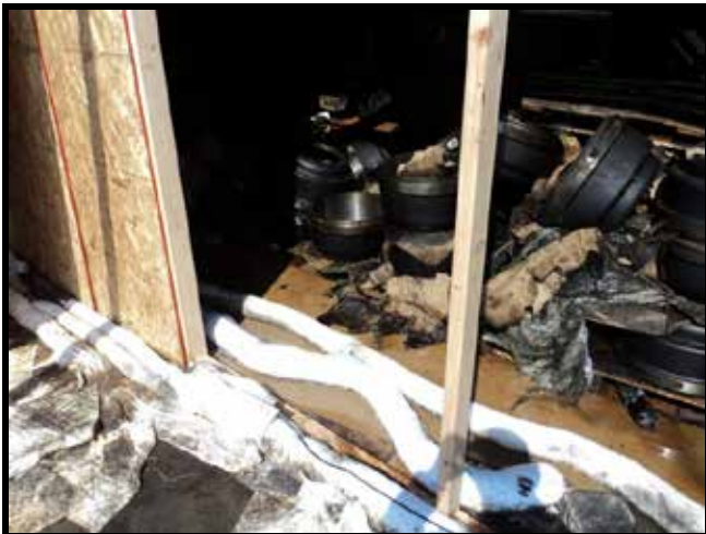
Photo 5: 5/27/2011 – South warehouse door sludge containment.
