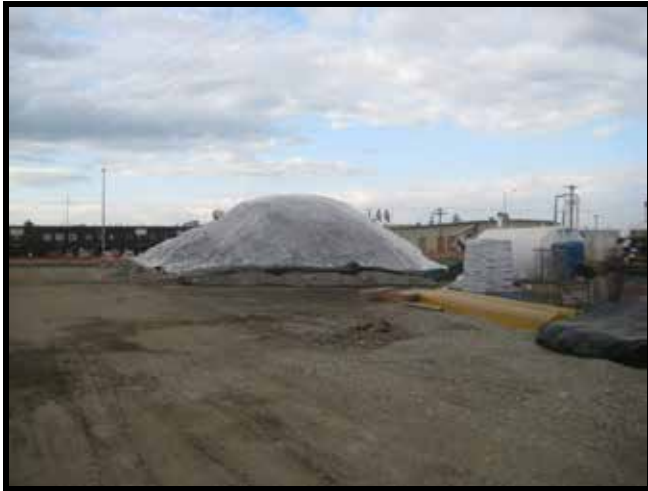
Photo 19: 6/3/2011 - Eastern stockpile excavated from perimeter ditches.
