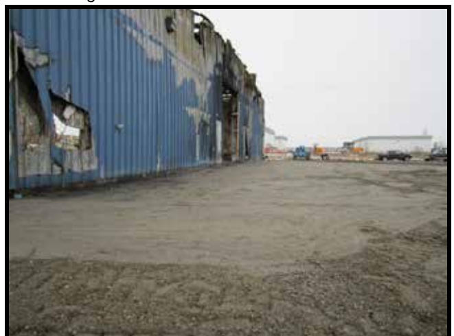
Photo 60: 10/18/2011 – Typical final grade prior to building demolition.
