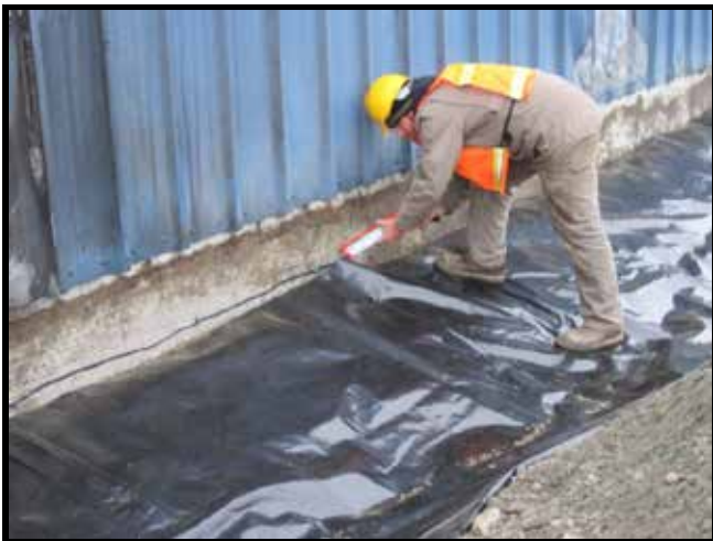
Photo 57: 10/17/2011 – Typical sealing of vapor barrier onto concrete pad.
