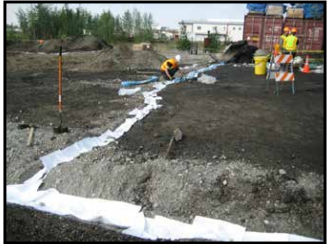
Photo 14: 5/29/2011 – Initial containment trench near the southeast corner of the building.
