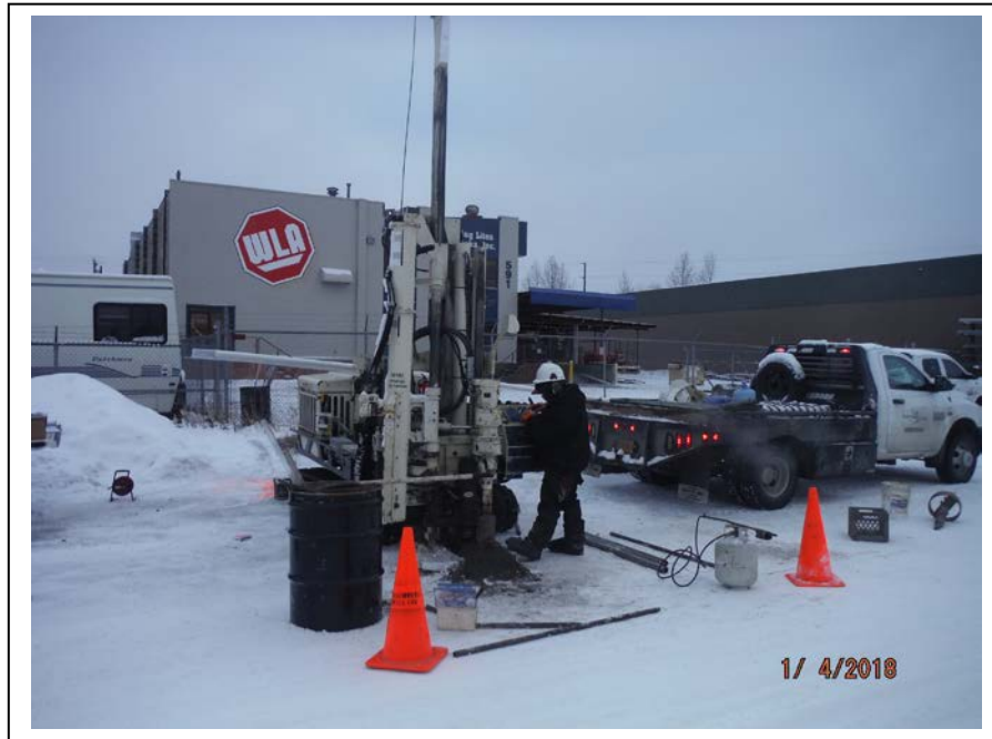
Photo 1: Looking north during the advancement of Boring B5. (January 4, 2018)
