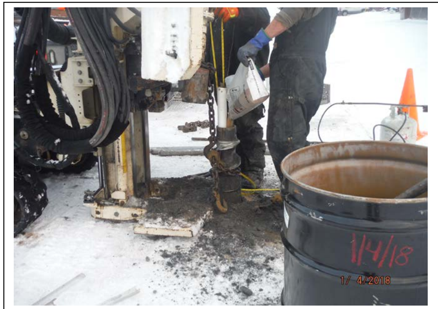
Photo 2: Looking east, Boring B5 was completed as Monitoring Well B5MW. (January 4, 2018)
