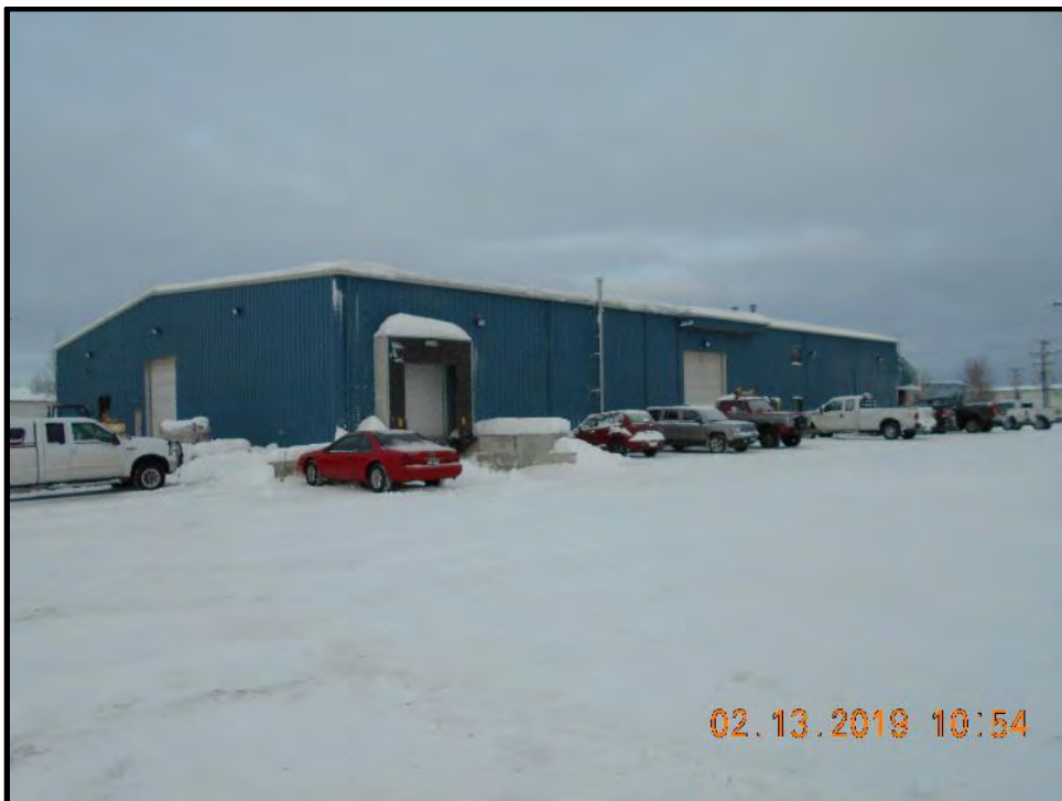
Photo 2: February 13, 2019. Looking northwest at the NAPA Auto Parts Store. MW4 is located adjacent to the east side VES housing stack shown rising to above the roof line. This well is situated at the corner of the rebuilt NAPA store before an addition was added in 2013.
