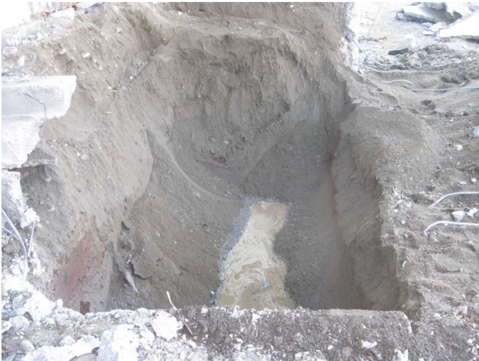
Photograph 2: Location of former UST. Groundwater at 3.5 feet below grade. View looking west.
