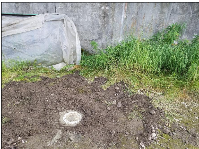
RSE-7 upgradient against Coastal Trail retaining wall.
