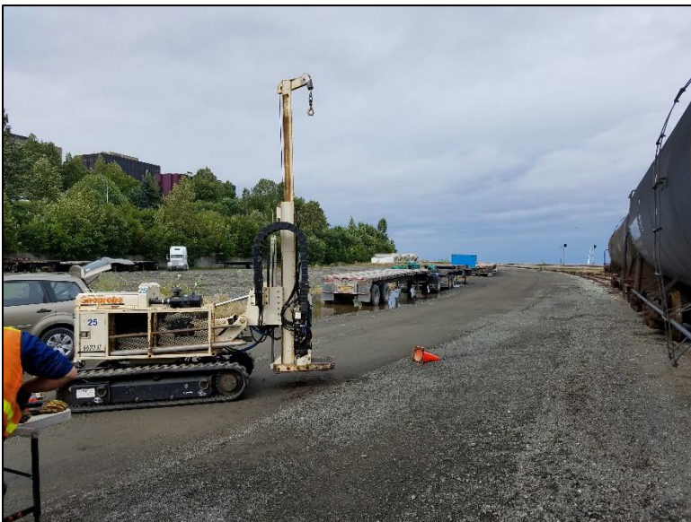
View RSE-2 facing west.
