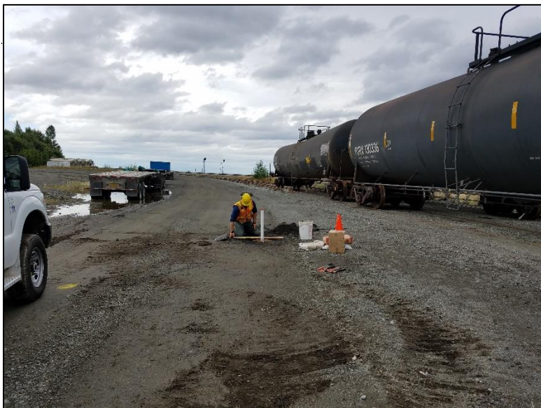
Setting the well at RSE-1. Facing west.
