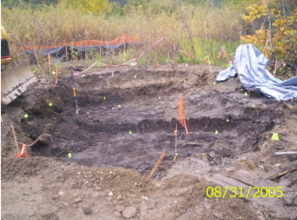
Photo 5. Inclusive contaminated area dug to 36 inches bgs.
