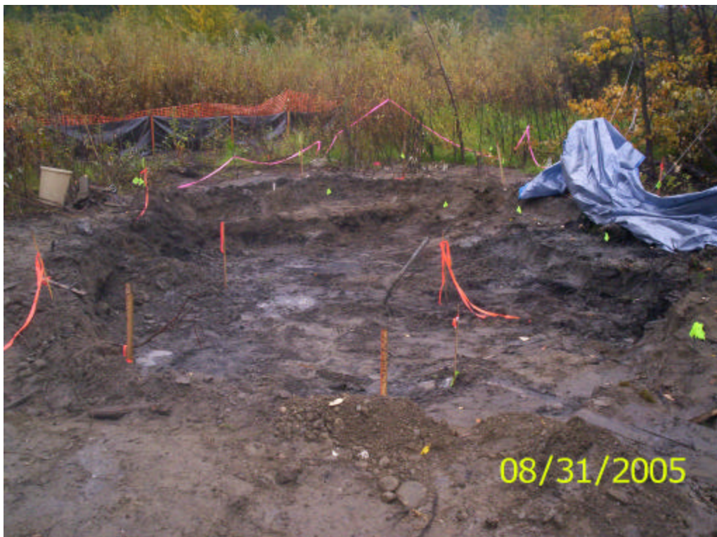
Photo 4. Inclusive contaminated area dug to 24 inches bgs.
