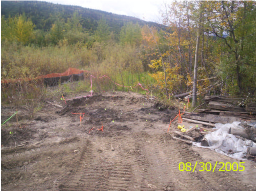
Photo 3. Inclusive contaminated area dug to 12 inches bgs.
