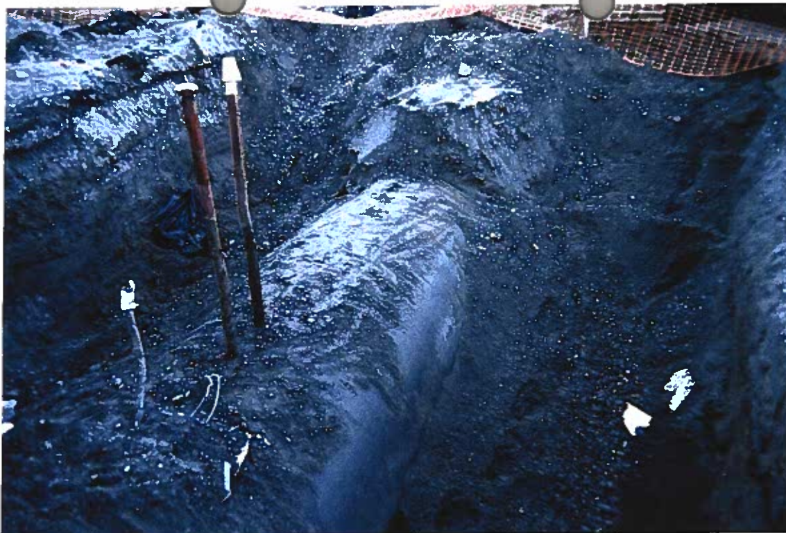
Photo 5: Looking east at the exposed 3,000-gallon heating oil tank. The final north side excavation wall was approximately six feet from the waste oil tank excavation.
