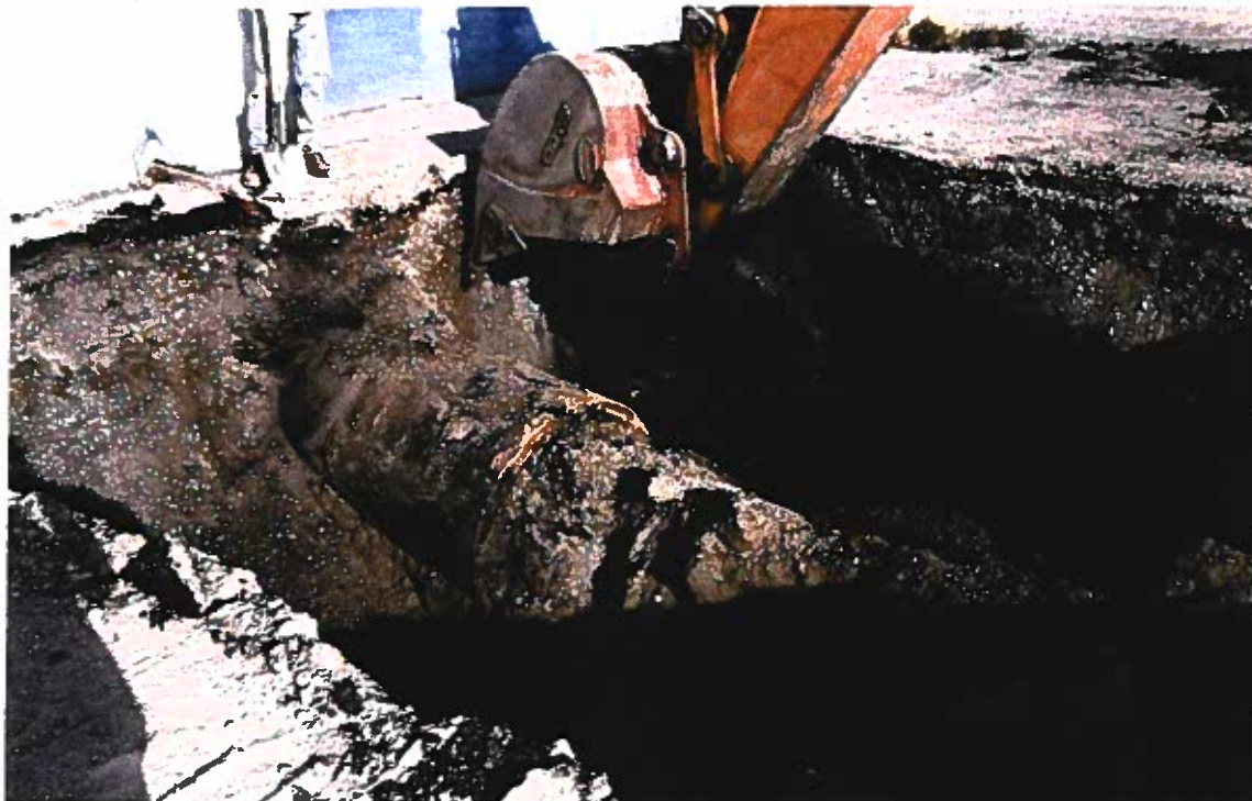
Photo 2: Looking northwest at the 500-gallon waste oil UST excavated on August 12, 1997. The gash located on the opposite side of the fill area was from the backhoe. The UST was pumped of waste oil prior to excavation and no waste oil leaked from the gash during removal.
