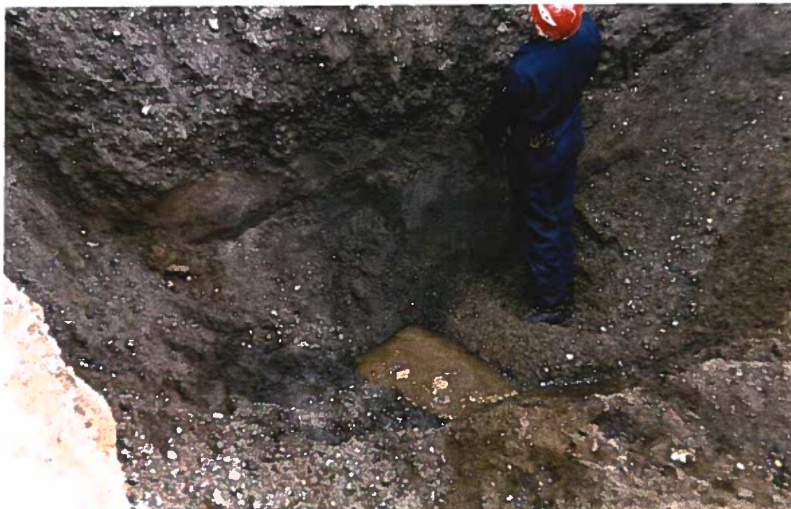
Photo 4: Looking northwest into the waste oil UST excavation. Groundwater was encountered at 10 feet below ground surface. Stained soils noticed at the sidewall (at the building foundation) are from fill pipe spillage down the outside of the tank.
