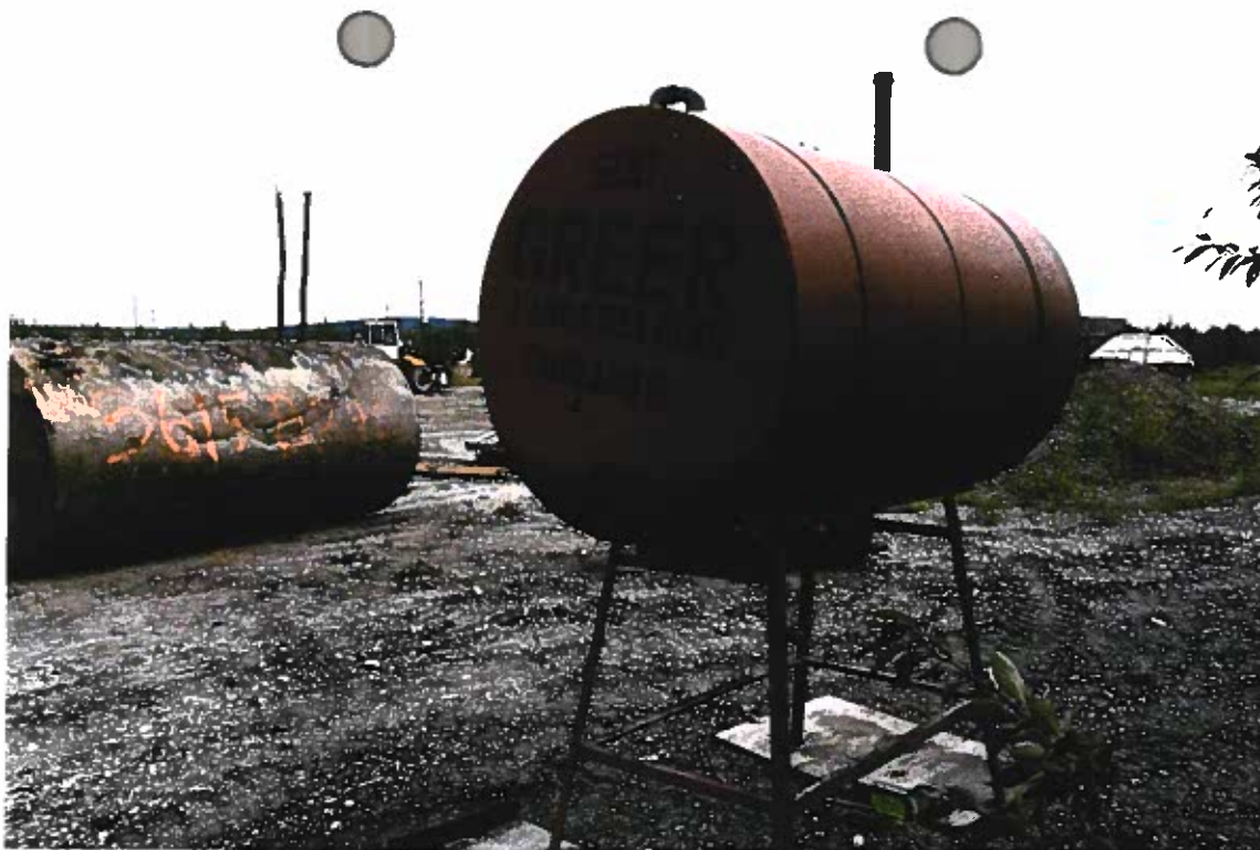
Photo 7: Looking northeast at the heating oil aboveground storage tank that was located in front of the warehouse on the south side of the warehouse addition. The stained area at the tank's bottom is thought to be where all the heating oil leaked. The 3,000-gallon heating oil tank is in the background.
