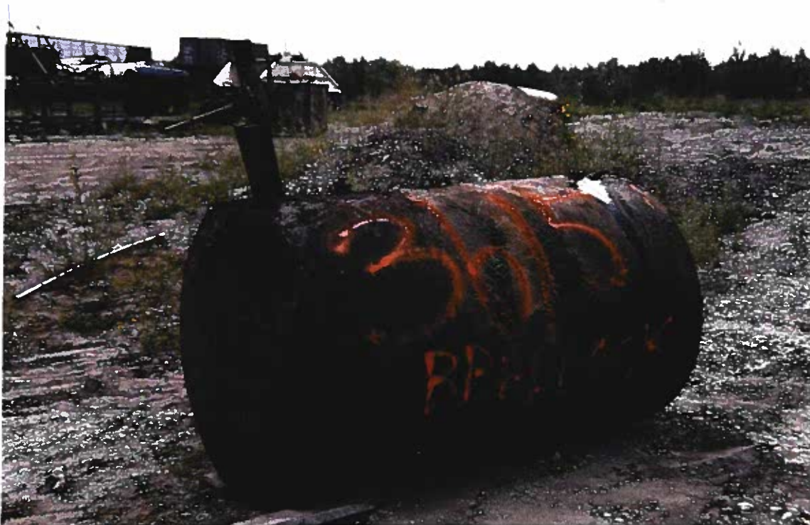
Photo 3: Looking northeast at the 500-gallon waste oil UST removed from behind the 3615 Braddock Street warehouse.
