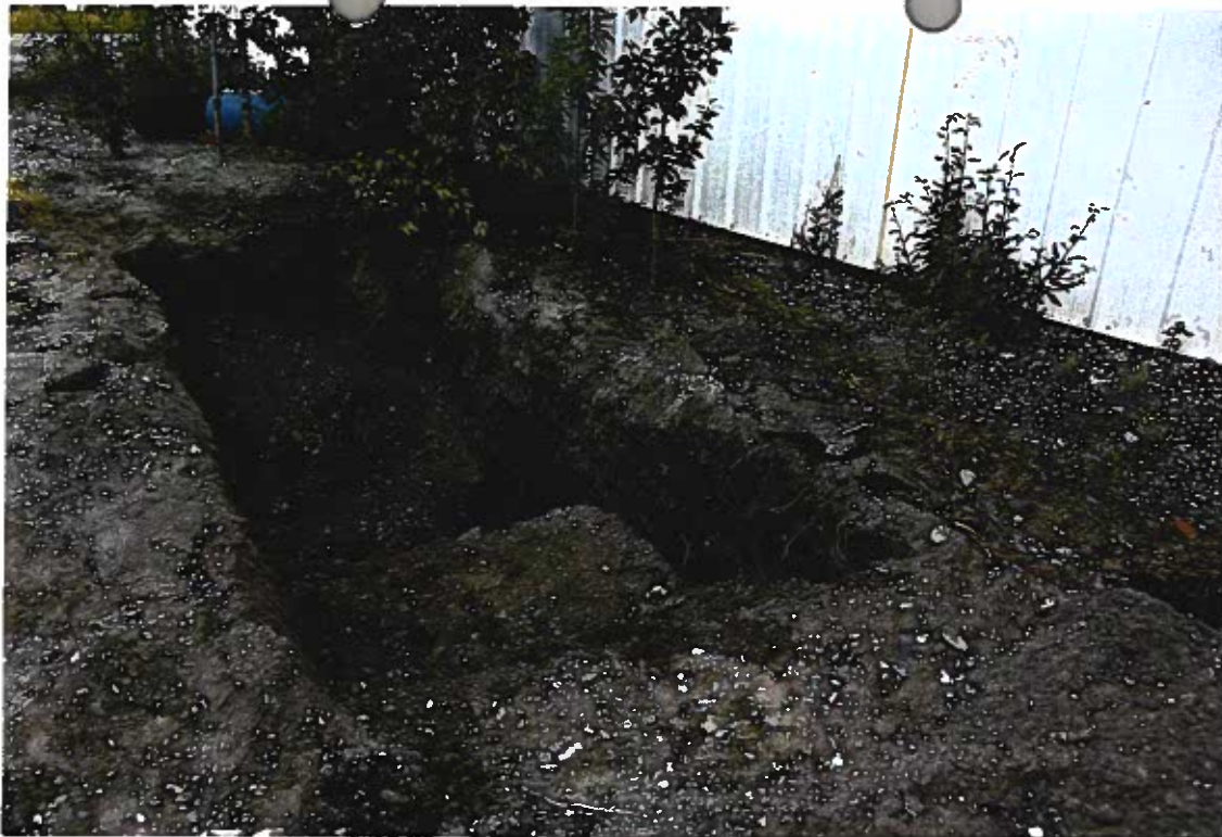
Photo 1: Looking northwest at the trench excavated in the "proposed" oil/water separator location on the south side of the building. No tanks or pipes were found and the oil/water separator was apparently never installed at this location.
