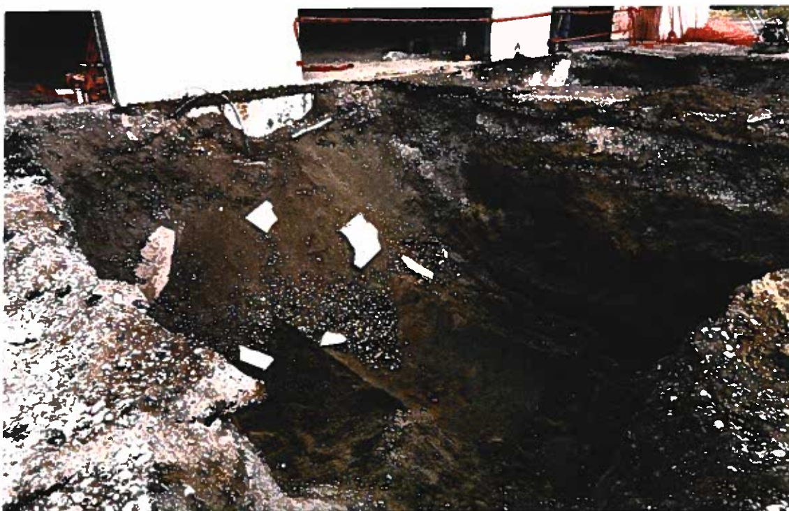
Photo 6: Looking northwest at the bottom impression of the 3,000-gallon heating oil tank removed. Final excavation limits are 25 feet long by 20 feet wide.
