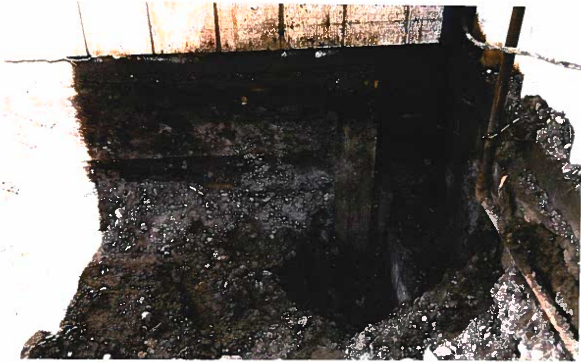
Photo 9: Looking at the northeast corner of the heating oil AST excavation. The corner is stained from dripping heating oil at fuel line fittings. Final excavation area was approximately 15 feet long by 13 feet wide, by 10 feet deep at its deepest. Groundwater was encountered at 10 feet below ground surface.
