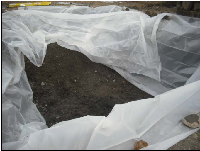
Photo 13: Excavation walls lined with polyethylene sheeting prior to backfill.
