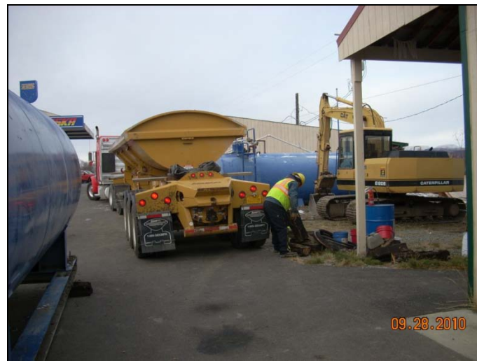
Photo 2: Preparing to excavate contaminated soil beneath storage tank, looking west.
