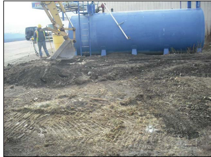
Photo 14: Backfilling excavation to replace tank.
