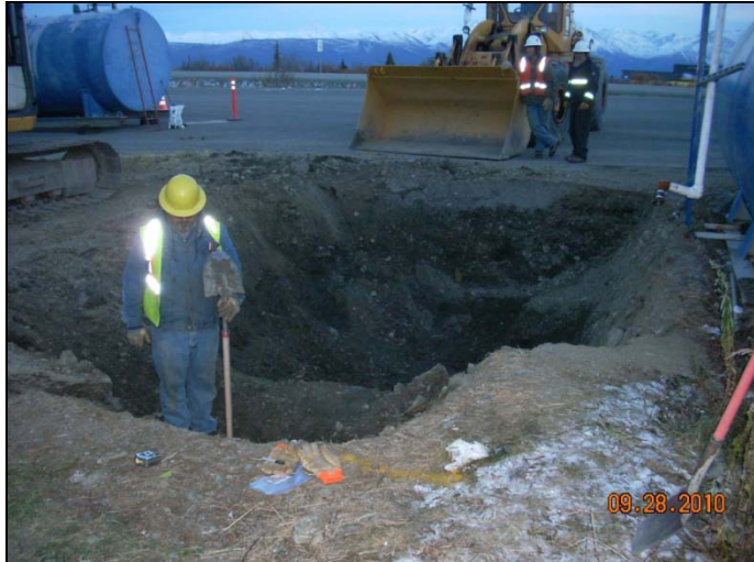
Photo 9: Excavation after filling third truck, showing screening sample location, looking southeast.
