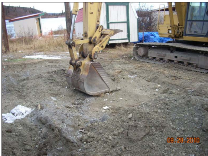
Photo 3: East tank pad prior to excavating, looking north.
