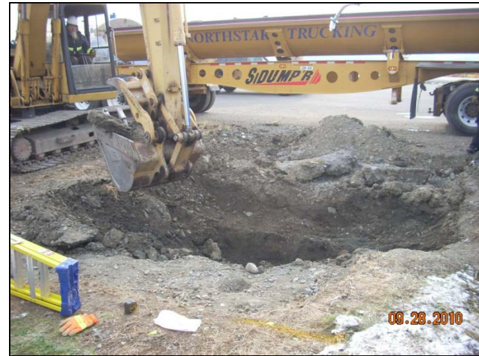
Photo 6: Excavating contaminated soil, looking southeast.
