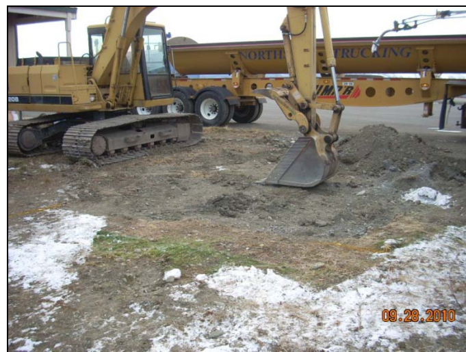
Photo 4: East tank pad prior to excavating, looking southeast.
