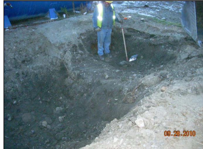
Photo 10: Excavation after filling third truck, showing screening sample location, looking northwest.
