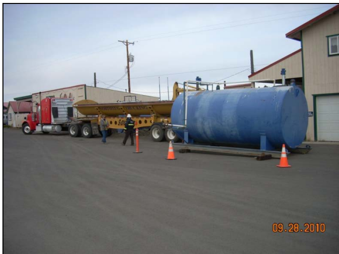
Photo 1: East tank temporarily moved for excavation, looking northwest.
