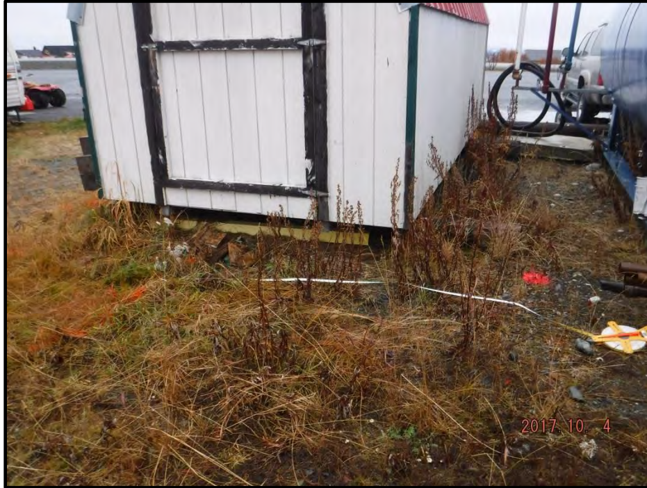
Photograph 9: Location of test boring 4, approximately 7 feet 5 inches away from communication line identified in orange.
