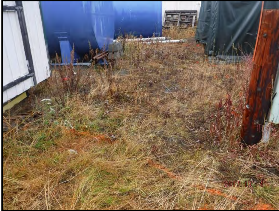
Photograph 3: Communication Lines from Utility Box leading under shed and west towards the site shop building.
