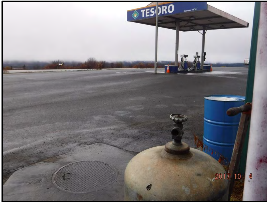
Photograph 5: Fuel Tank Sump located southwest of the fuel tanks.
