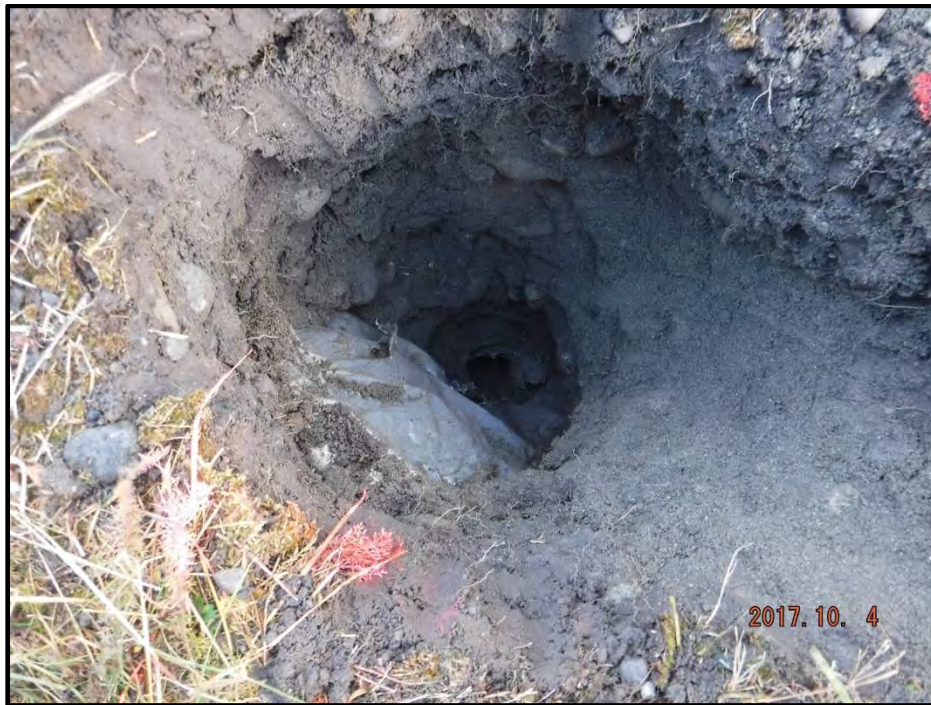
Photograph 8: Location of test boring 3. Plastic sheet identifying the extent of contamination was encountered at approximately one foot below ground surface.
