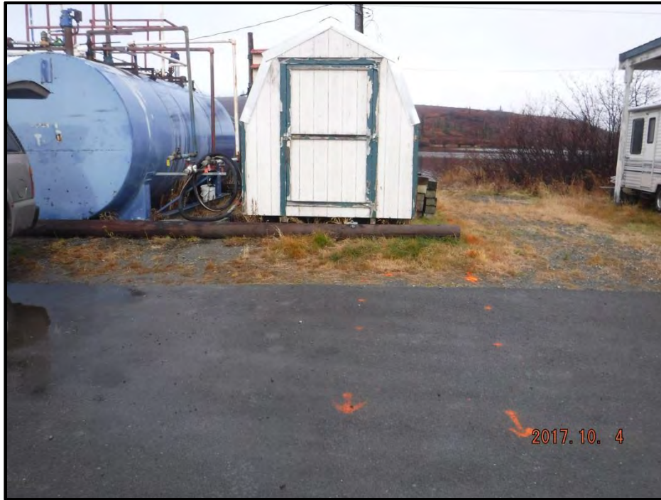
Photograph 1: Communication Lines marked by public utility locates. Picture was taken facing north.
