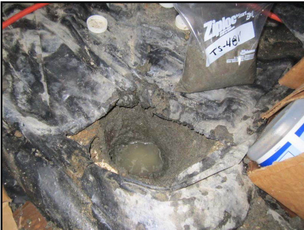
Photo 6: TS-4 soil boring location. Soil types and groundwater encountered.
