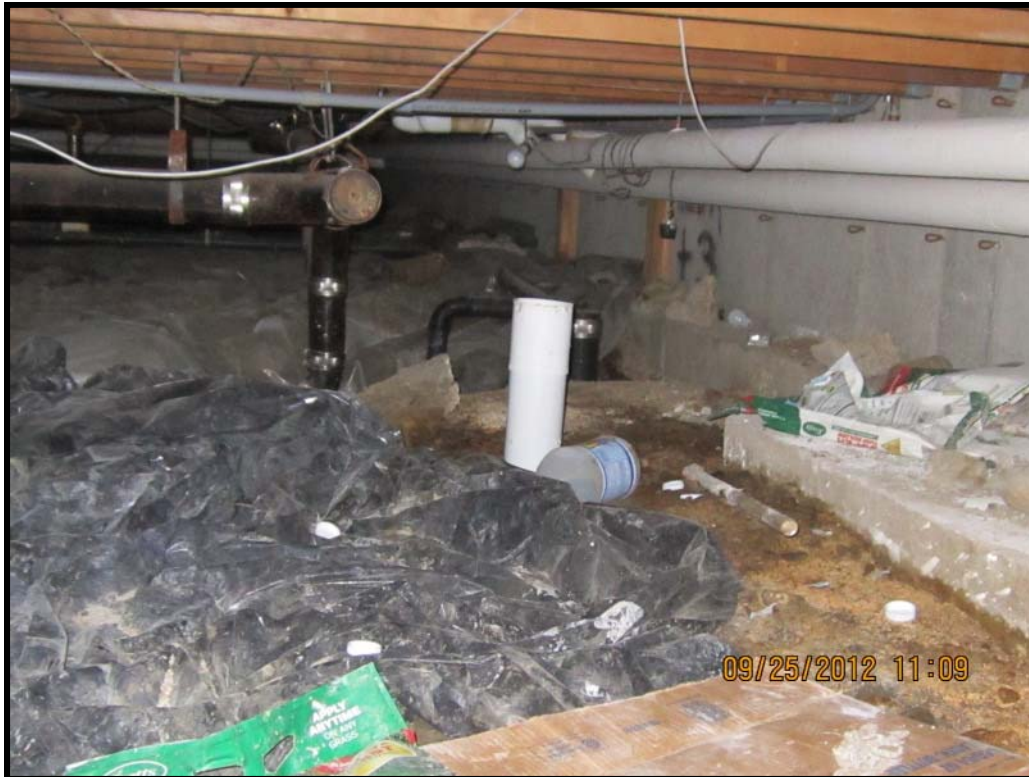
Photo 1: General Site conditions.
