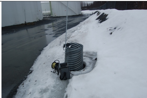
One dry well on the south side of the containment area.
