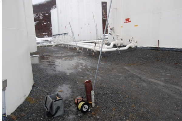
MW1 between tanks within the containment area.
