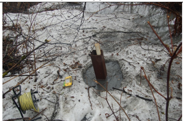
Damaged stand pipe on MW21.
