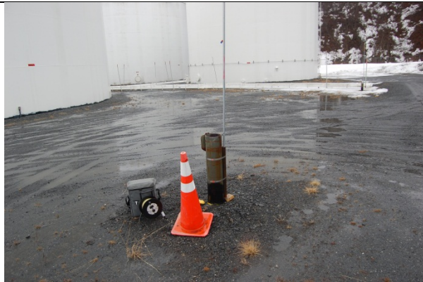
MW12 within the containment area.
