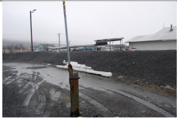
MW13 inside containment area.
