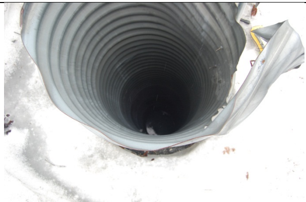
Inside the possible dry well.
