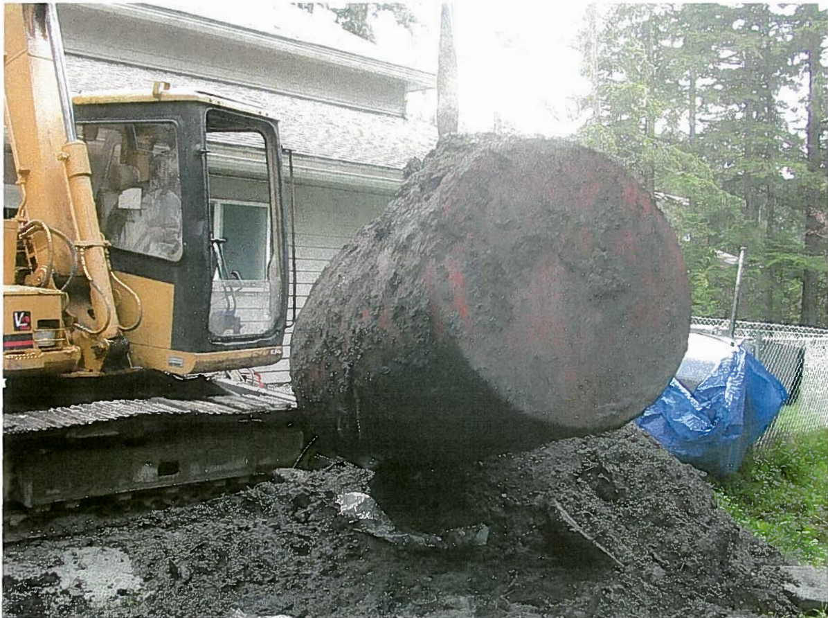
UST removed from 10481 Ann Coleman Drive
