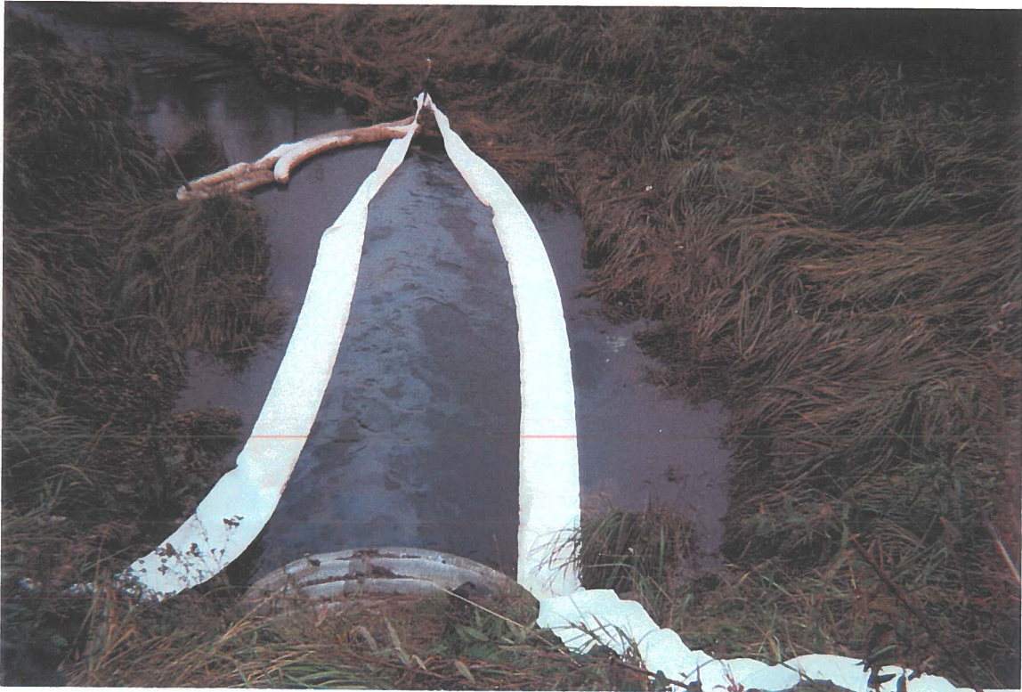
Sorbent boom and sweep deployed near the mouth of Duck Creek.
