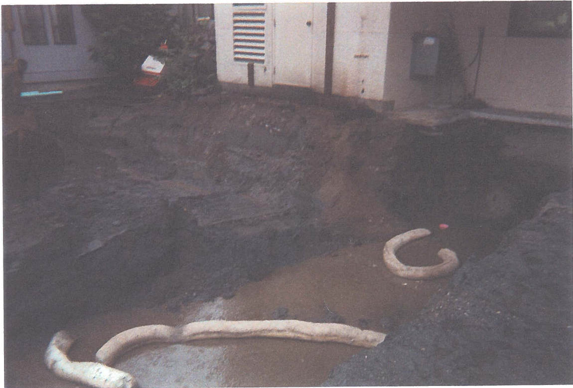
Contaminated soil excavation area, September 16, 2000.
