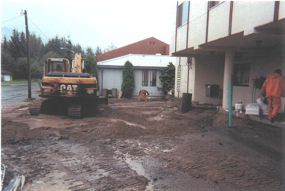
Backfilling the contaminated soil excavation area, note piping monitoring ports.
