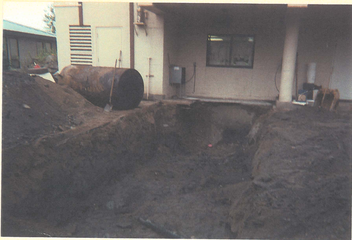
Excavation to remove the leaking UST, September 15, 2000.
