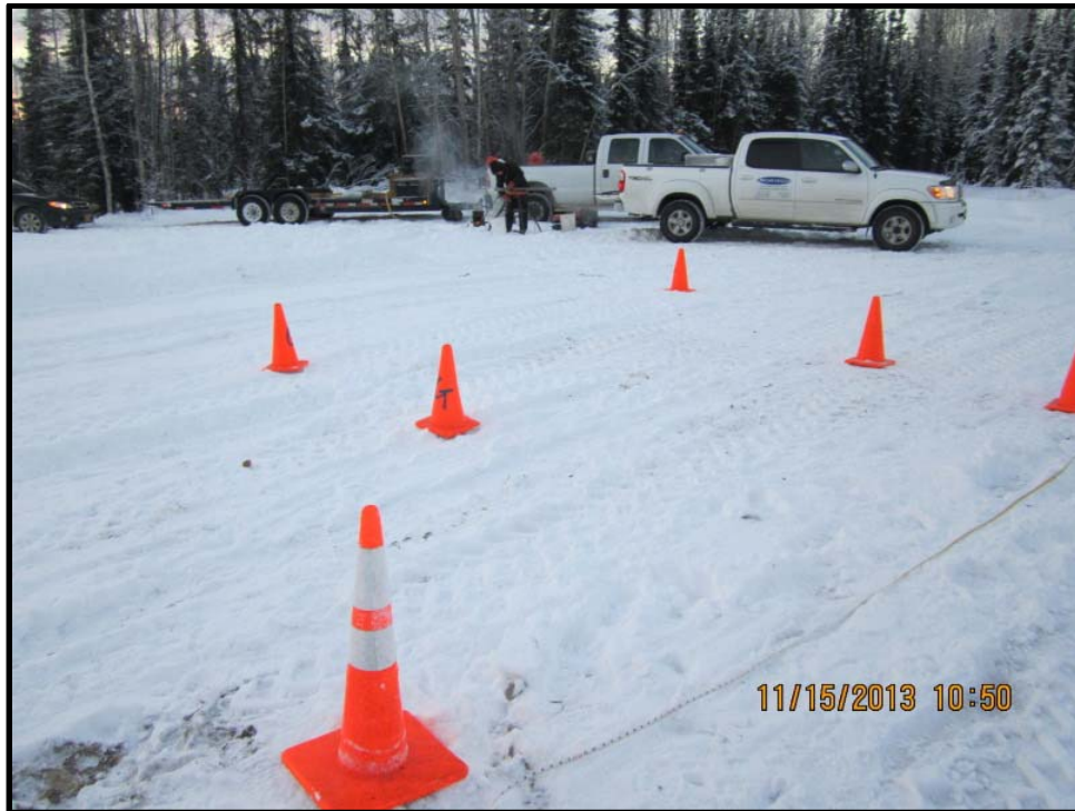
Photo 5: Looking southwest across former LIDAR Tower footprint with cones marking locations for installation of soil gas sampling ports with Geotek staff at decon station in background.
