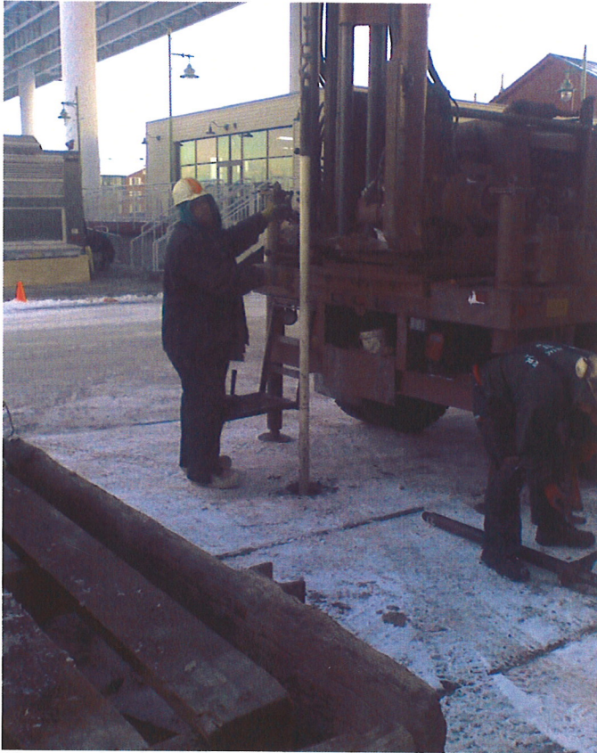
Photograph 1 Abandonment of MW-2 November 11, 2010.
