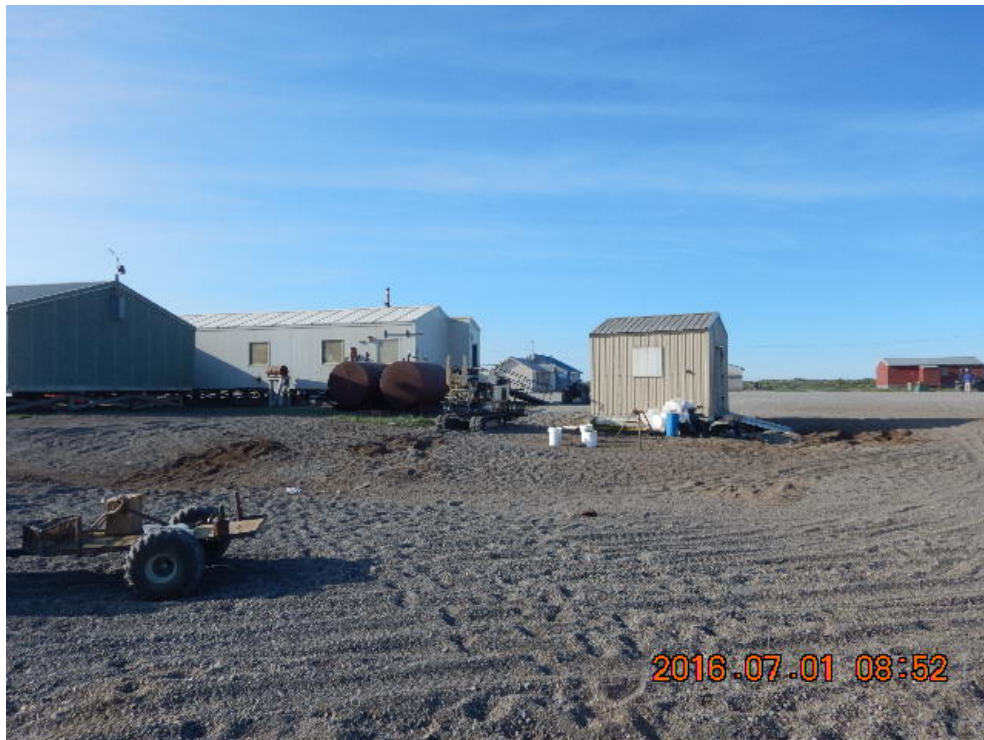
Photograph 6: The Gambell FSRC jobsite. Facing south.
