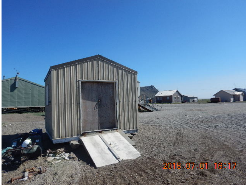
Photograph 11: Shed used for swing tie measurements. Facing east.
