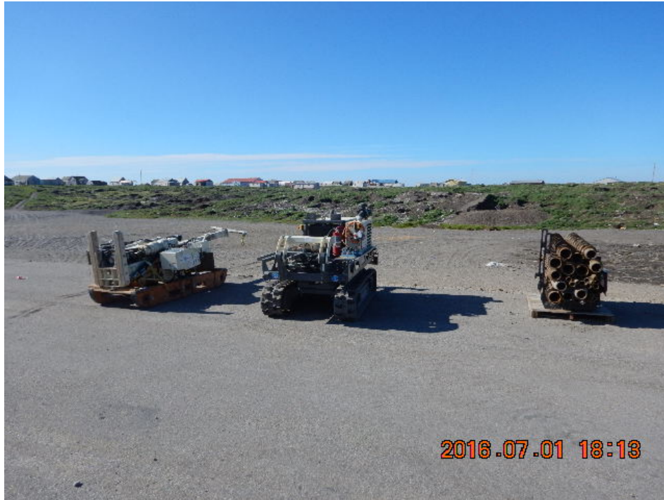
Photograph 13: Drill rig and tooling staged at the airport for pick-up by the Sherpa. Facing north.
