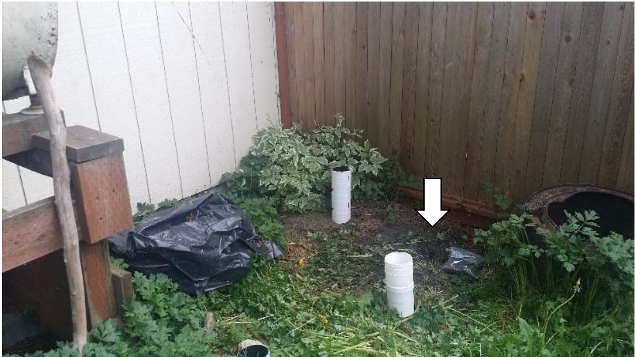
Photo 3: Location of soil boring S3 in relation to nutrient ports and the AST.
