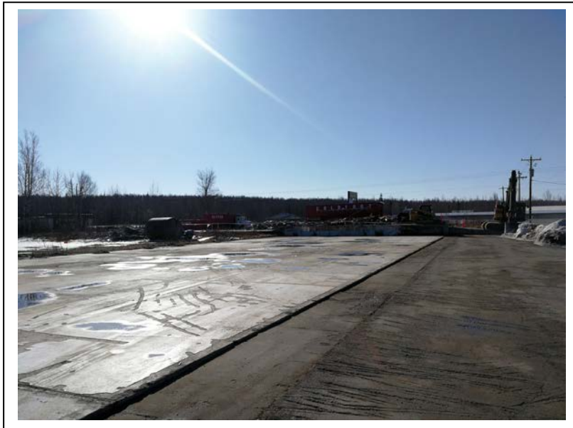
Photo 3: Looking northwest at the concrete slab. (March 28, 2019 – photo provide by Coldfoot)
