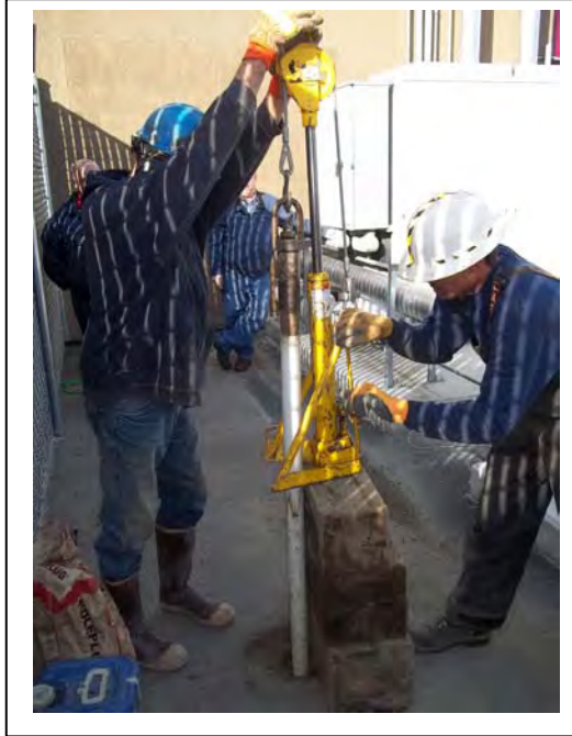
Photo 5: Monitoring Well B10MW was pulled up with a hydraulic jack. (September 16, 2013)
