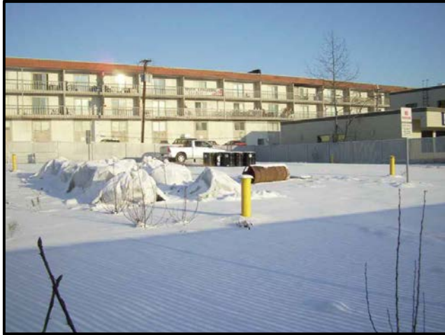
1. Site layout looking Northeast
