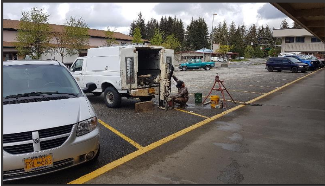
Photo 3: View looking northwest at sample location BH-03/MW-3. This is located on the west side of the building.
