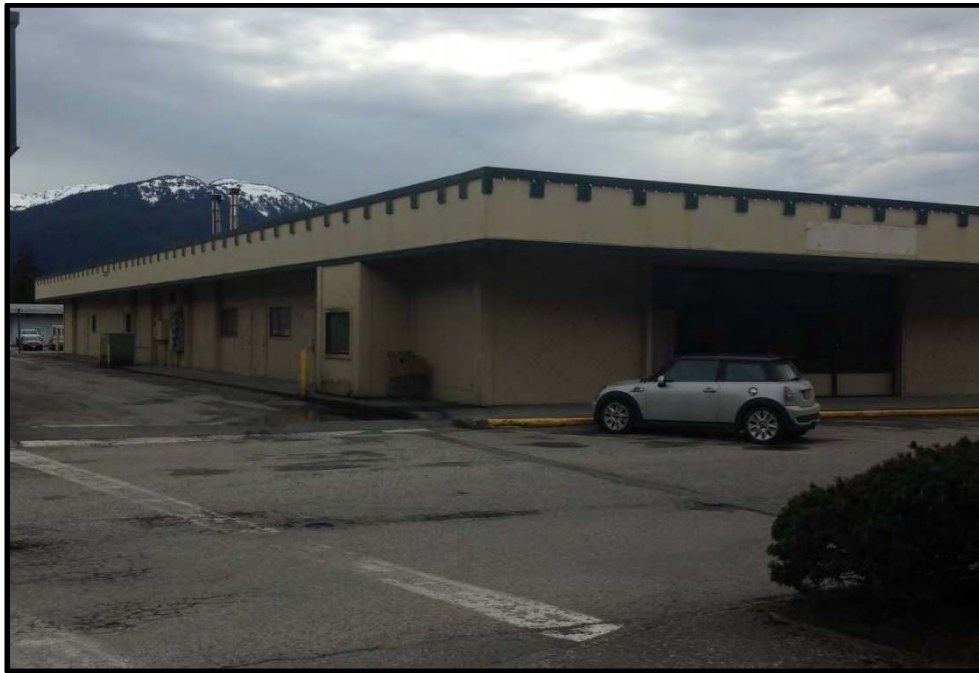
Photo 1: Looking southwest at the northwest corner of the building (suite 550).
