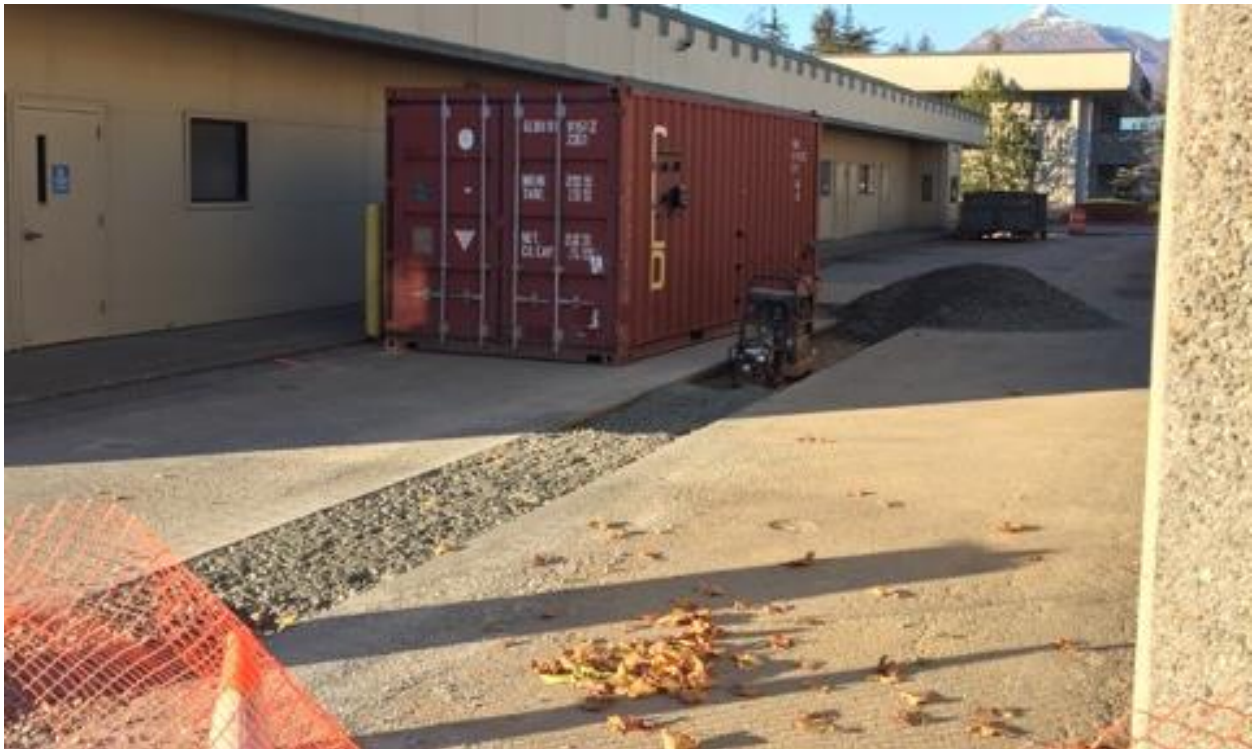
Backfilling of SVE trench and SVE treatment container
