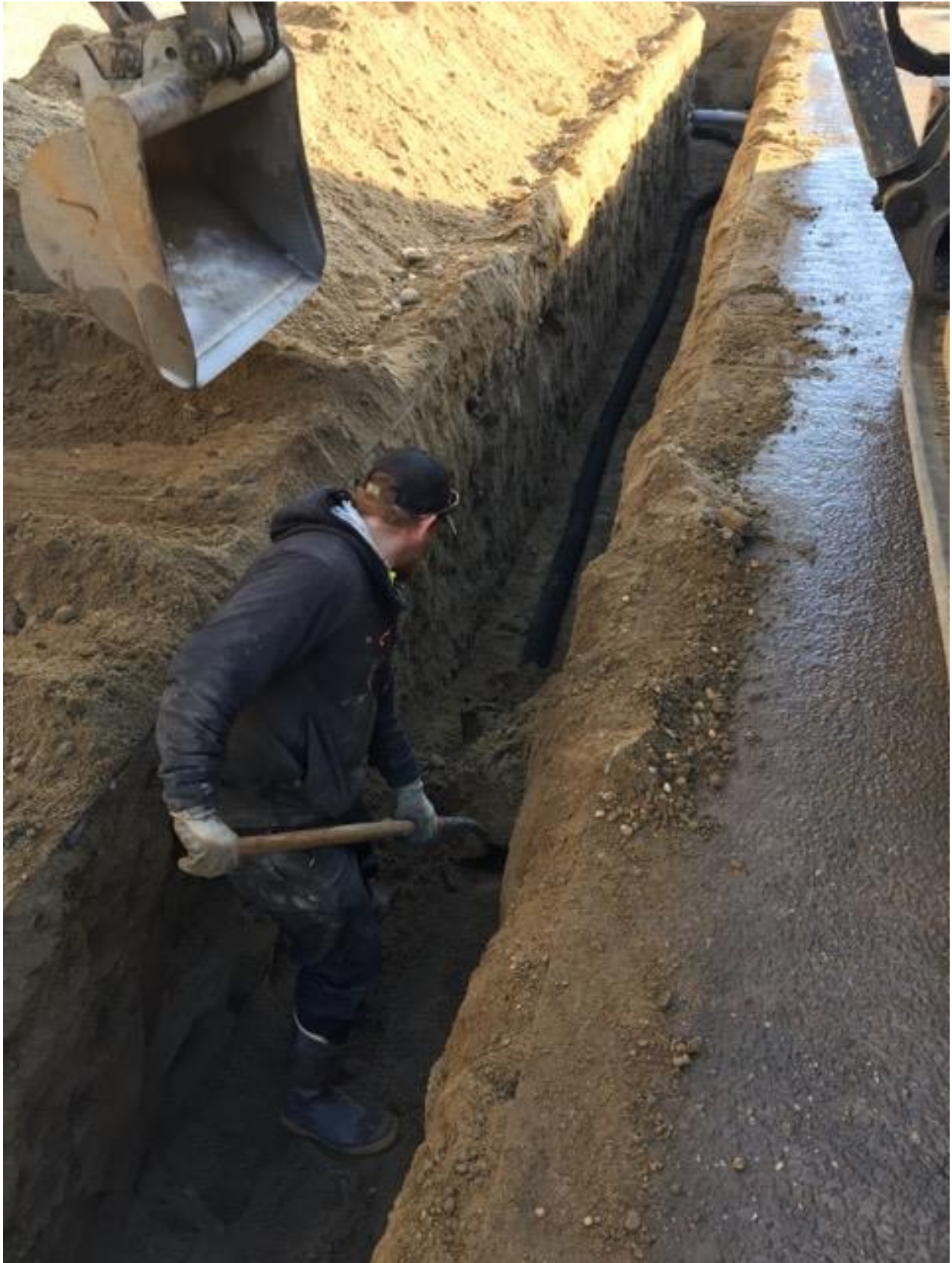
Trench with SVE piping
