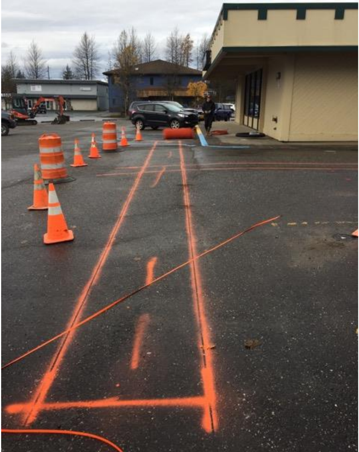
Marking for SVE trench
