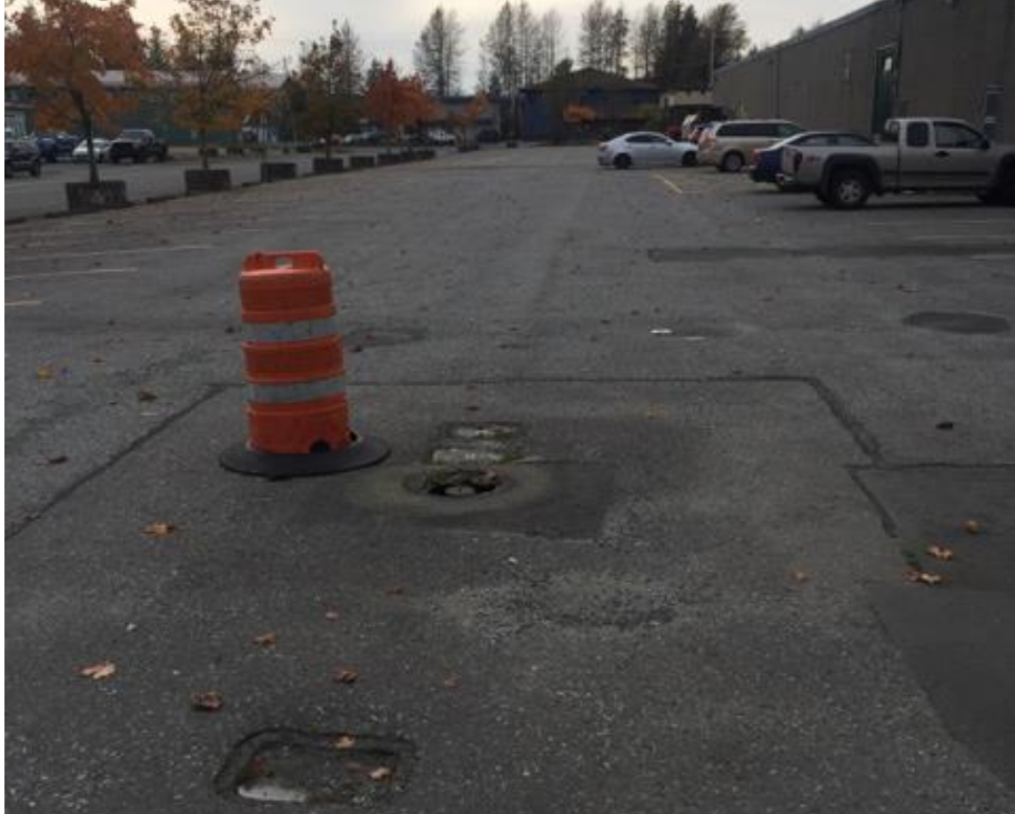
Location of Diesel UST
