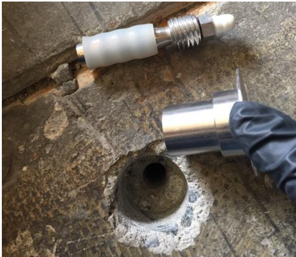
Subslab Vapor Pin Installation (SS5)
