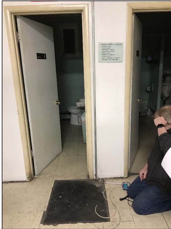
Photo 3: Measuring different pressure between occupied space and utilidor. Basement boiler room is present beneath the bathroom at back of photo.
