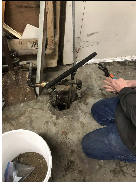
Photo 1: Hole in the concrete slab that was reportedly used for fluid disposal. Pipes coming from the hole appear to be the connection to the public water utility and the “T” handle is the hand auger that was used to collect soil samples for field screening and laboratory testing from below the concrete slab. Recovered soil is visible in the bucket.
