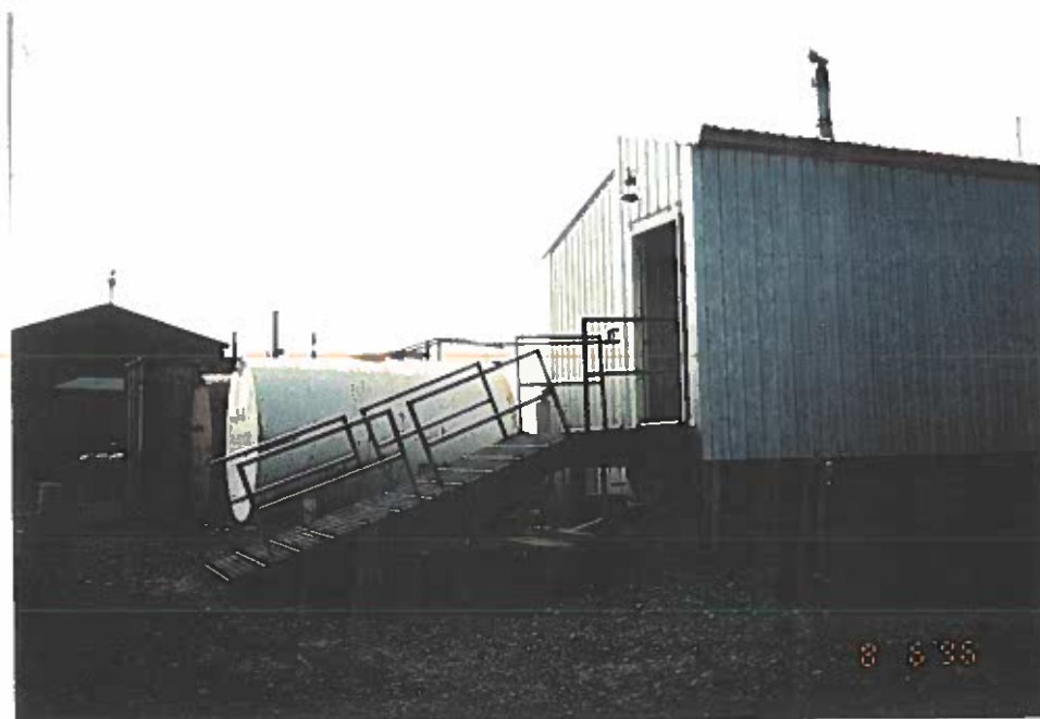
Front of Old Armory. Looking Southwest.
