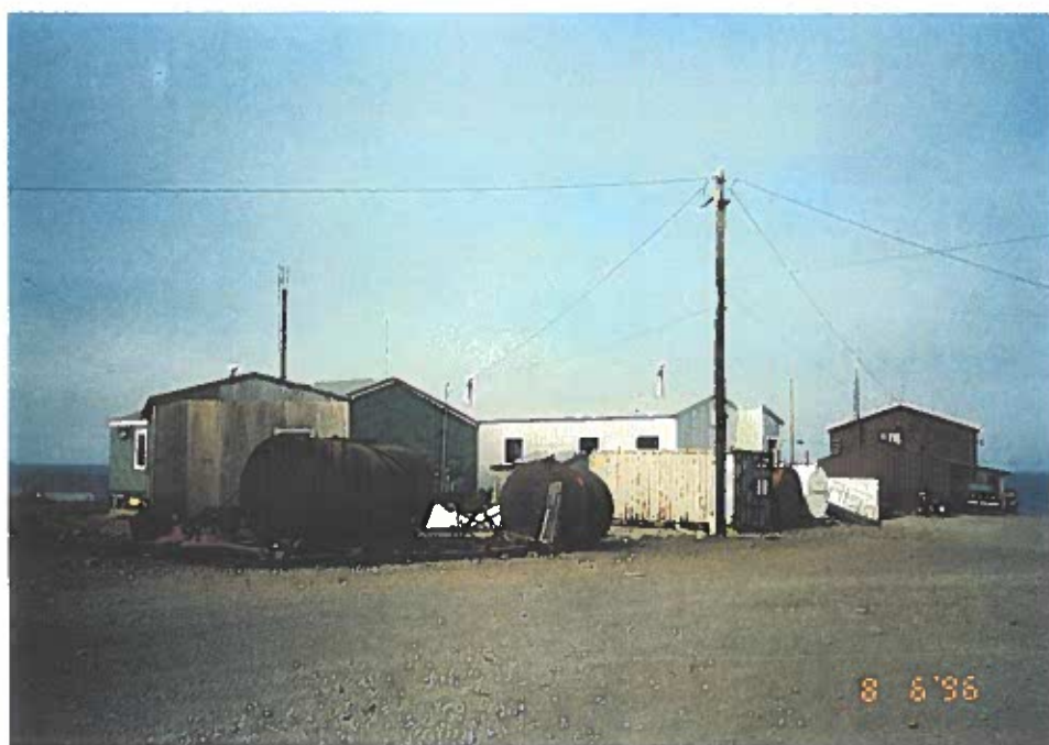
Road in Front of Armory. Looking North.
