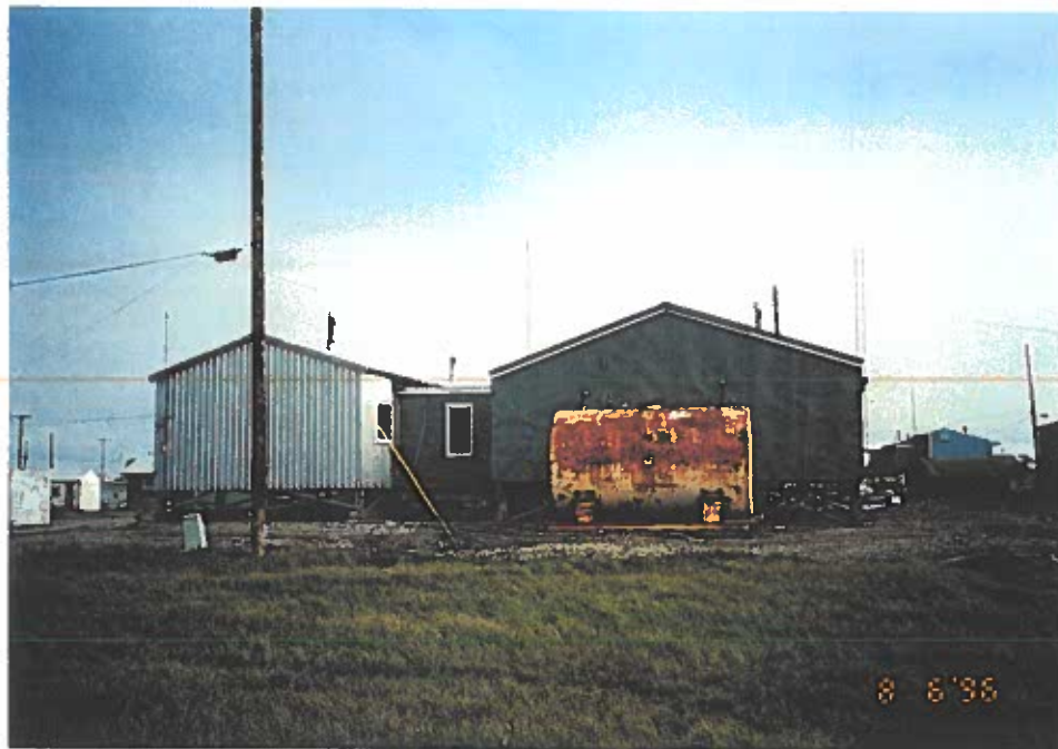
Back of Armory. Looking Southeast at Heating Oil AST.
