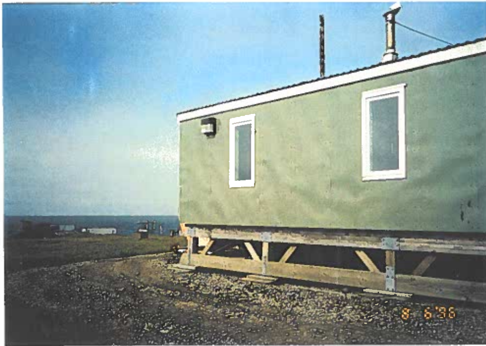
Southwest Side of Armory. Looking North.
