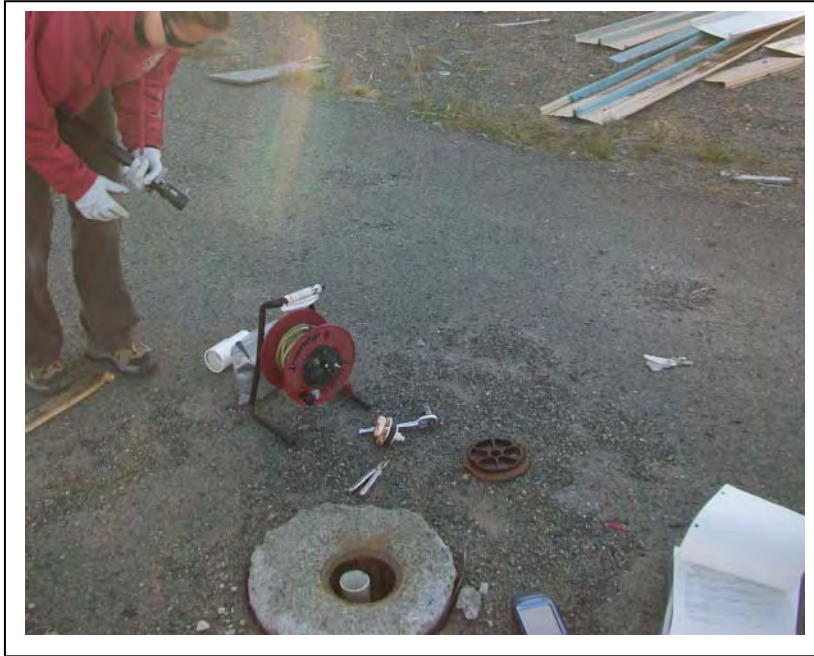
Photo 5: Looking northeast, the former MarkAir Monitoring Well MW-7 frost jacking caused the cement embedding to separate from the adjacent asphalt surface. (5/19/2010)
