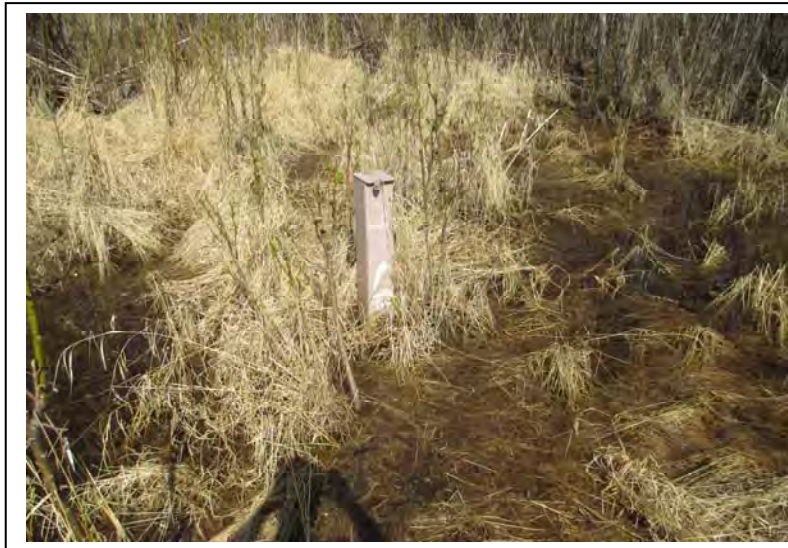
Photo 4: Looking north, Monitoring Well RA-MW6 is located in an area of standing surface water at the Runway Apron area. (5/13/2014)
