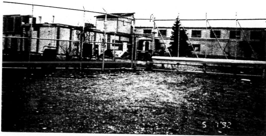
PHOTO # 1 GOOSE BAY CORRECTIONAL FACILITY
