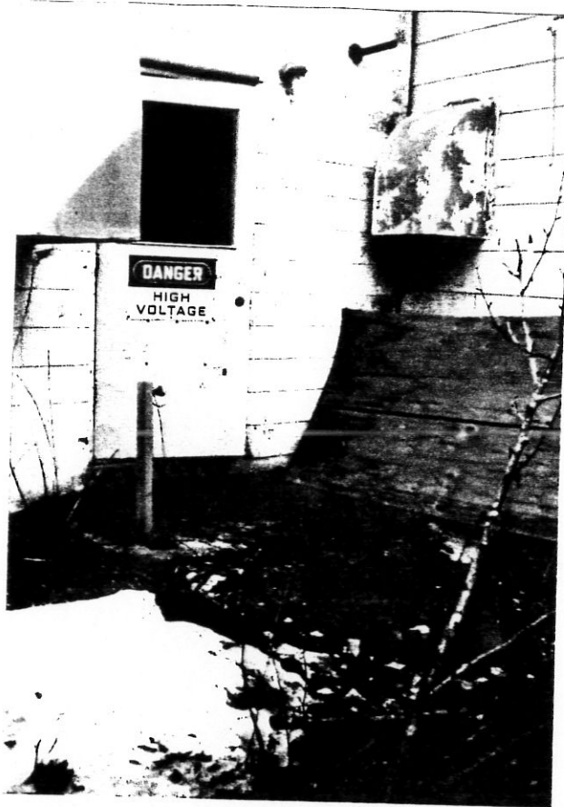
PHOTO # 5 GOOSE BAY NIKE MISSILE SITE OUTSIDE DOOR TO GENERATOR BUILDING-OIL SPILL
