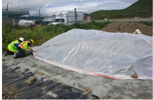
Covering of the soil stockpiles following sample collection.
