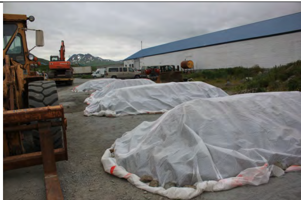
Covered soil stockpiles.
