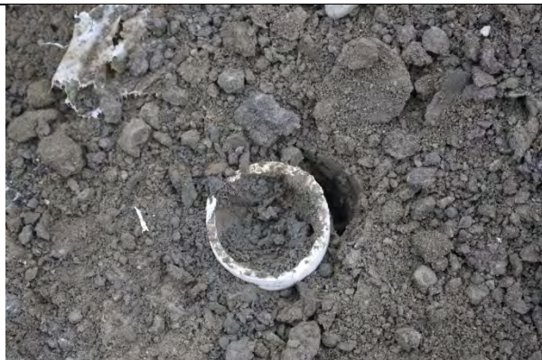
The damaged, broken, and filled MW-3.
