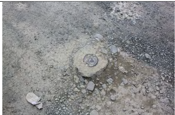
MW-1 well cover and concrete pad.
