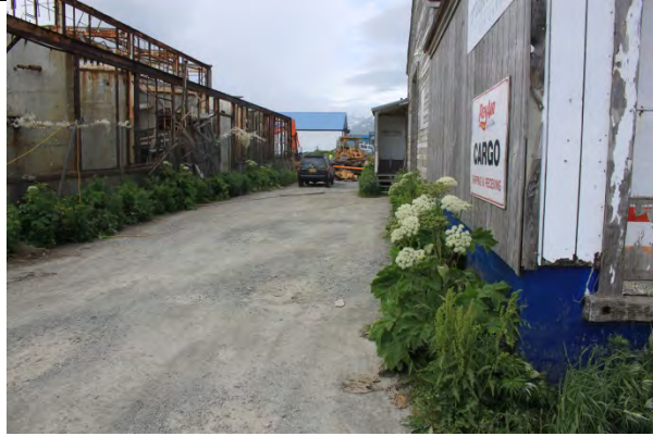
Location of MW-1 looking along Torpedo Building.
