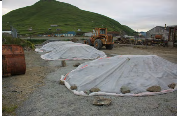
Covered soil stockpiles on site.
