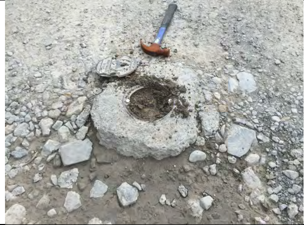
Removing compacted soil around MW-1 cap.
