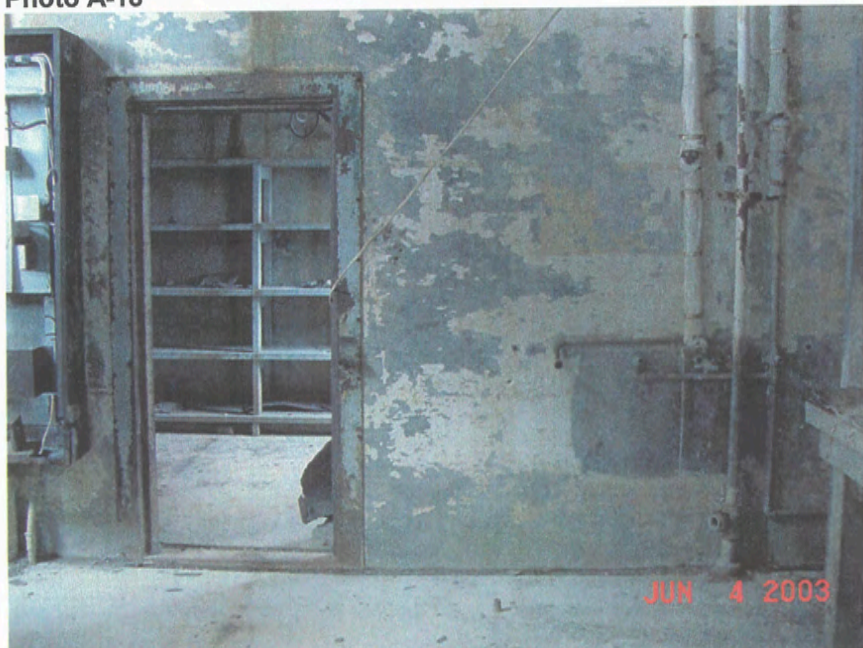
Looking through doorway toward west elevation, Room 108-Bombsight Storage, June 2003
