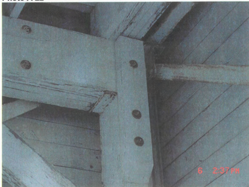
Detail of wood framing construction, Room 111-Loft, June 2003
