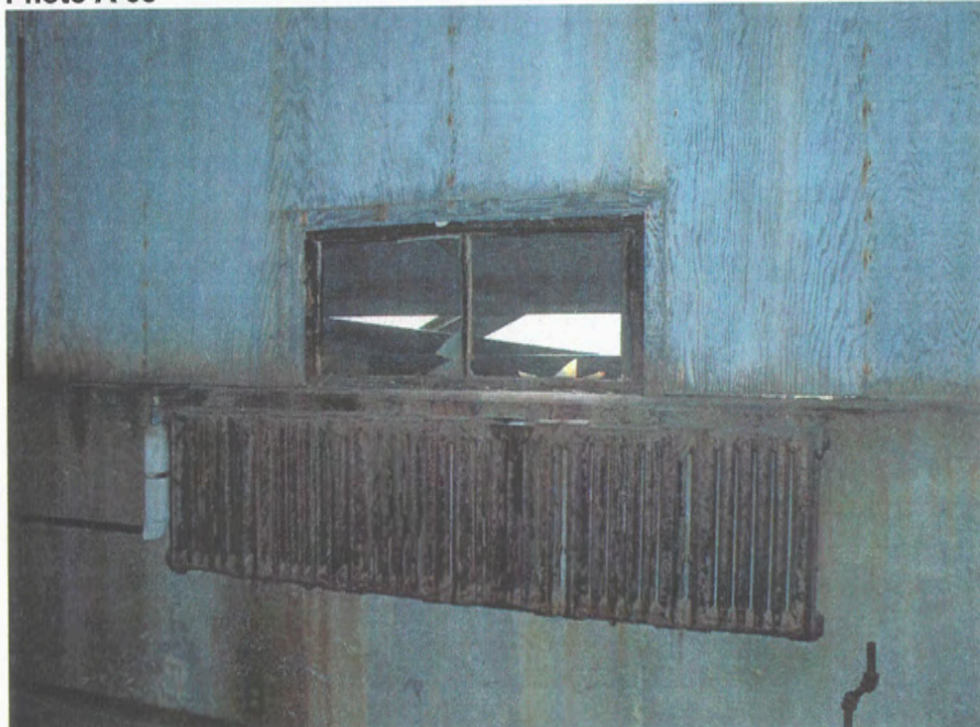
North elevation of Room 100-Office, June 2003
