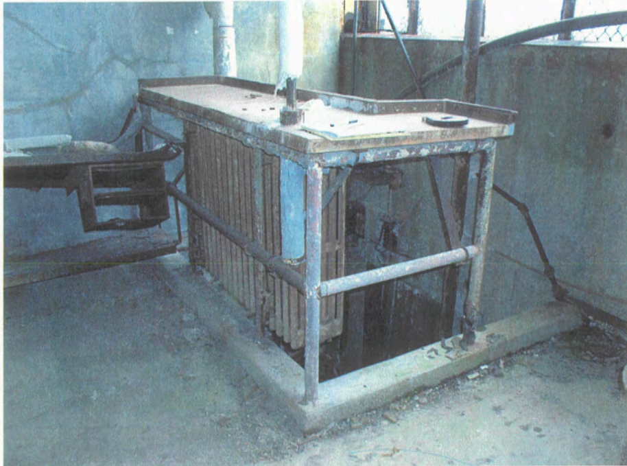
Boiler Pit, Northwest corner of Room 104-Tool & Storage, June 2003
