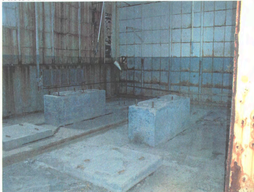
Southwestern corner, Room 113-Compressor Room, June 2003
