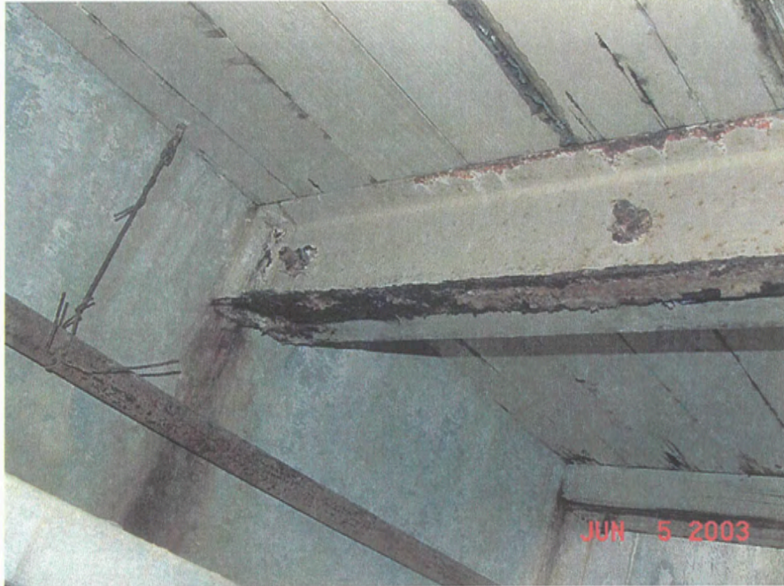
Grid 5.75/C.25 – Mechanical floor, wood beam bolted to steel channel, June 2003
