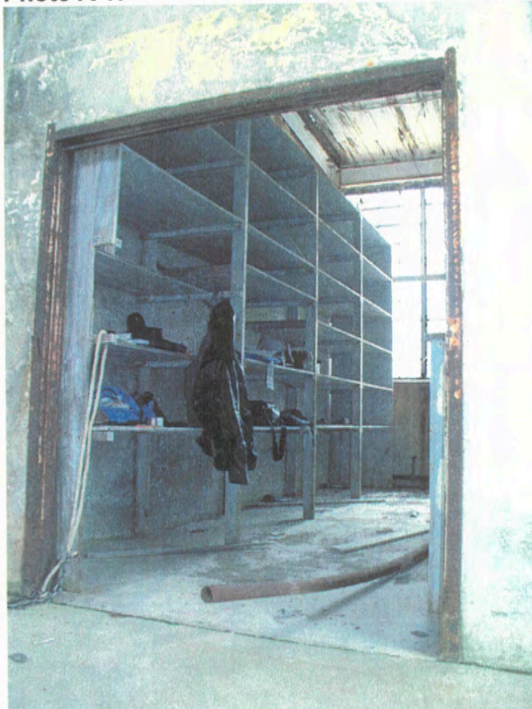
Looking through doorway toward north elevation, Room 107-Ordnance Storage, June 2003
