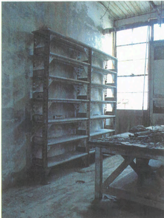
Northwest corner of Room 105-Battery Room, June 2003
