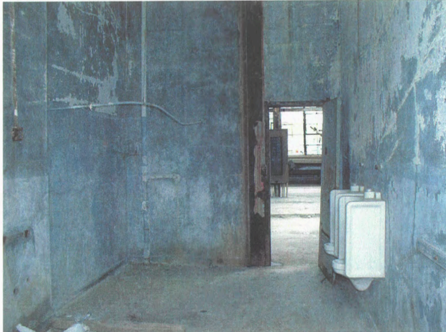
South elevation of Room 103-Toilet, June 2003
