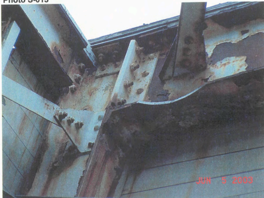
Grid 7/C – Northeast corner of central H roof, June 2003
