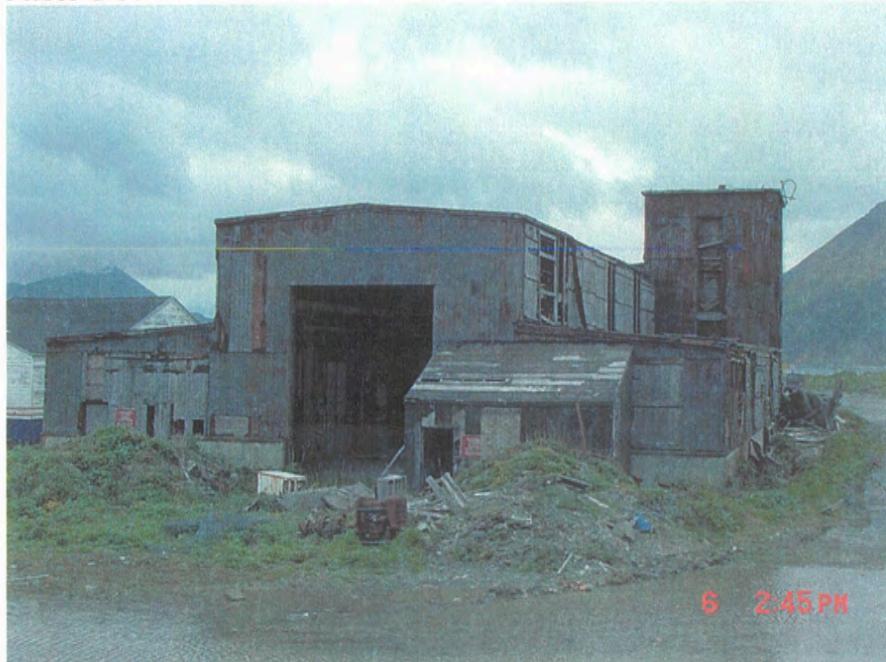
Southwestern exterior elevation, June 2003
