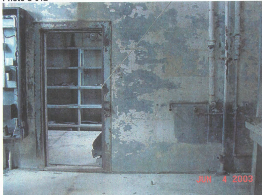
Grid 6/C – interior elevation, south side of concrete shear wall, June 2003
