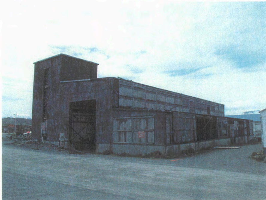
Northeastern corner of building, June 2003
