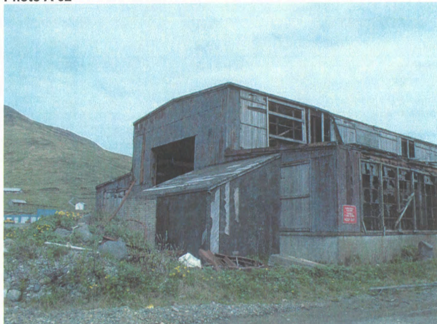
Wood-frame addition to south elevation, June 2003
