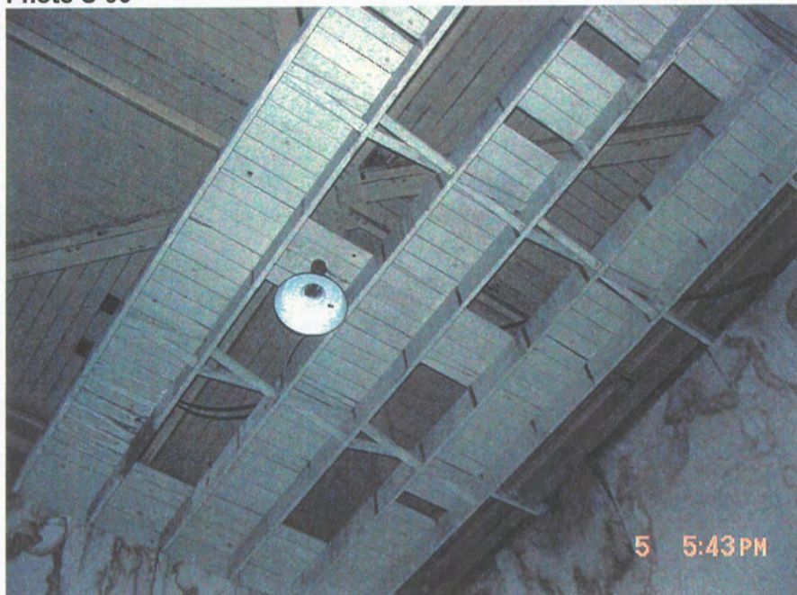
Grid 6-7/A-B – parachute loft roof deck/framing from below, June 2003
