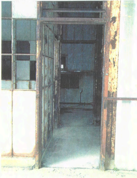
North elevation of Room 102-Passage, June 2003
