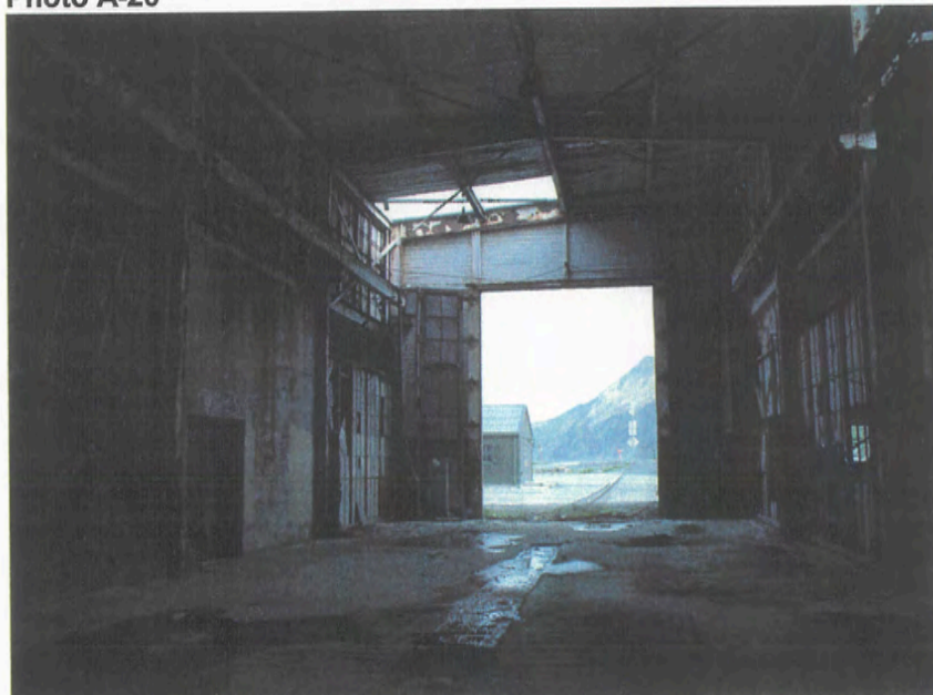
Looking east, Room 110-Craneway, June 2003
