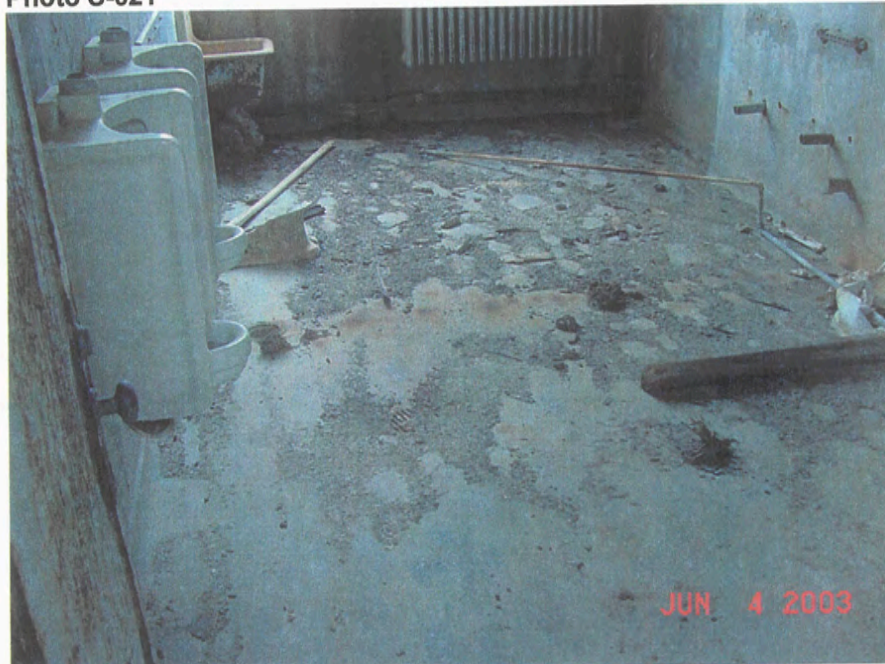
Grid 2/C-D – slab on grade, toilet room, June 2003
