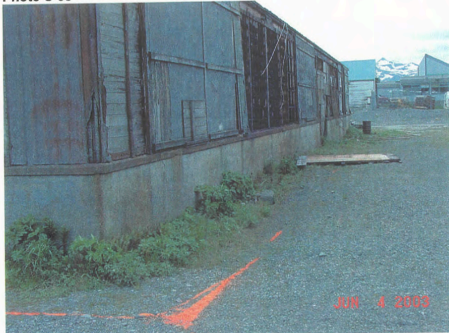
Grid D – typical exterior concrete wall, June 2003
