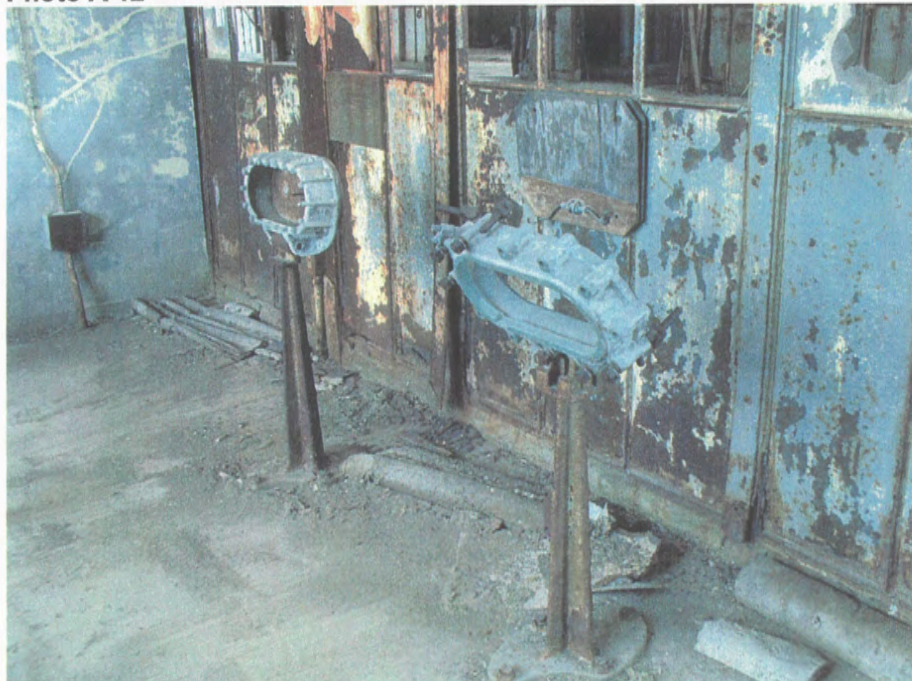
Southwest corner of Room 104-Tool & Storage, June 2003
