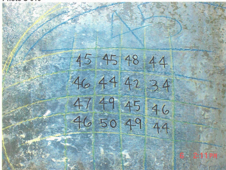
Grid 5/D – concrete wall west face; reinforcing size and spa, June 2003
