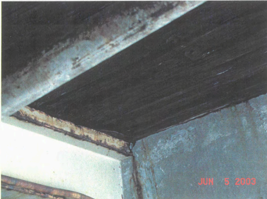
Grid 5.5/C.5 – W-beam through concrete wall, June 2003
