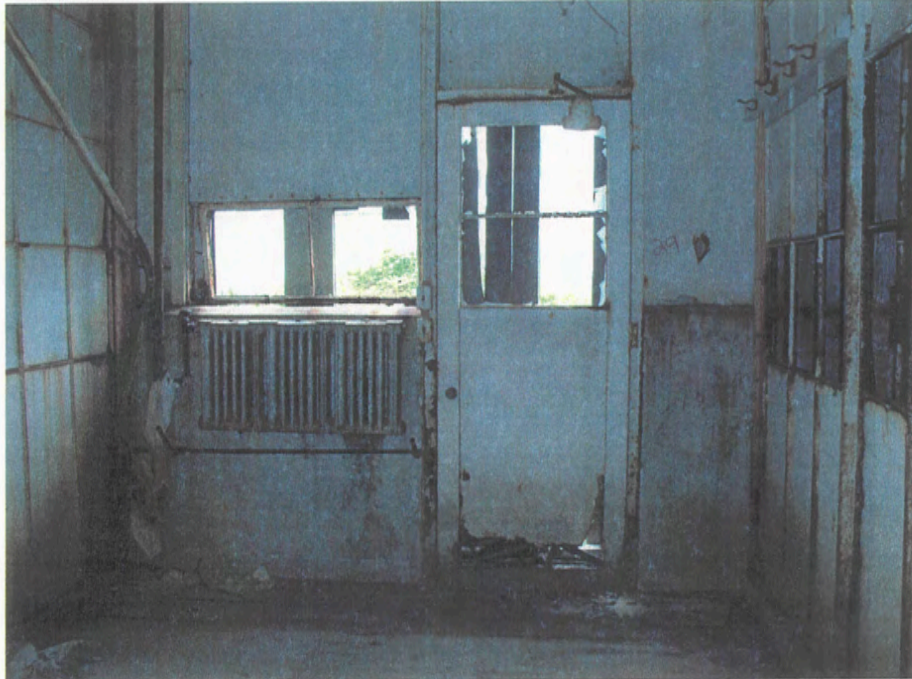
West elevation of Room 101-Office, June 2003
