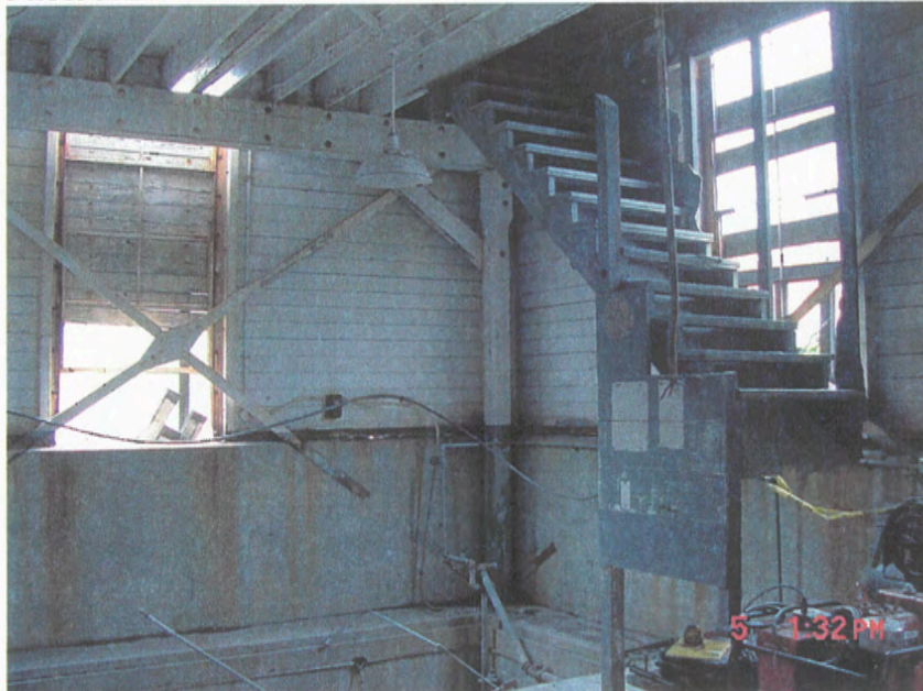
Southeastern corner at stair to Room 111-Loft, June 2003
