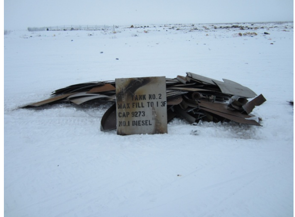
Fully cut and removed fuel tank.
