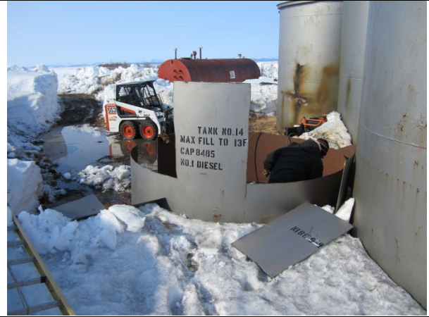
Cutting of fuel tanks at the barge landing site.
