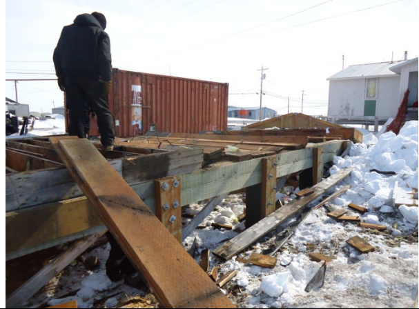
Structural demolition of foundation.
