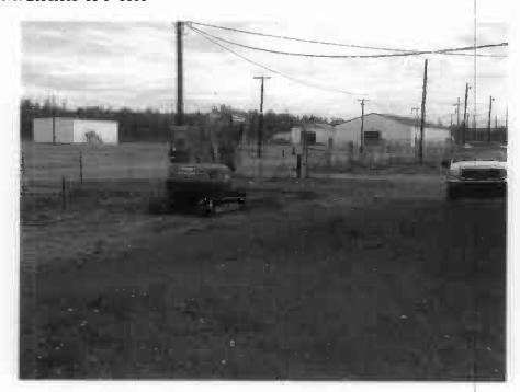
A small excavation of the original utility trench was done with the Hatachi EX55 excavator to expose conduit and cable on May  $27^{th}$ . Telephone cable and 1 inch electrical conduit were pulled and disposed of at Anchorage Municipal Landfill. The excavation was backfilled after cable and conduit were removed.
