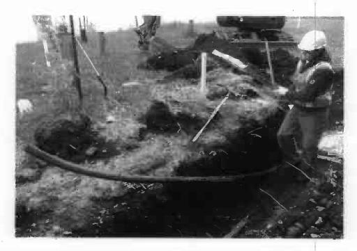
Sod (2-4 inches thick) was removed and placed in a separate stockpile for replacement following backfill. Areas around vapor extraction wells were exposed approximately 3 to 4 feet in diameter in preparation for decommissioning by subcontractor Denali Drilling. Trenches and excavation were backfilled and graded on the 26<sup>th</sup> and 27<sup>th</sup> of May.
