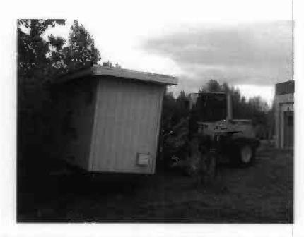
Blower building anchors were excavated and exhaust stack removed. Building and exhaust stack were relocated with the loader to the staging area behind Building 955.
