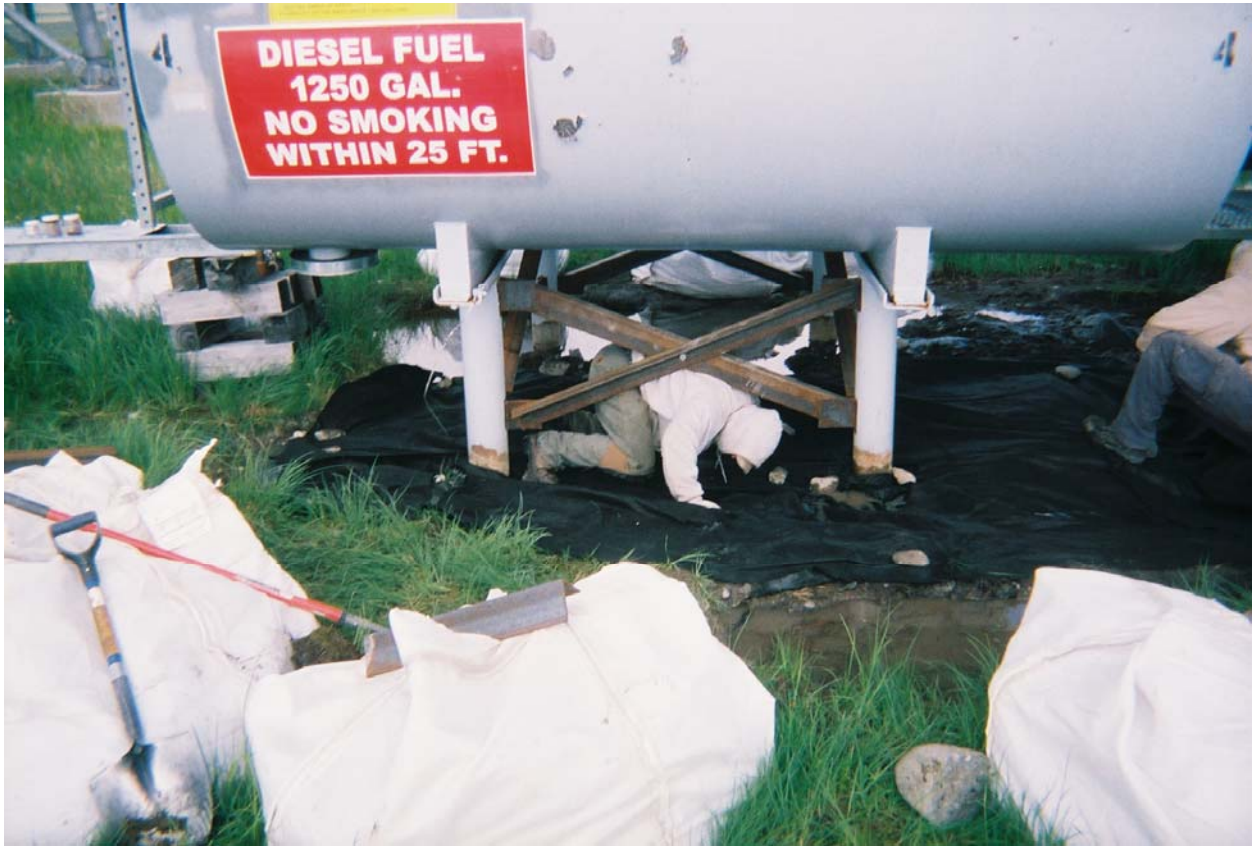
Installing geofabric liner beneath AST 4 and AST 1. Looking north.
