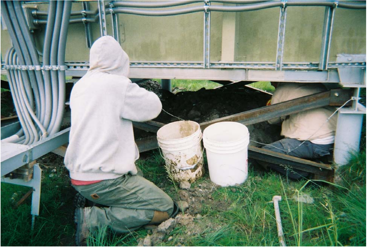
Generator module excavation in progress. Looking west.
