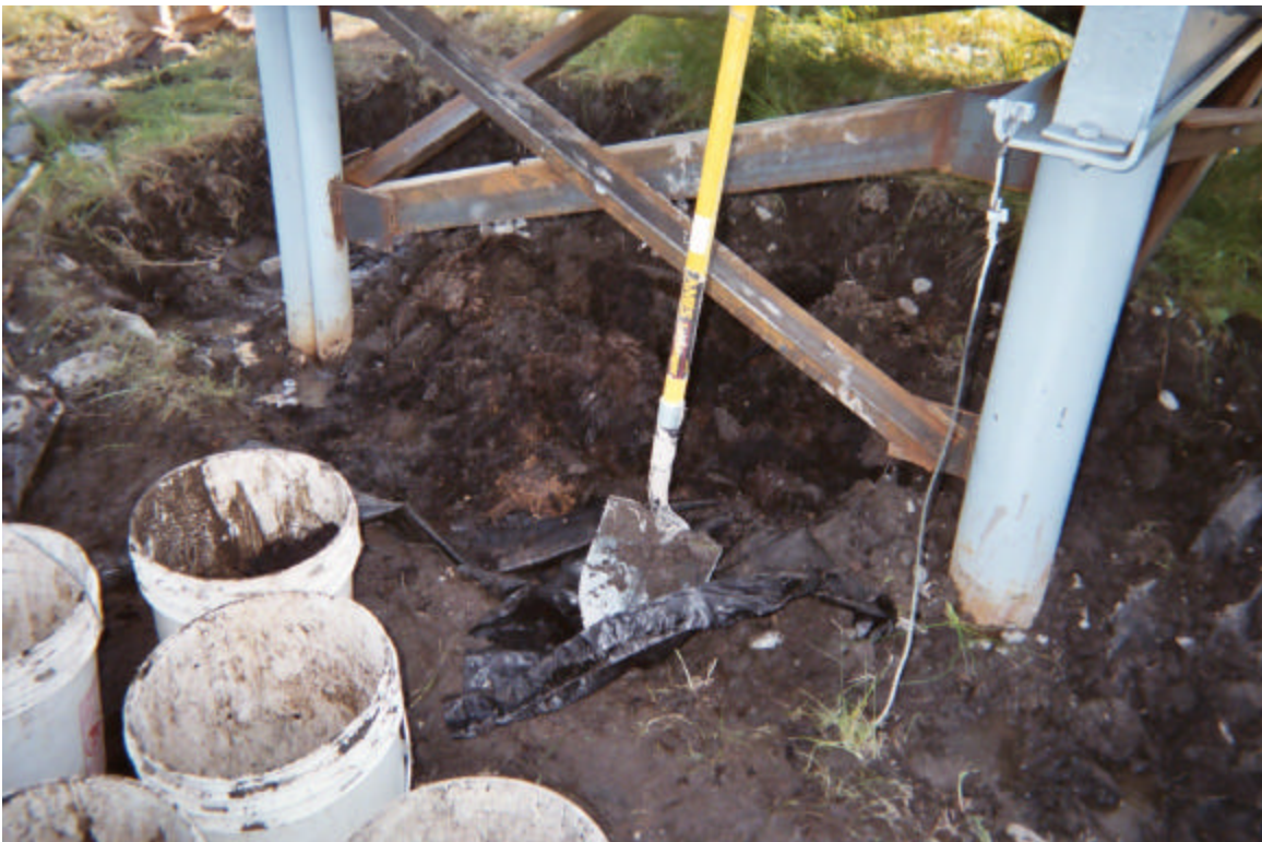
Excavation at Tank 2 center, note contaminated organic matter.
