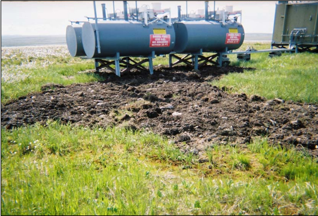
Tundra material fill from 2006 field season with re-vegetation in progress looking south.
