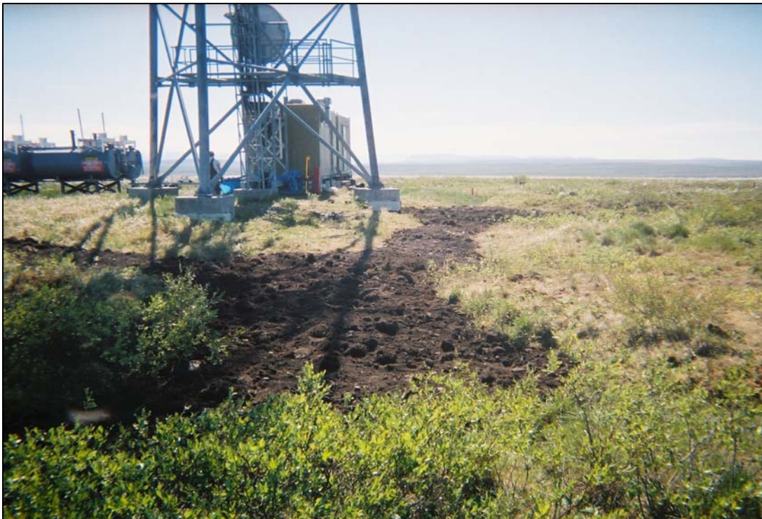
Tundra material backfill complete in the depression looking south.
