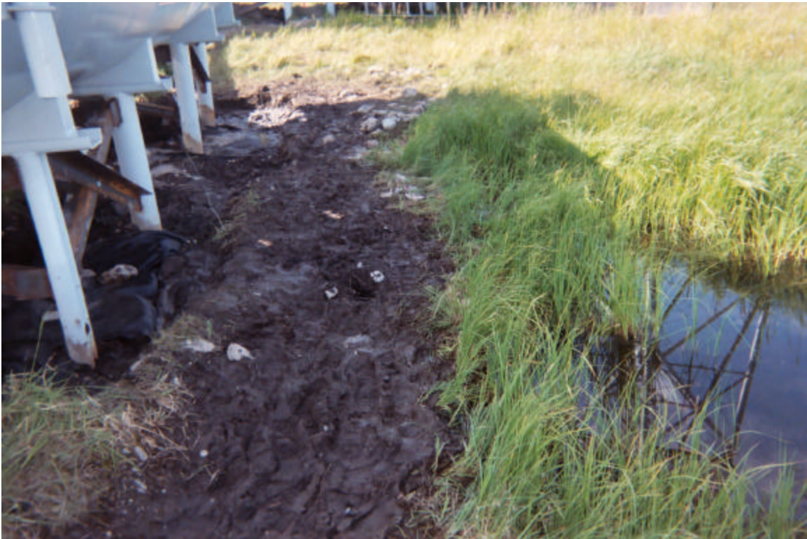
View between tank and water; looking west.
