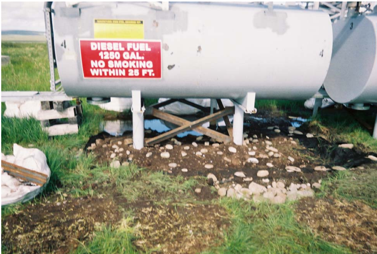
Initial layer of native fill material applied at AST 4. Looking north.
