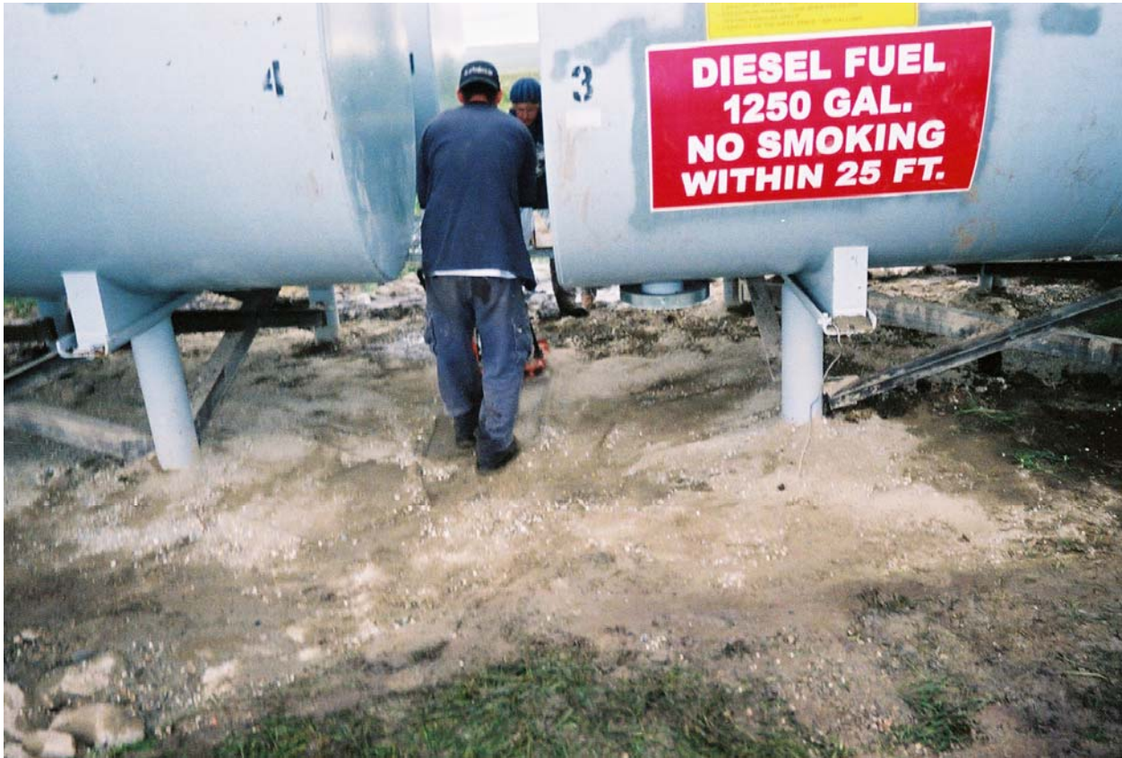
Compacting fill between AST's 3 and 4. Looking north.
