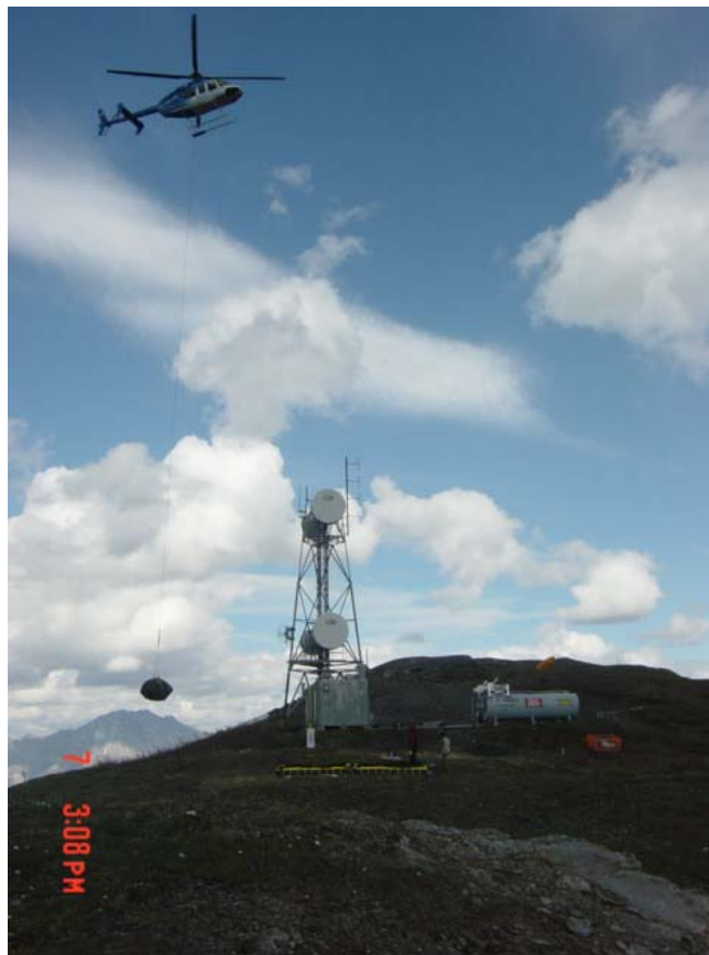
Fuel bladder sling load to portable secondary containment system on ground at repeater site.
