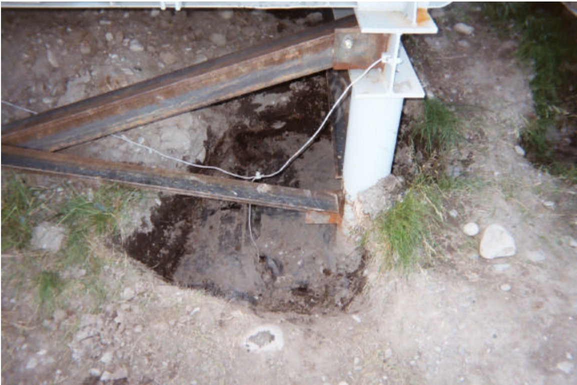
Final excavation at generator module.
