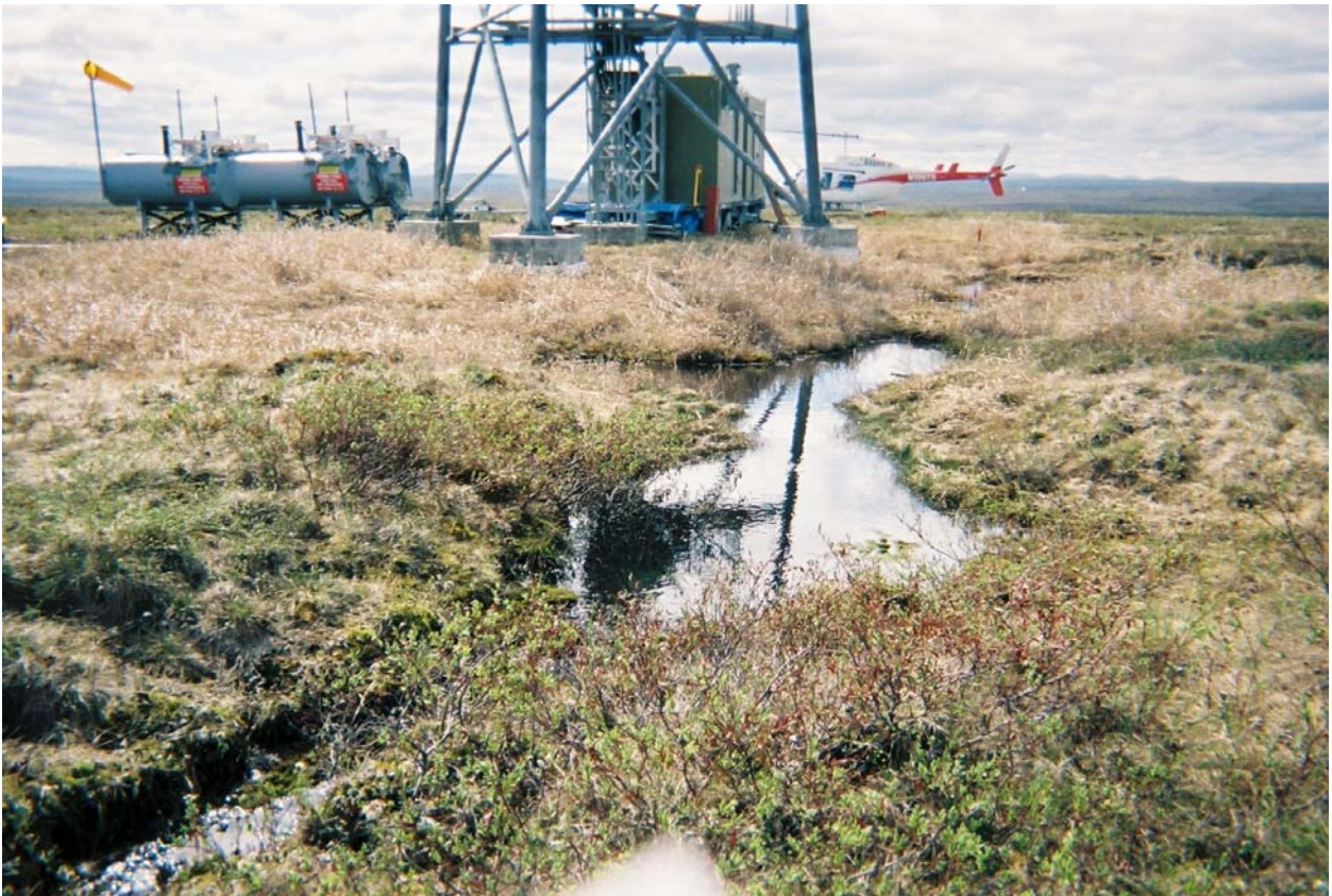
Surface Water pond north of the Communication Tower looking south.
