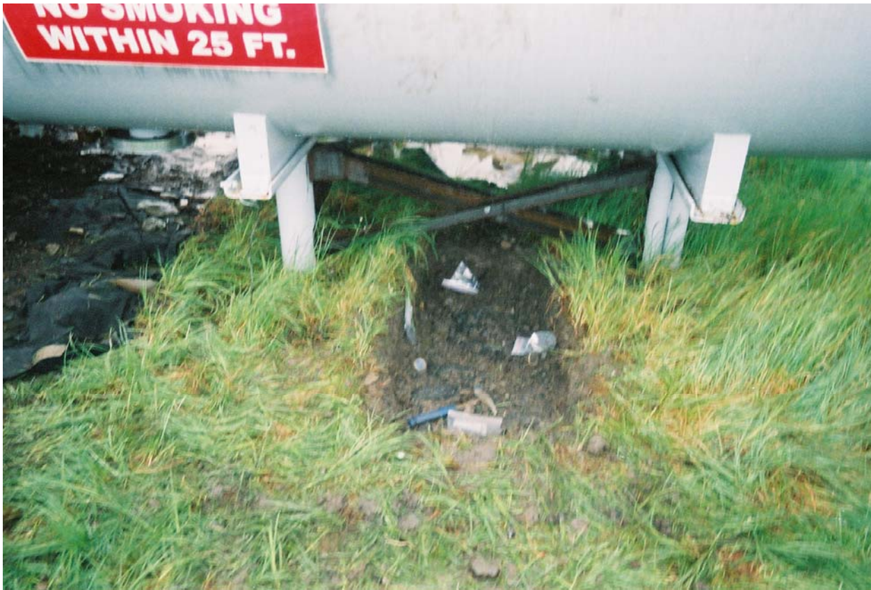
Early stages of excavation beneath AST 3. Looking north.
