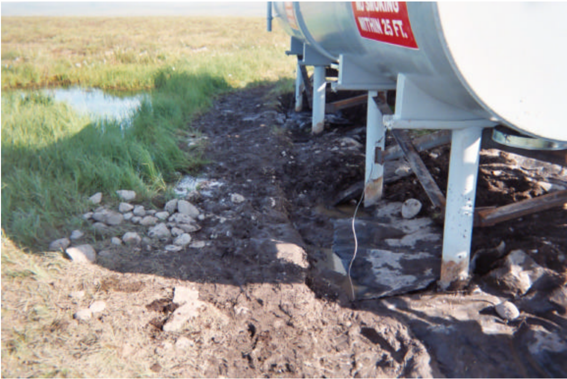
Excavation at Tank 1 and Tank 2; note distance to adjacent surface water.
