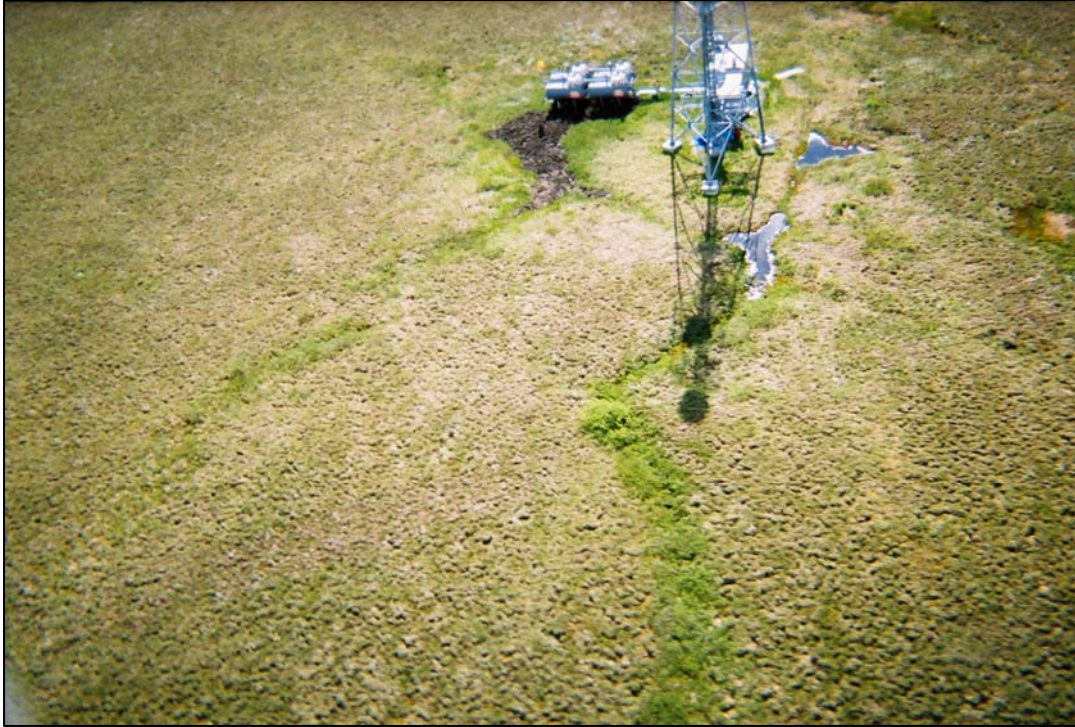
Costa Hill Repeater prior to dewatering activities looking south.
