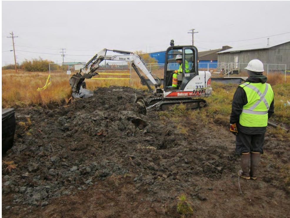
**PHOTOGRAPH 13: PLACING DRUMS BACK INTO TRENCHES AND RETURNING SOIL TO ITS APPROXIMATE ORIGINAL LOCATION; LOOKING SOUTHEAST. 10/05/2013.**
