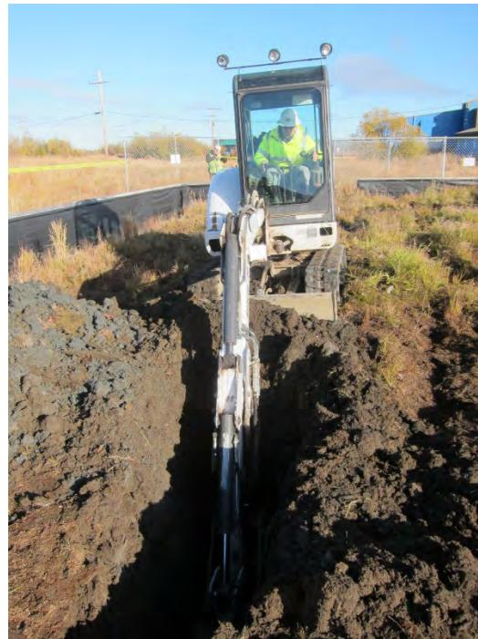
**PHOTOGRAPH 2: EXCAVATING TO PROPOSED DEPTH OF 8' BELOW GROUND SURFACE AT WEST END OF PROPOSED EAST/WEST TRENDING TRENCH; LOOKING EAST 10/04/2103.**
