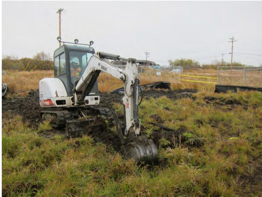
**PHOTOGRAPH 11: DIGGING TEST PITS TO BETTER DELINEATE PERIMETER OF BURIED DRUM CLUSTER; LOOKING SOUTHEAST. 10/05/2013.**
