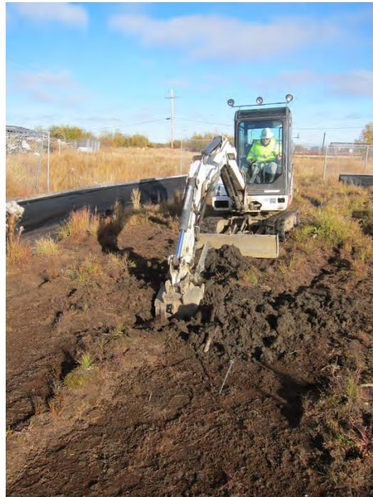
**PHOTOGRAPH 1: BEGINNING TO EXCAVATE AT WEST END OF PROPOSED EAST/WEST TRENDING TRENCH IN AREA OF SUSPECTED BURIED DRUMS; LOOKING EAST. 10/04/2013.**
