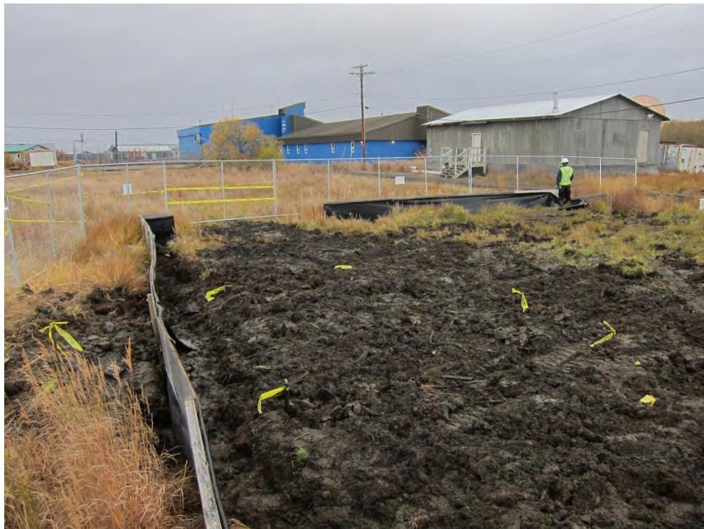
**PHOTOGRAPH 14: PLACE FLAGGING ALONG PERIMETER OF BURIED DRUM CLUSTER FOR VISUAL REFERENCE; LOOKING SOUTHEAST. 10/05/2013.**
