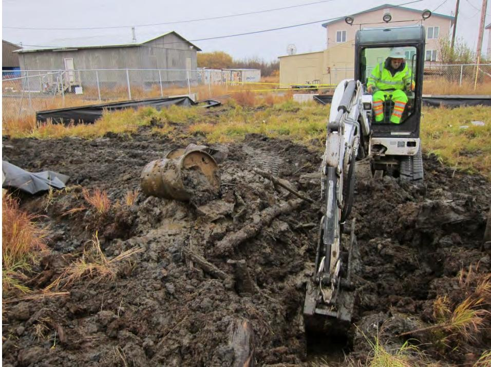
**PHOTOGRAPH 5: EXCAVATING TRENCH FROM NORTH TO SOUTH THROUGH ASSUMED CENTER OF BURIED DRUM CLUSTER. DRUMS ENCOUNTERED AND REMOVED FOR VISUAL INSPECTION; LOOKING SOUTH. 10/05/2013.**
