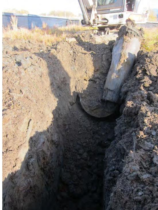
**PHOTOGRAPH 4: ENCOUNTERING BURIED DRUMS AND WOODEN PILINGS APPROXIMATELY 1.5 TO 2' BELOW GROUND SURFACE AND 8' EAST OF WESTERN STARTING POINT OF TRENCH EXCAVATION; LOOKING EAST. 10/04/2013.**
