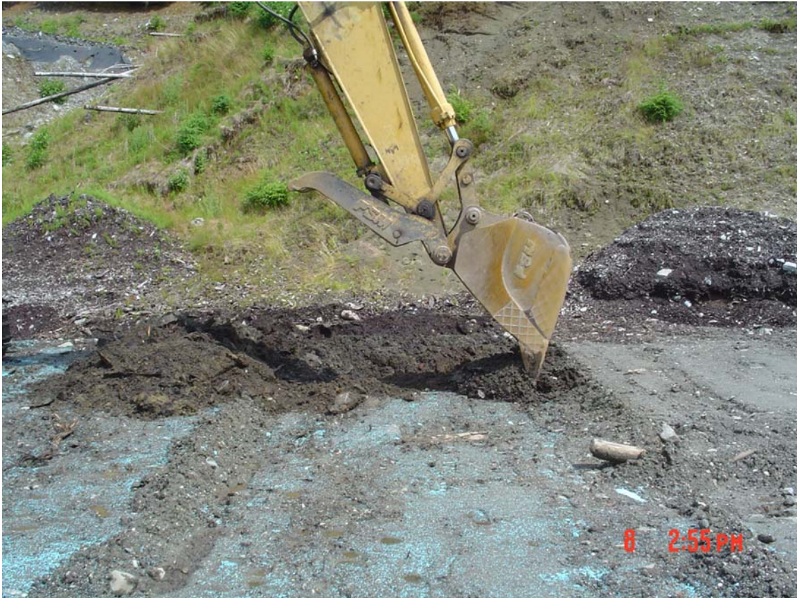
Photo 13. Mixing Soil Using an Excavator Bucket
