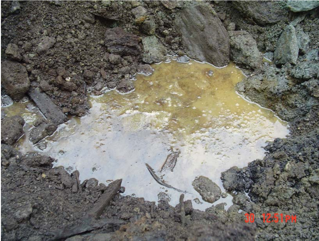
Photo 9. View of Oil on Water Table After First Round of Excavation
