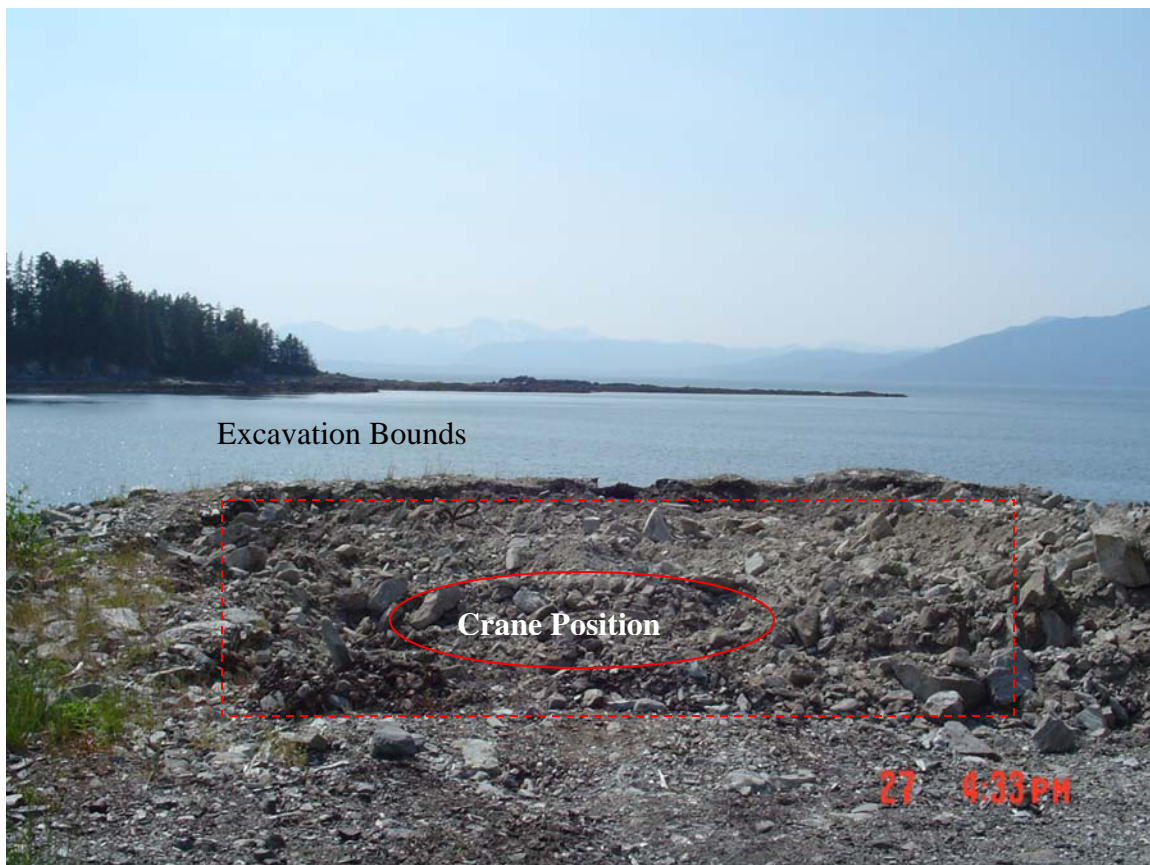
Photo 6. LTF Crane Pad Excavation
