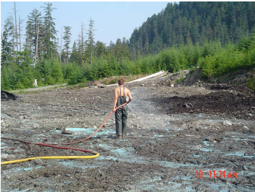
Photo 12. Spraying Microbes Across a Typical Grid.
