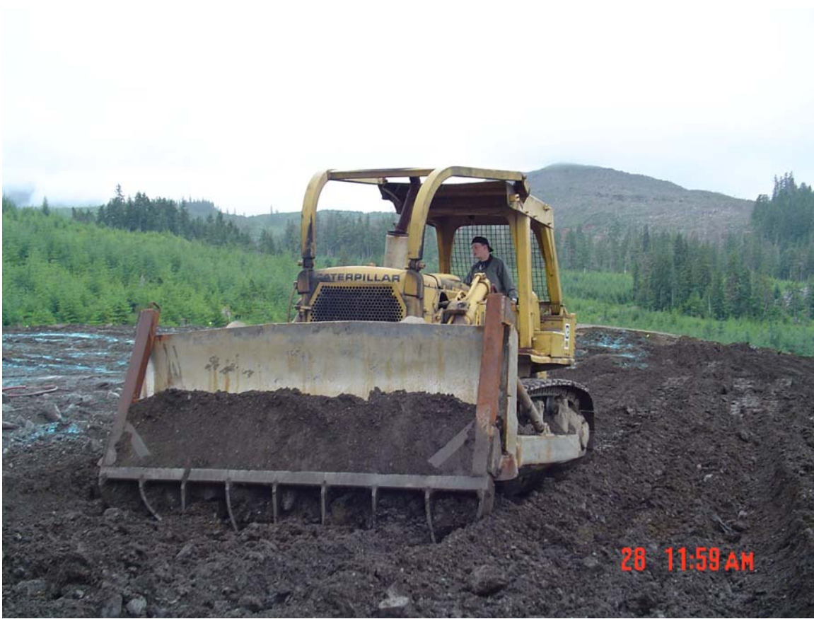
Photo 14. Mixing Soil Using a Dozer Rake.
