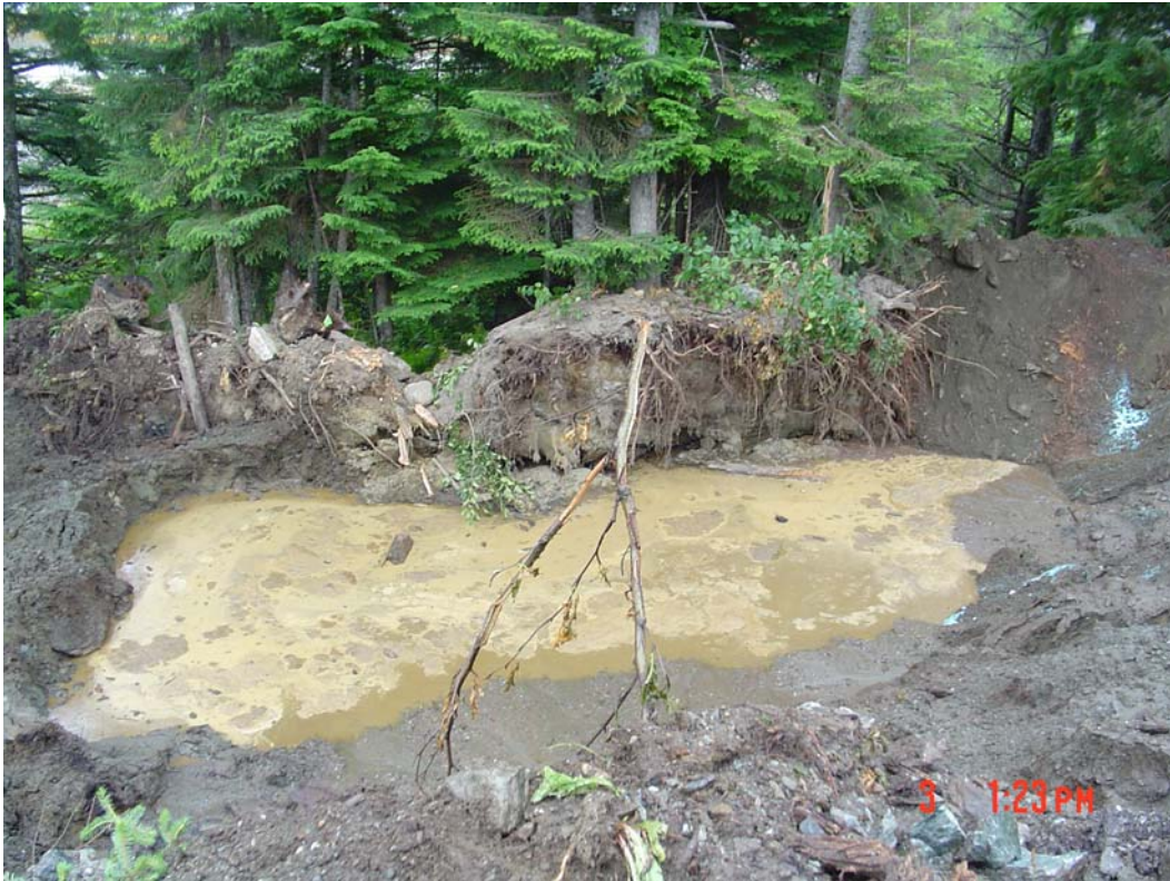
Photo 15. Microbes and Nutrient Added to Lower Fuel Depot.
