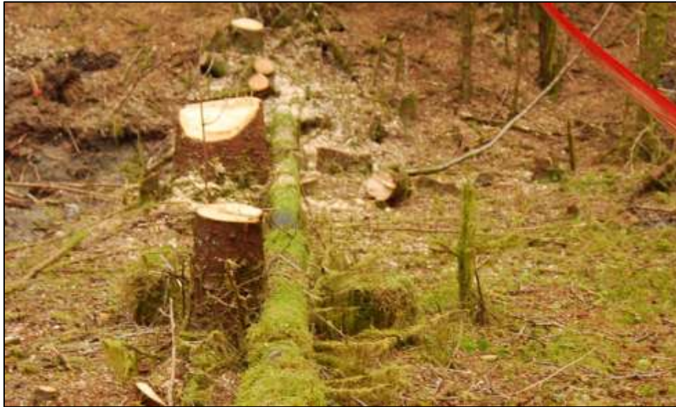
Photograph 3. Site clearing in preparation for abatement.
