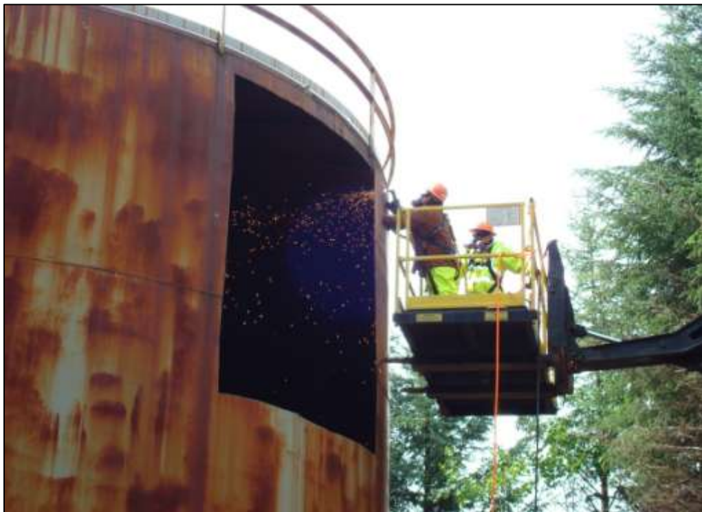
Photograph 10. Dismantling the 130,000-gallon AST.
