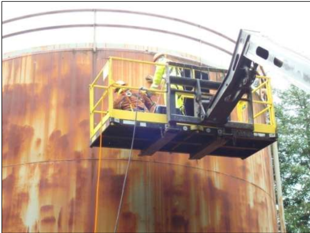
Photograph 9. Starting the task of dismantling the 130,000-gallon AST.
