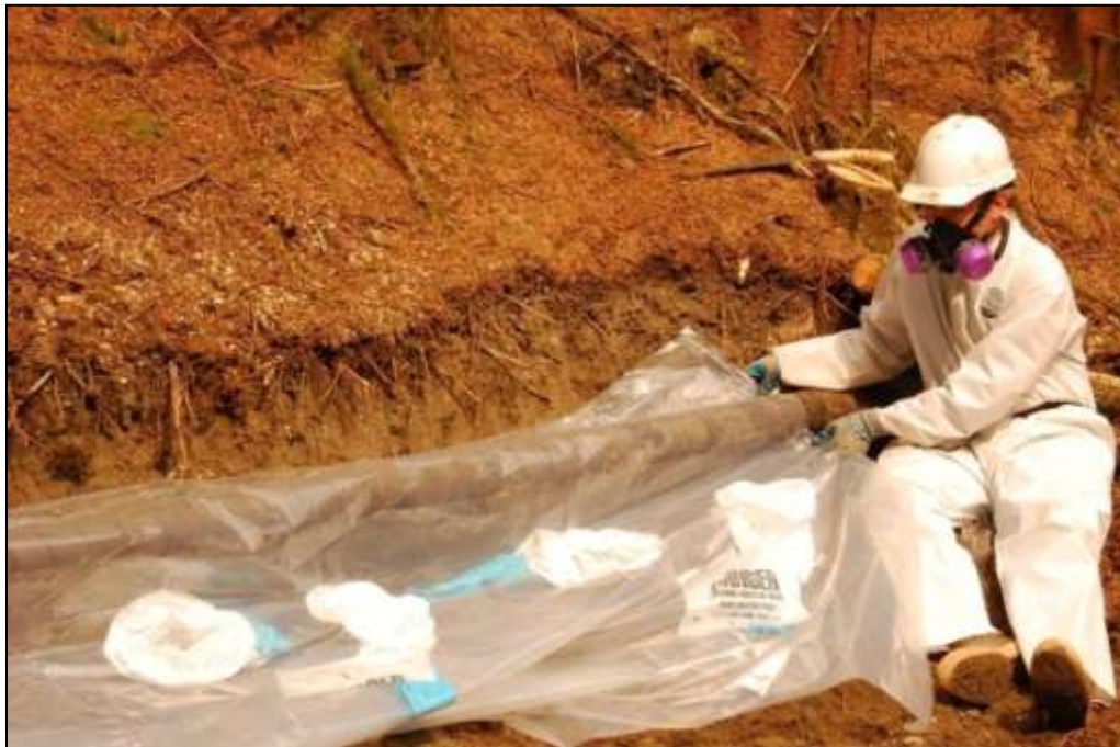
Photograph 5. Wrapping the pipe with the glovebag.
