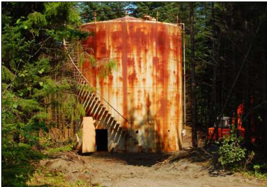
Photograph 2. 130,000-Gallon Fuel Tank with Access Door
