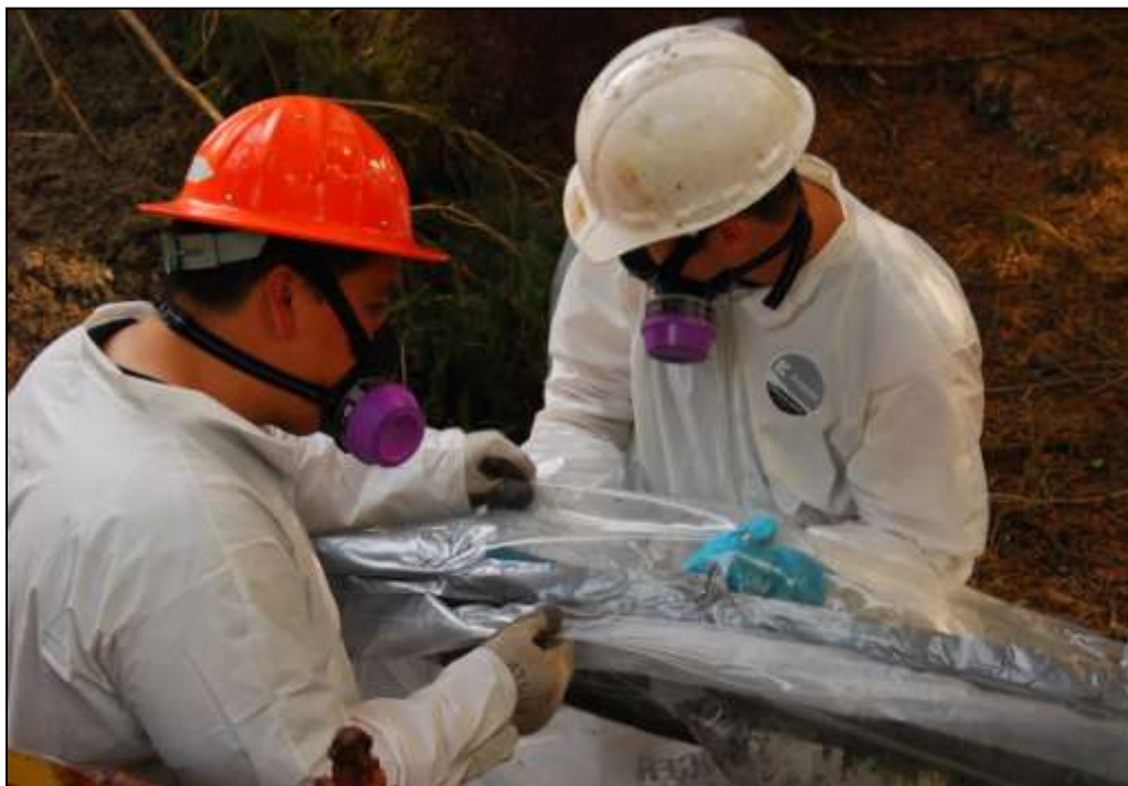
Photograph 6. Sealing the top of the glovebag.
