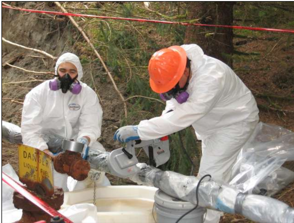
Photograph 7. Cutting pipe into sections with plastic containment below the pipe.
