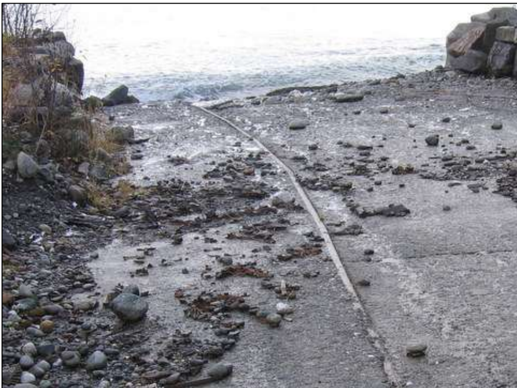
Photograph 14. Rails remaining at the Seaplane Ramp.
