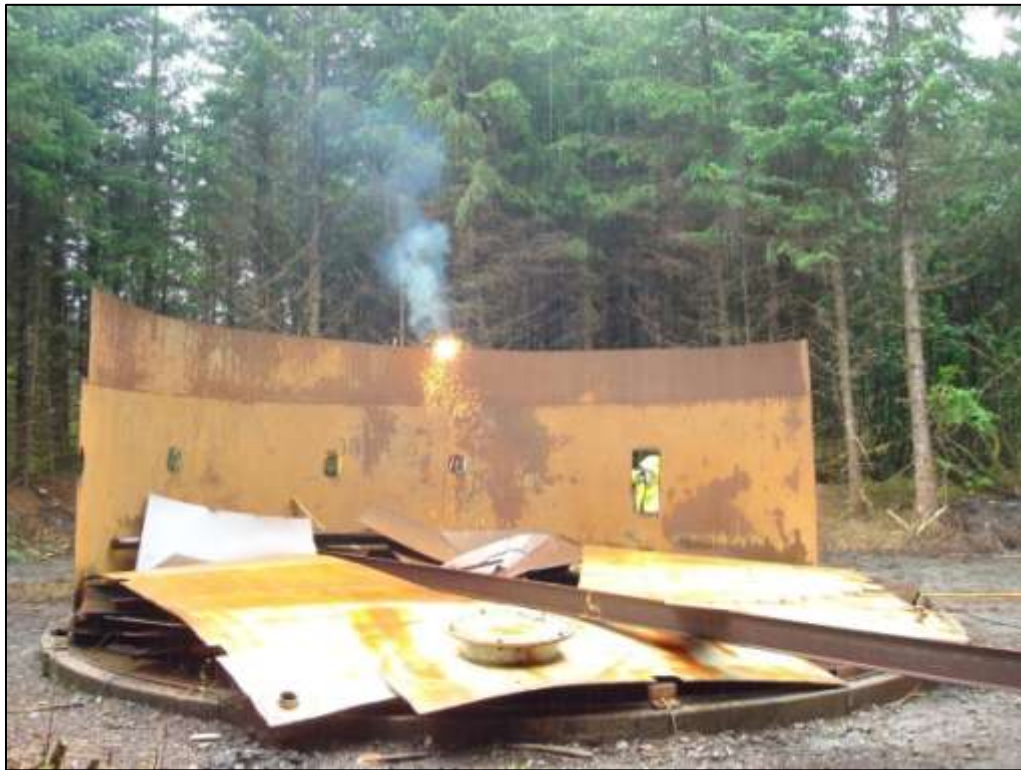
Photograph 11. Dismantling the lower section of the AST.
