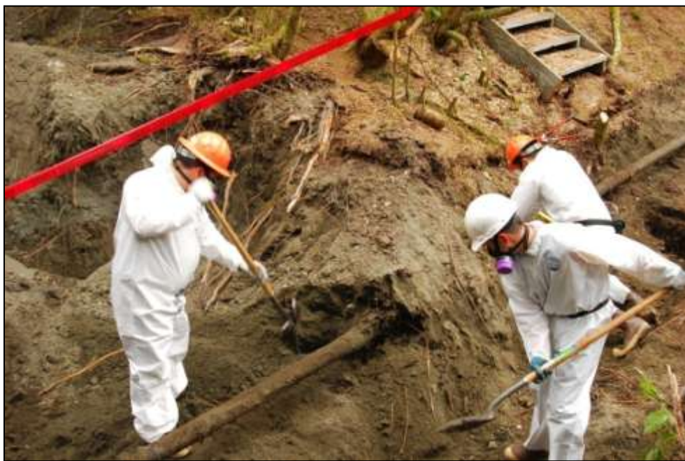
Photograph 4. Uncovering the pipe from beneath the berm using hand tools.
