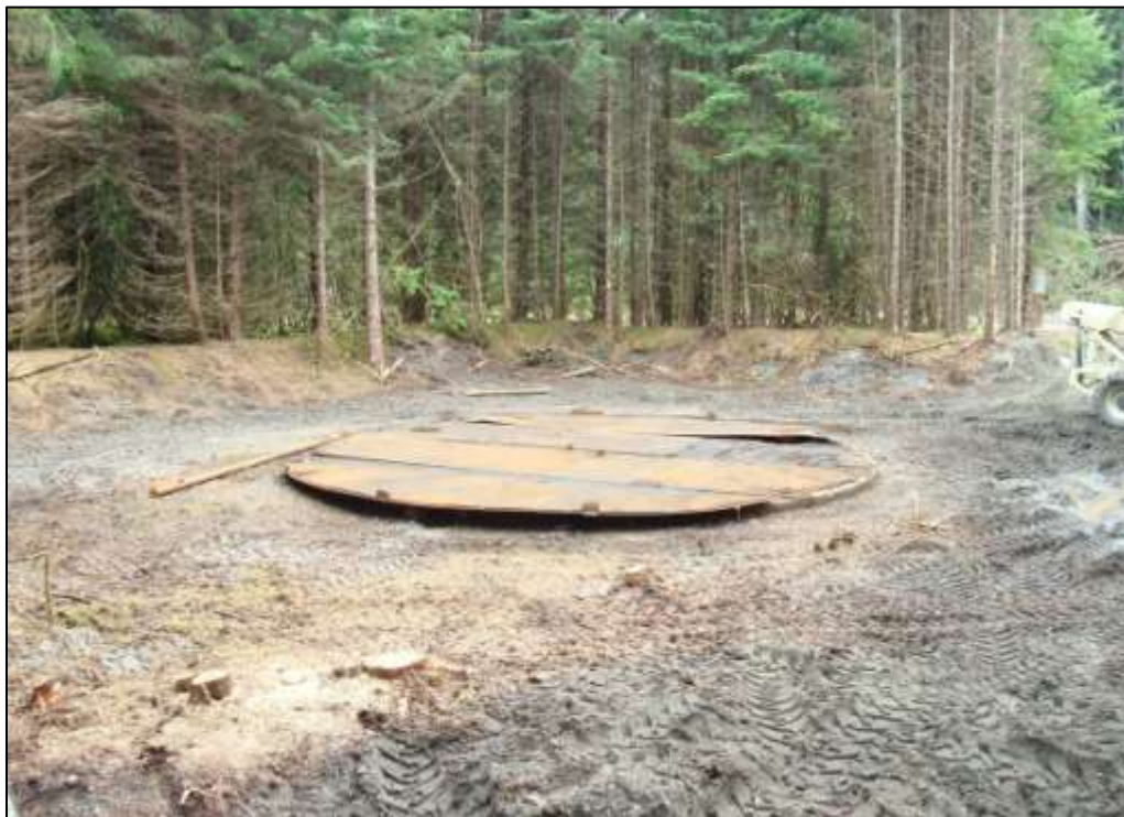
Photograph 12. Site after completion of AST removal.
