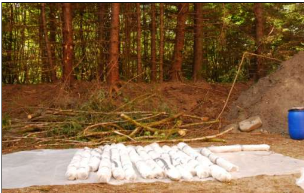
Photograph 8. Fourteen (14) sections of wrapped pipes ready for disposal.
